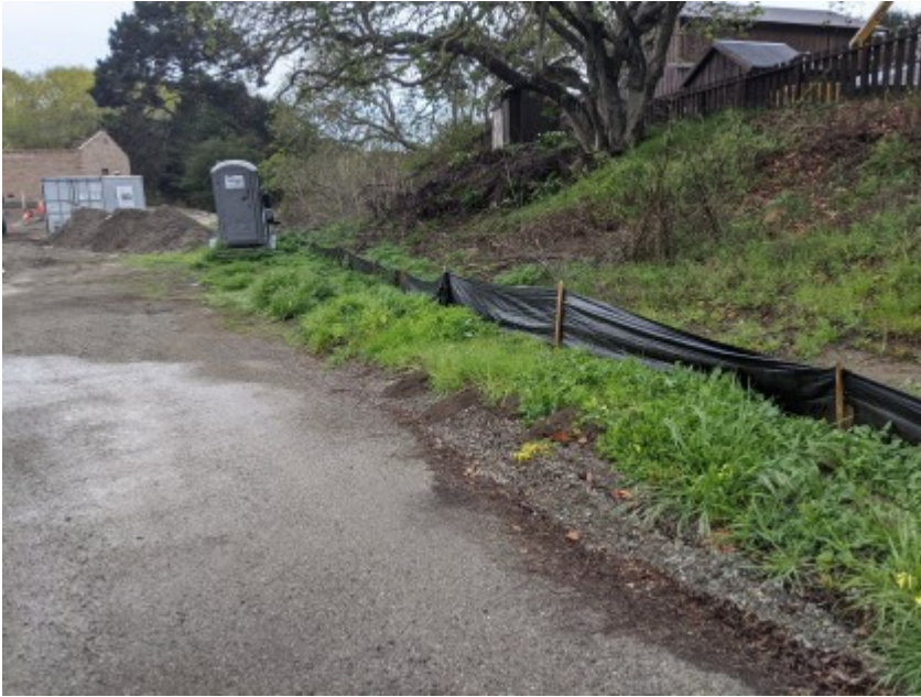
03/09/2021 - Intact exclusionary fencing surrounding work area.
