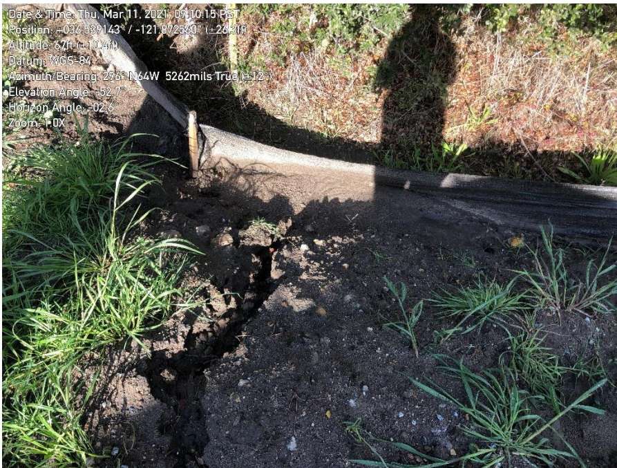
Photo 5. Sediment starting to back up against silt fence due to recent rain event.
