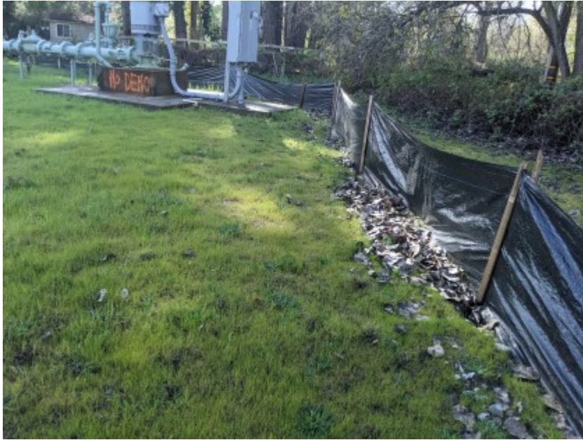
03/11/2021 - Intact exclusionary fencing surrounding work area.
