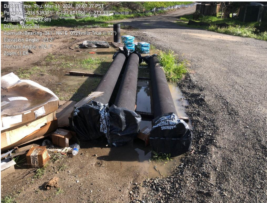
Photo 3. Pipes capped.
