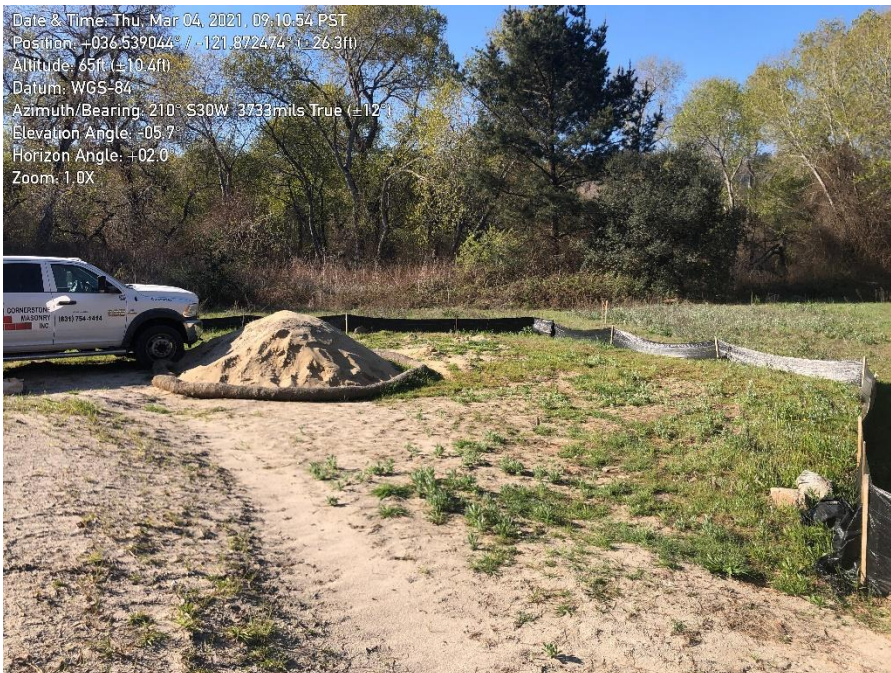
Photo 4. BMPs in place.
