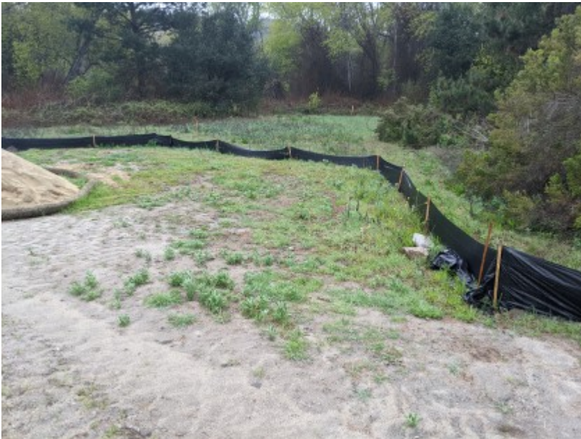
03/09/2021 - Intact exclusionary fencing surrounding work area.
