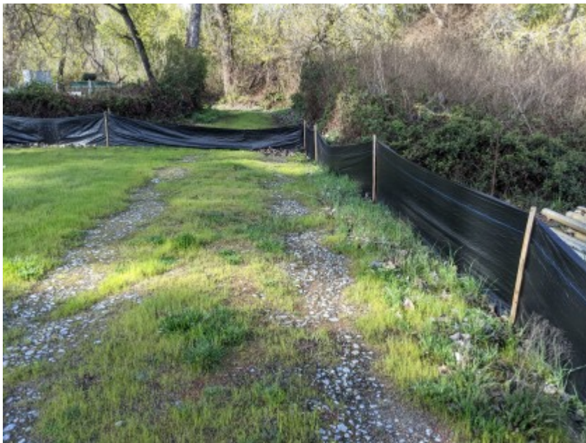
03/11/2021 - Intact exclusionary fencing surrounding work area.
