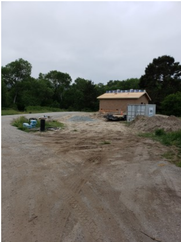
04/22/2021 - Typical site conditions.
