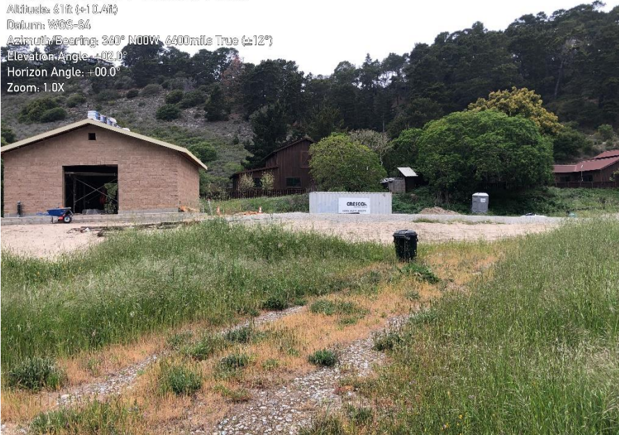
Photo 1. Pump station and overall site conditions.
