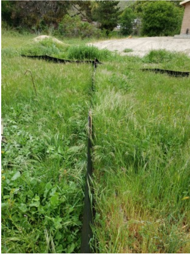
04/22/2021 - Recommend vegetation removal on exclusion fence.
