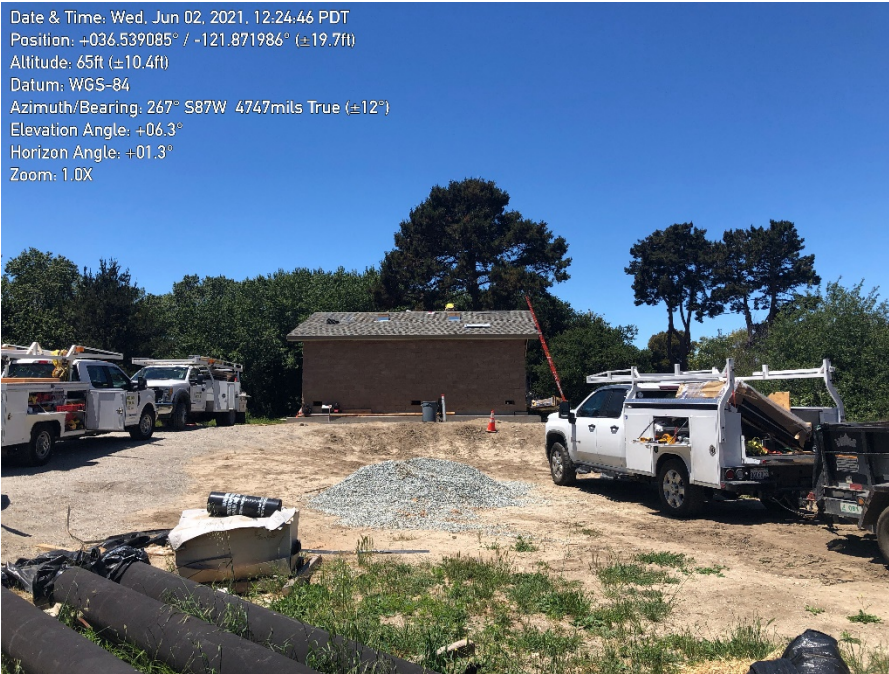
Photo 1. General site conditions.
