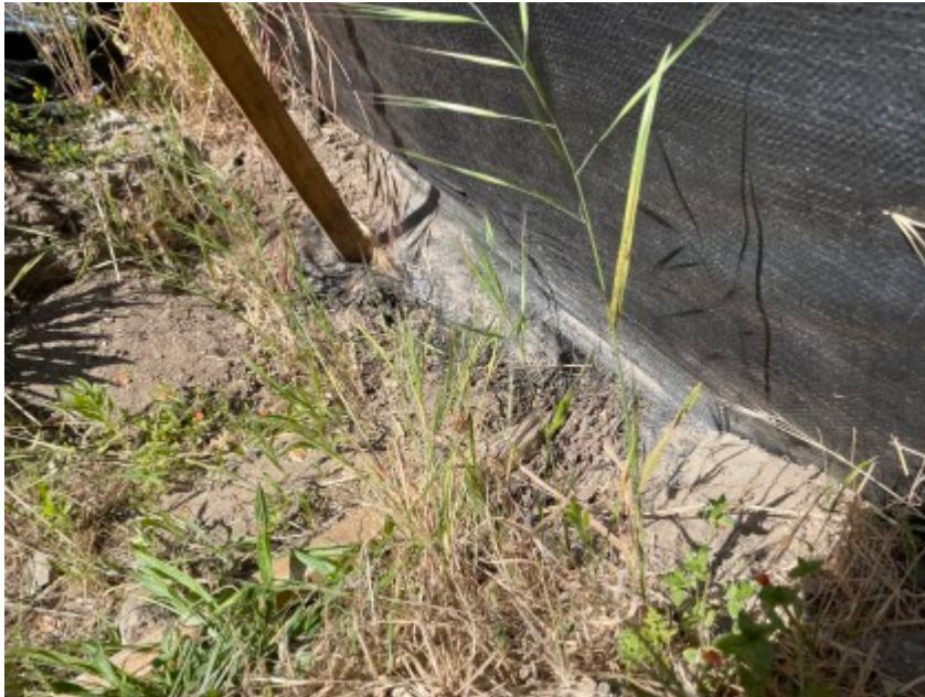
06/10/2021 - Hole located at the bottom of exclusion fencing.
