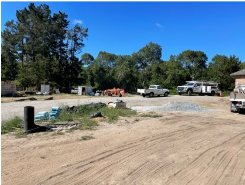
06/10/2021 - Typical site conditions.
