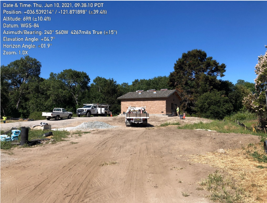
Photo 1. General site conditions.
