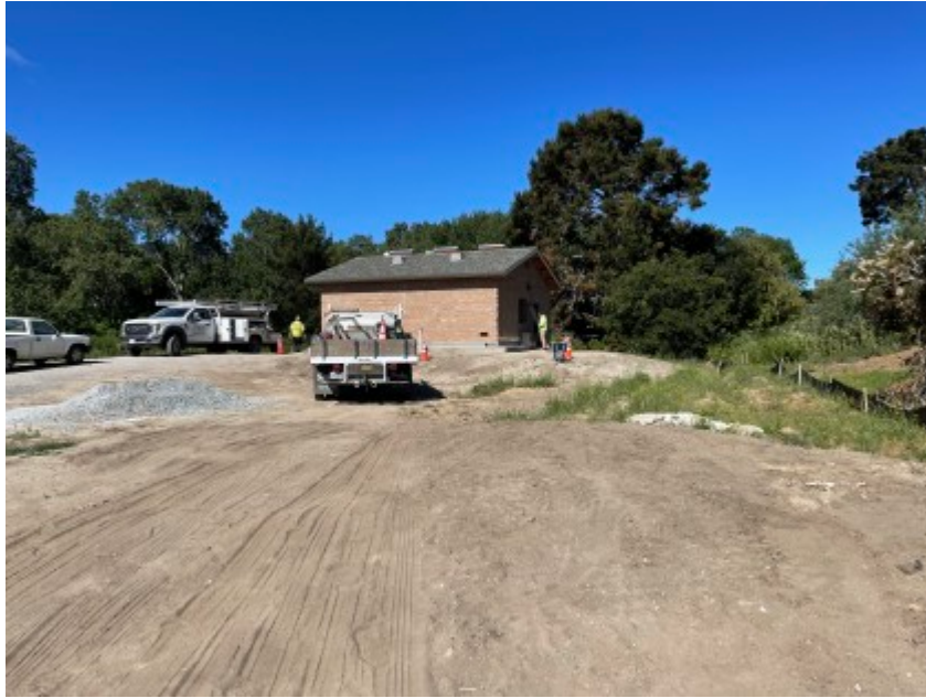
06/10/2021 - Typical site conditions.
