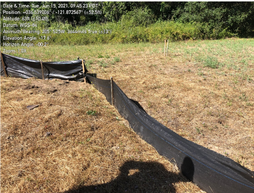
Photo 2. Exclusion fencing in acceptable condition.
