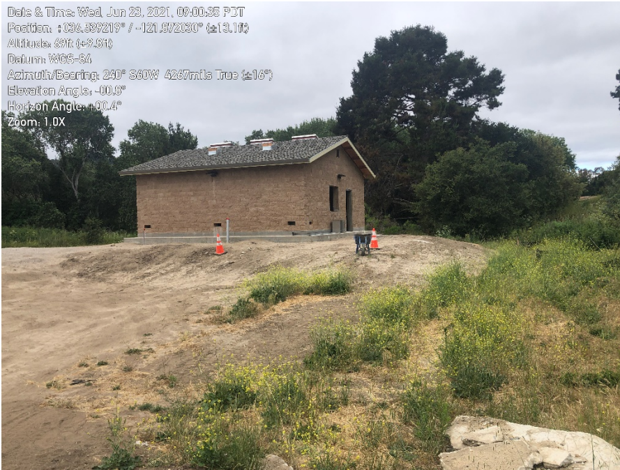
Photo 3. General site conditions.
