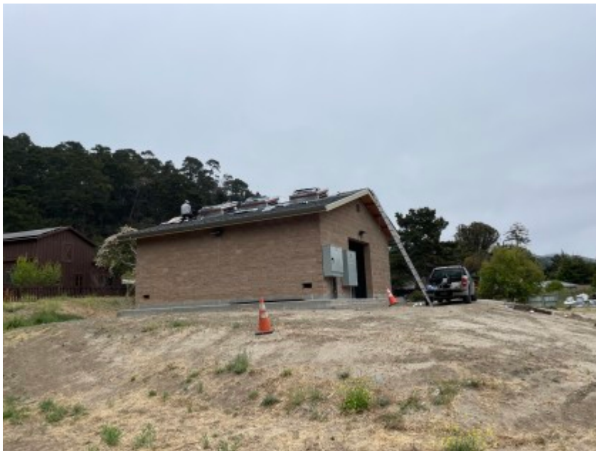
06/21/2021 - Construction activities observed (roofing)
