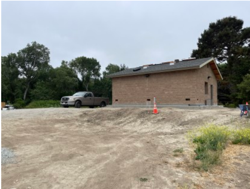
06/21/2021 - Project site overview
