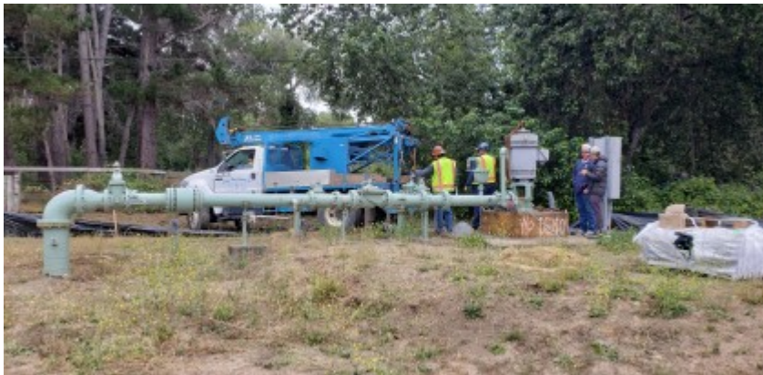
07/13/2021 - Well demolition activities.
