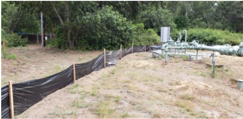
07/15/2021 - Reinstalled exclusion fencing.
