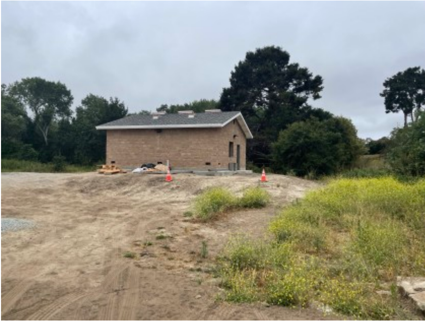
07/14/2021 - Project site conditions.
