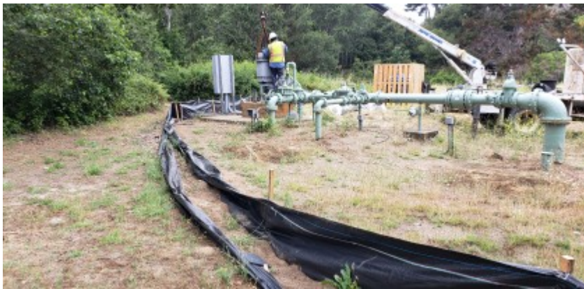
07/13/2021 - Well demolition activities.
