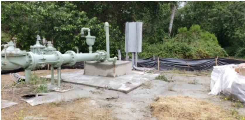
07/15/2021 - Well demo complete. Excess grout to be removed by project contractor.
