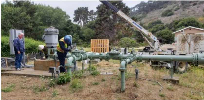
07/13/2021 - Well demolition activities.
