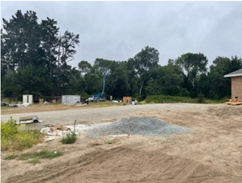
07/14/2021 - Project site conditions.
