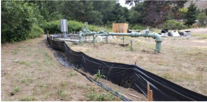
07/15/2021 - Reinstalled exclusion fence.
