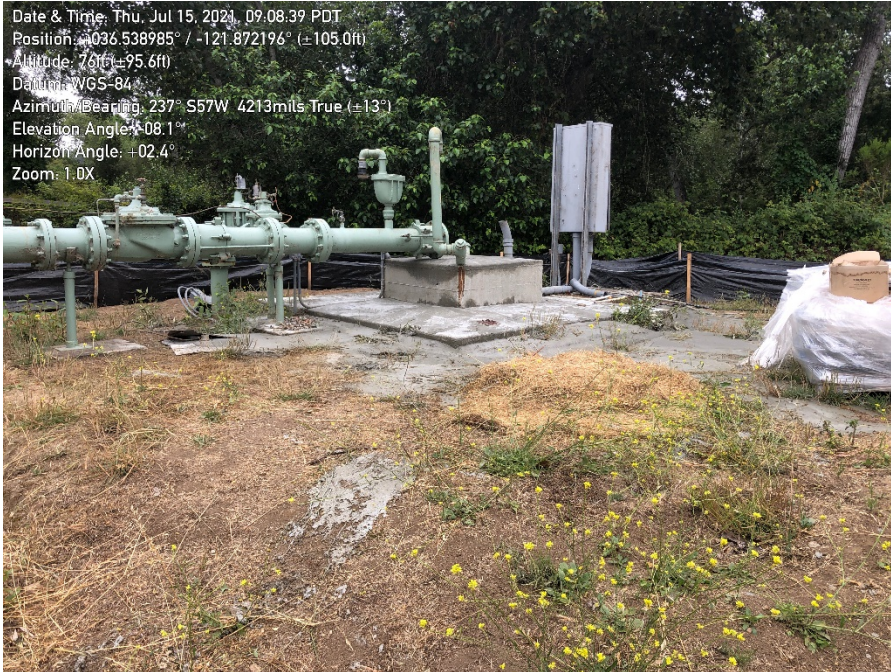
Photo 1. Well demolition (sealing of well).
