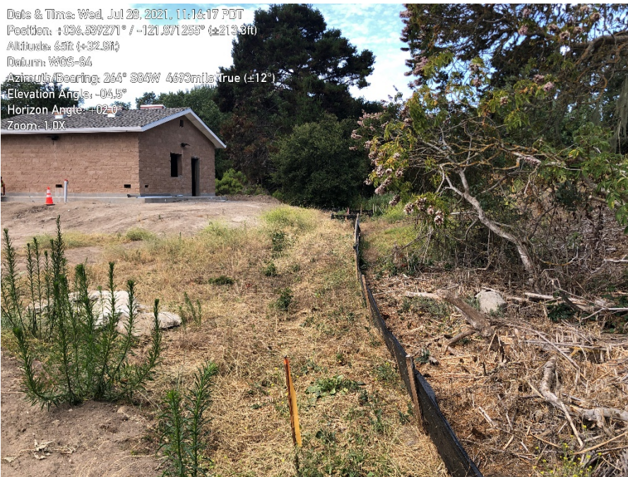
Photo 2. Mustard along silt fence has been mowed.
