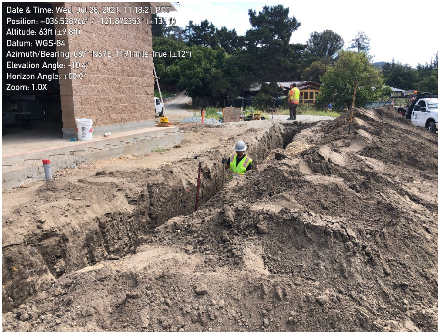
Photo 3. Trenching and pipe installation along south side of pump station.
