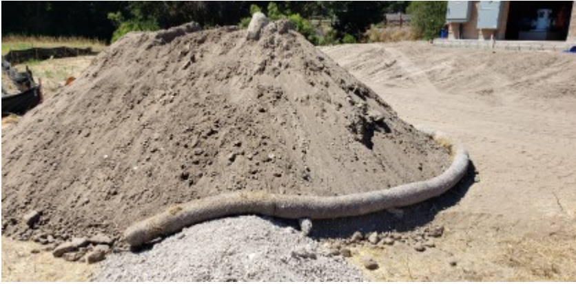
08/04/2021 - Spoils pile with plastic monofilament wattle.
