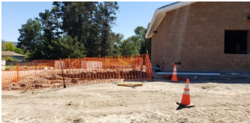
08/04/2021 - Fencing surrounding excavation.
