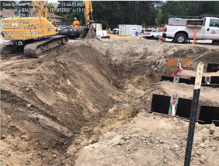
Photo 2. Trenches ramped to prevent wildlife entrapment.
