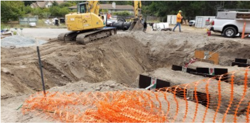
08/17/2021 - Suction manifold installation pit.
