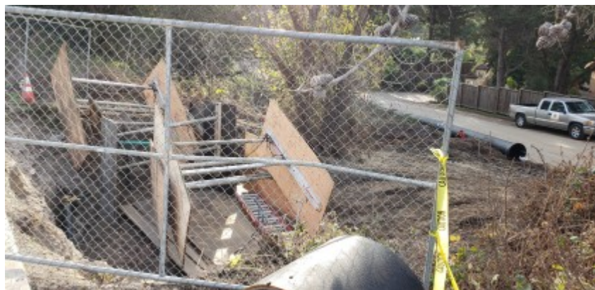
11/18/2021 - Trench shoring materials staged in tie in location.
