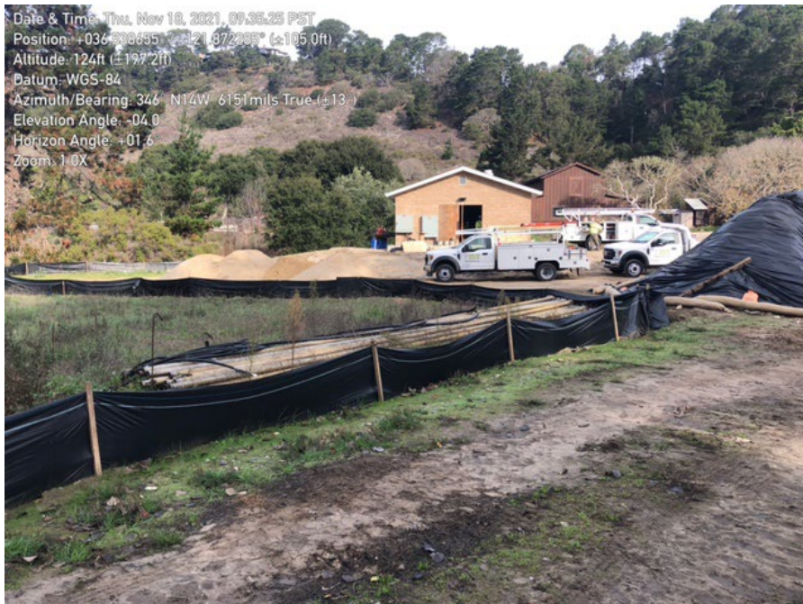
Photo 4. Silt fence in good condition.
