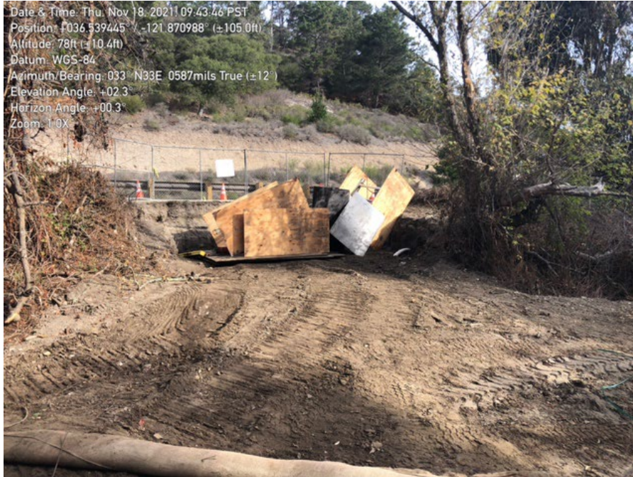
Photo 1. Shoring stored tie-in excavation.
