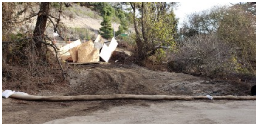
11/18/2021 - Carmel Valley Road tie in location, staged trench shoring materials, erosion control BMPs.
