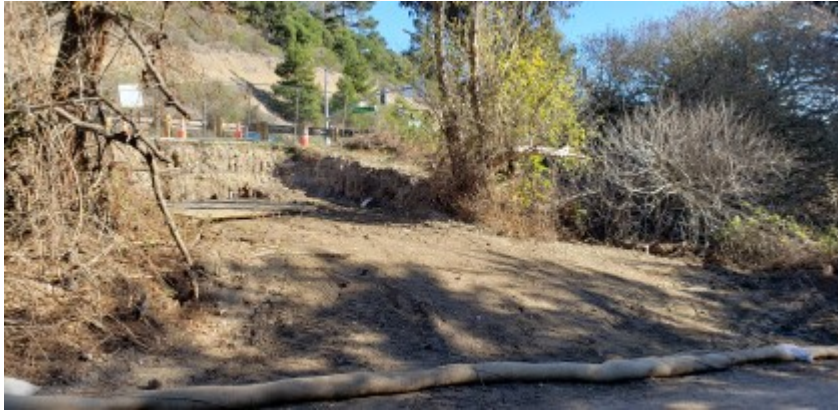
11/24/2021 - Carmel Valley Road tie in location.
