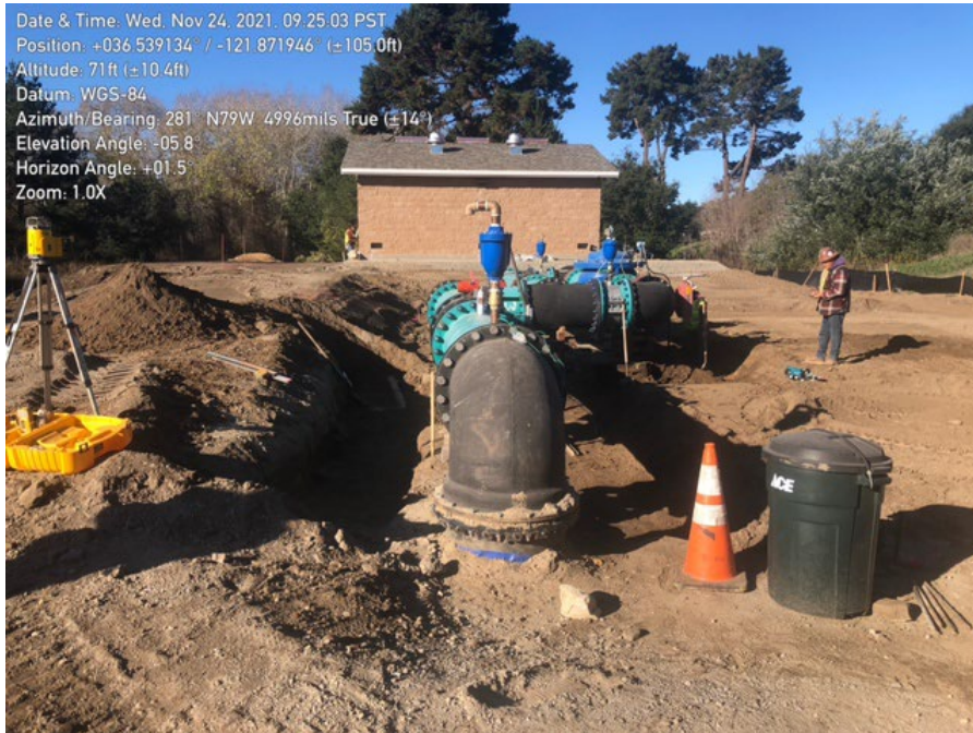
Photo 3. Prep for concrete pour.
