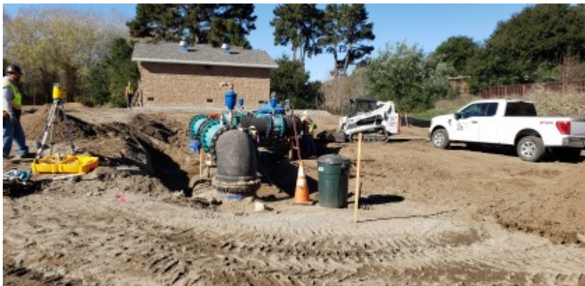
11/24/2021 - Grading activities prior to concrete slab pour.
