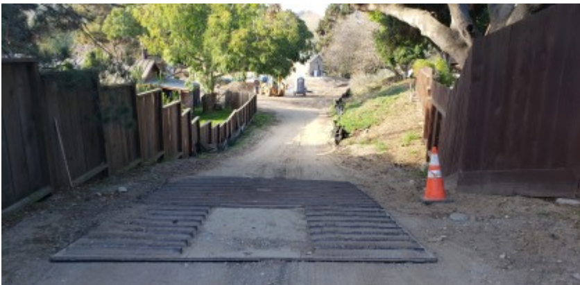
12/02/2021 - CVPS site access.
