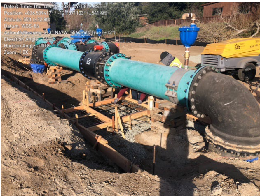
Photo 4. Installation of forms and prep for concrete.
