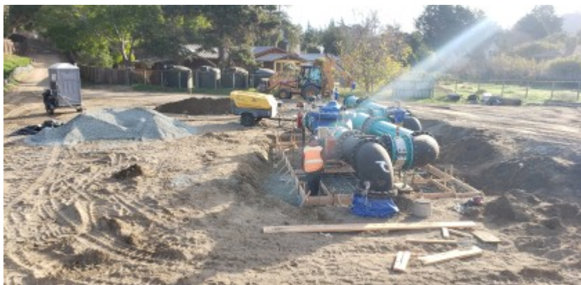
12/02/2021 - Constructing forms for concrete pour.
