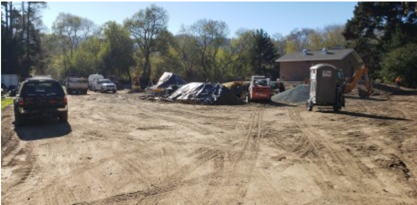
11/29/2021 - Site conditions. Advised CM to apply water for dust control.
