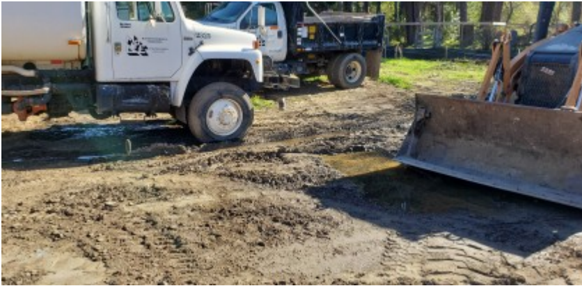
11/29/2021 - Water truck still leaking, standing water on-site.
