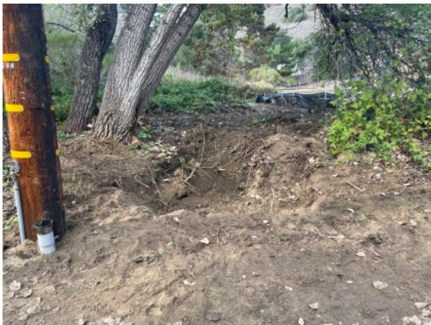
12/09/2021 - MPE completed waterline repair. MPE still needs to add soil to area to meet natural grade.
