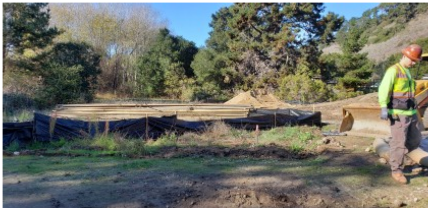
12/07/2021 - Realignment of the exclusion fencing following completion of clearance surveys.
