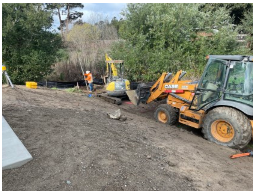
12/09/2021 - MPE beginning the construction of the overflow V ditch along the northern edge of the project.
