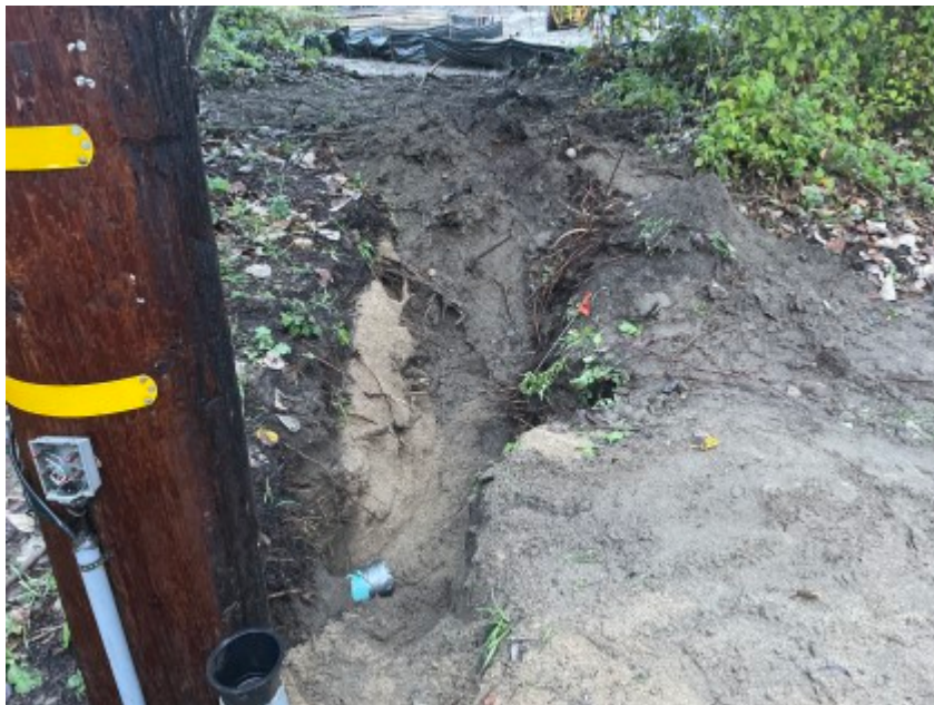
12/09/2021 - Open trench prior to any construction related activities, severed waterline shown in bottom left.
