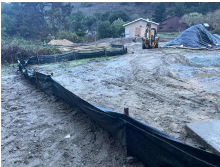
12/09/2021 - CVPS site conditions and re-installed silt/exclusion fencing.
