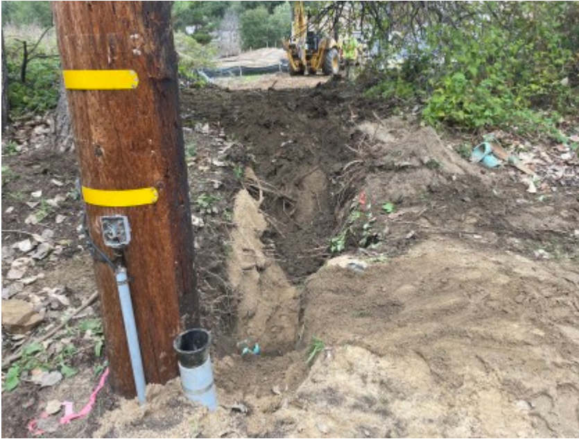
12/08/2021 - Completed electrical installation outside of silt fence, open hole left for MPE to fix broken water pipe. Ramp built for wildlife to exit and not become entrapped.
