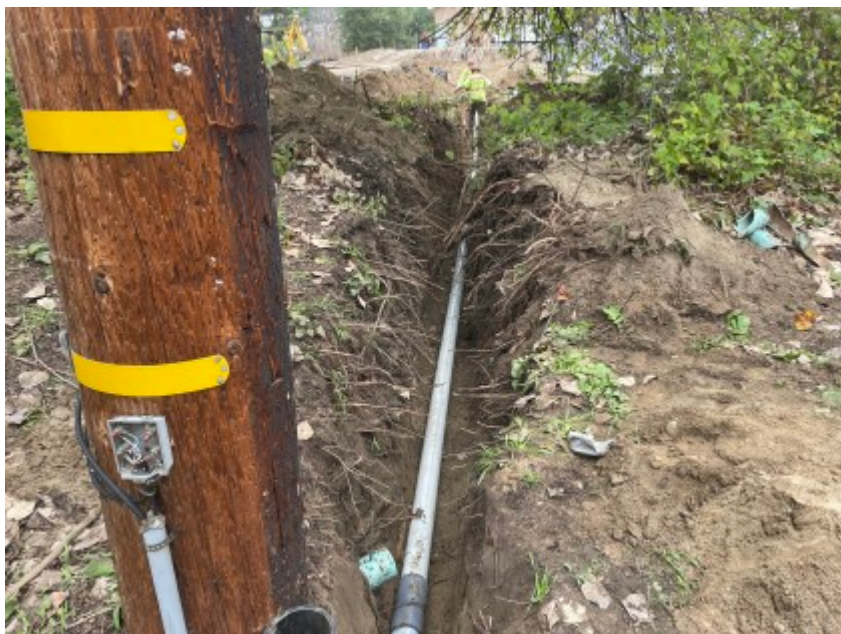
12/08/2021 - Installation of electrical line to CVPS.
