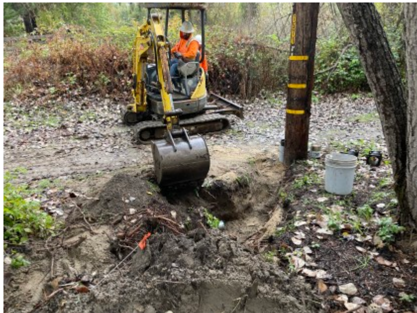
12/09/2021 - MPE fixing broken water line outside of silt fence.
