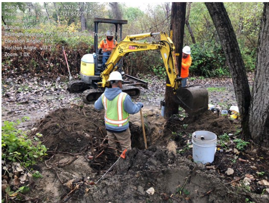
Photo 3. Installation of electrical conduit at PGE pole.
