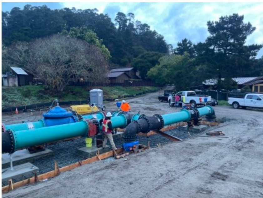
12/09/2021 - CVPS and concrete pad MPE is currently installing.
