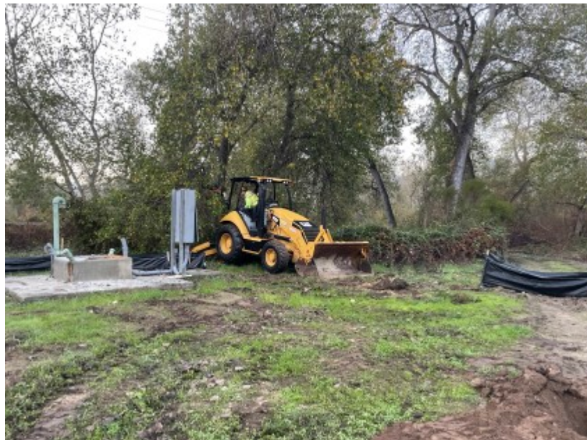
12/08/2021 - Electrical contractor working outside silt fencing along southern edge of the project.
