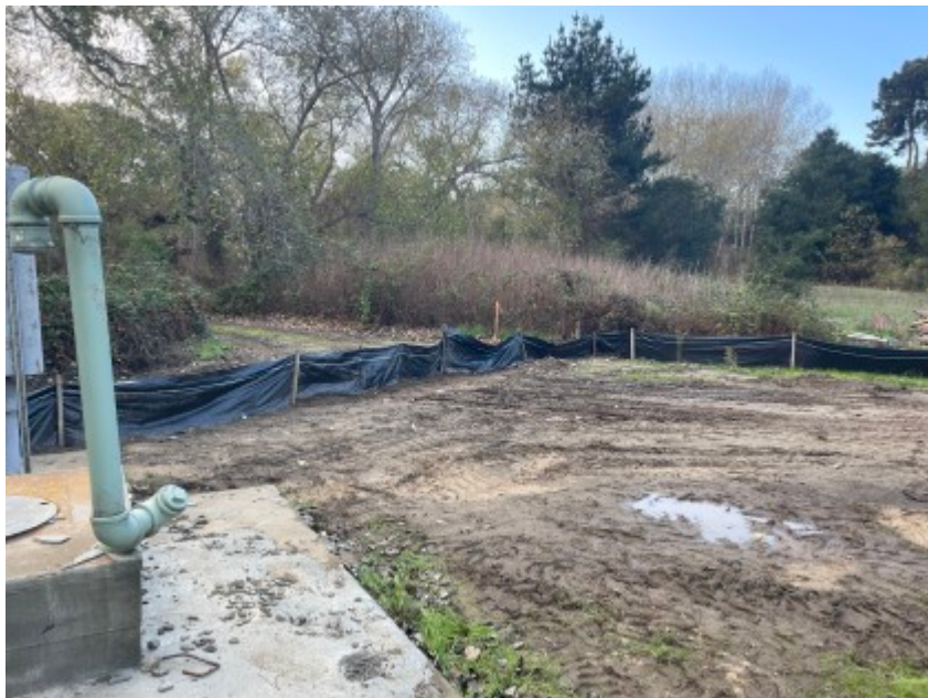
12/09/2021 - MPE re-installed silt fencing on southern edge of project.
