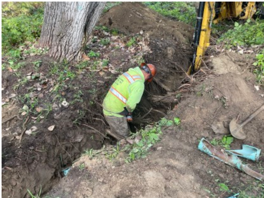
12/08/2021 - Electrical contractor trimming roots with sawzall.
