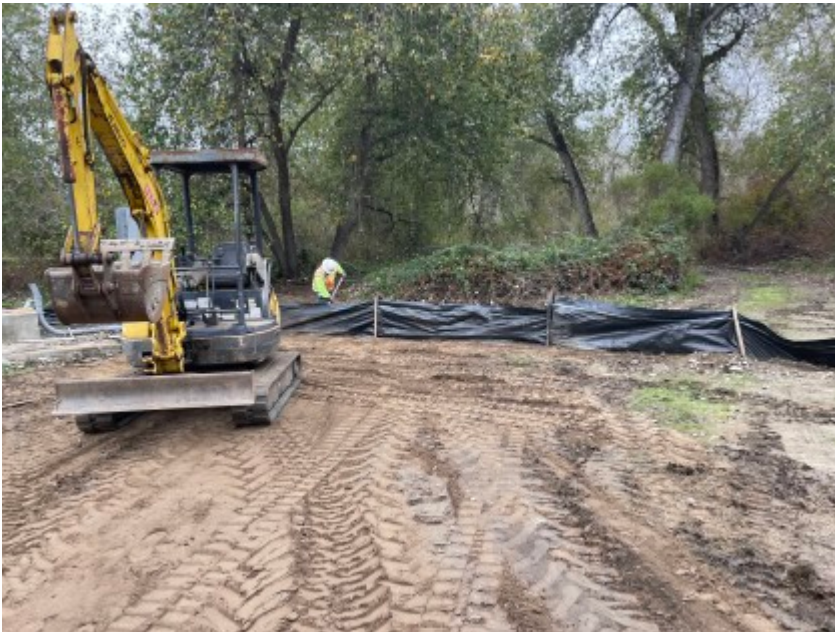
12/08/2021 - MPE re-installing silt fencing where it was taken down to install the electrical line.
