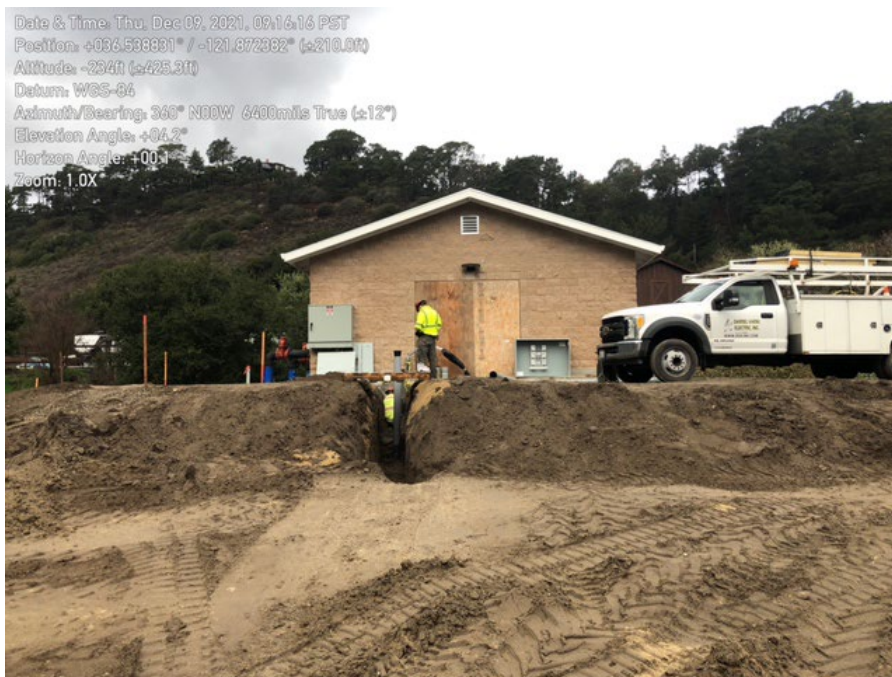
Photo 2. Electrical conduit installation at pump station.
