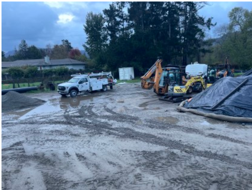
12/09/2021 - CVPS site conditions.
