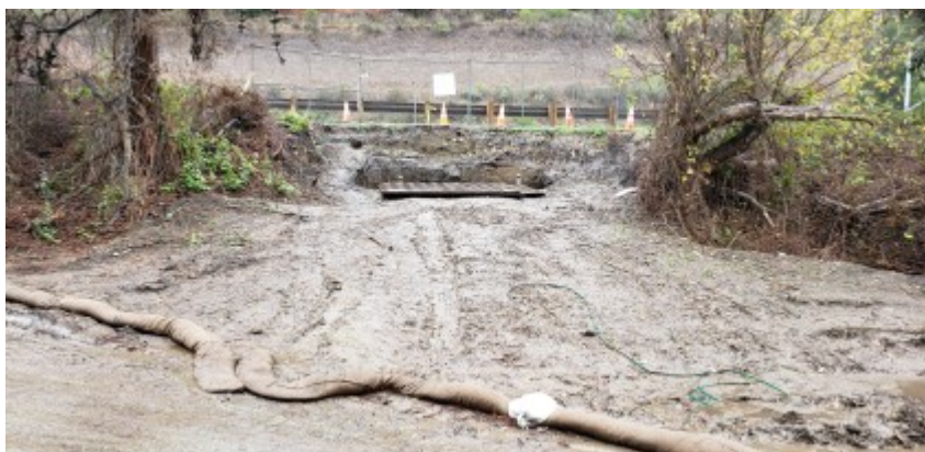
12/23/2021 - Carmel Valley Road tie in location.
