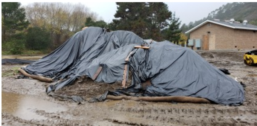
12/23/2021 - Spoils pile erosion control BMP's repaired.
