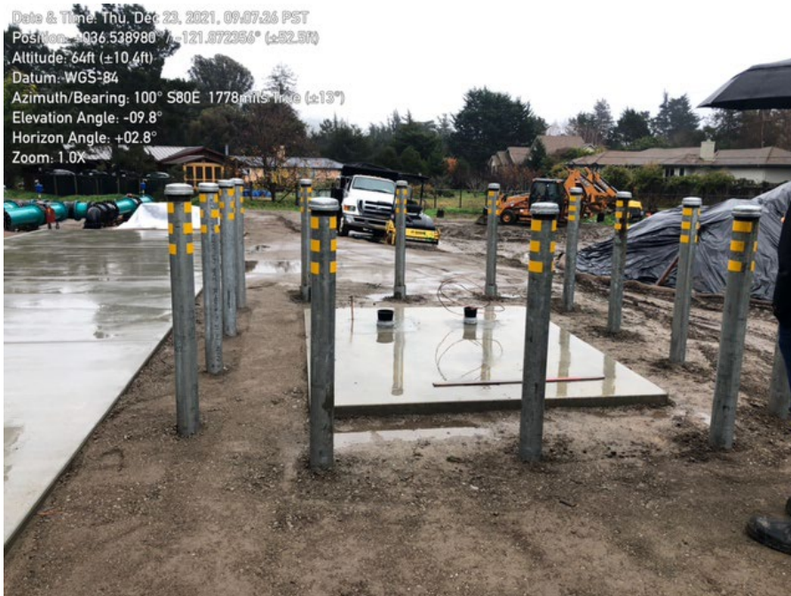
Photo 2. New transformer pad on south side of pump station.
