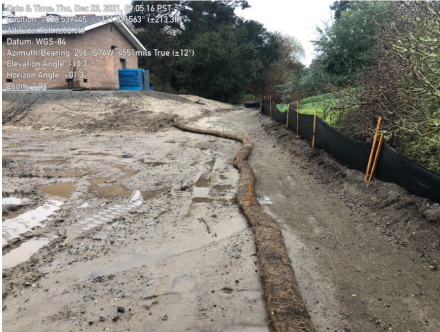
Photo 1. Monofilament straw wattle installed on site.
