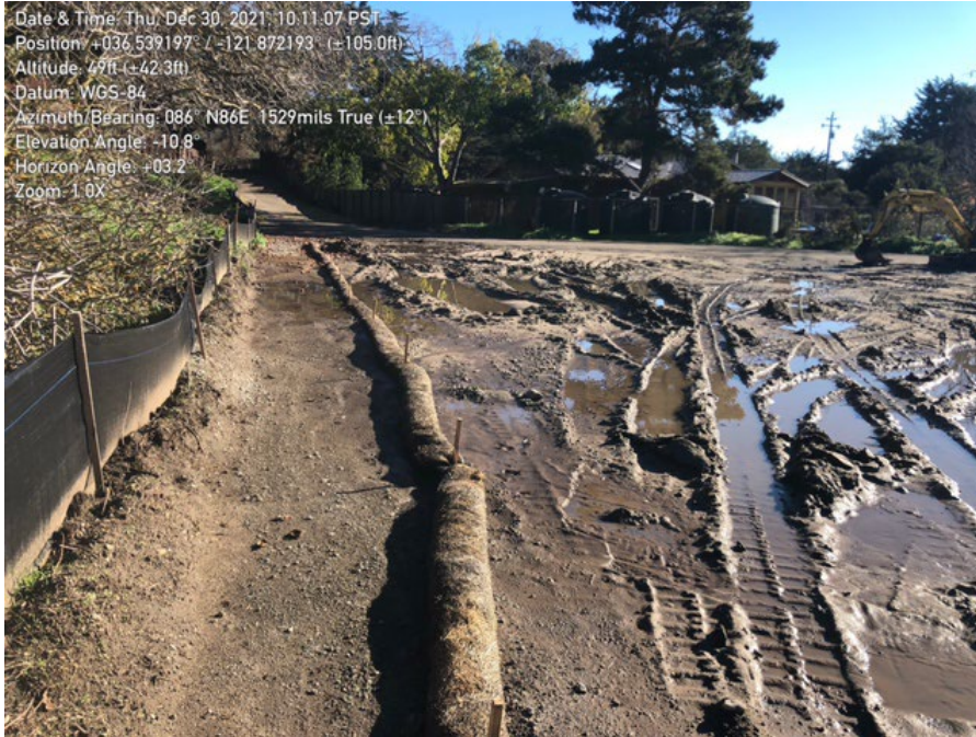
Photo 1. Monofilament straw wattle installed on site.
