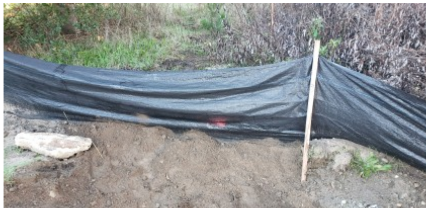
01/06/2022 - Exclusion fence reinstalled at v-ditch location.
