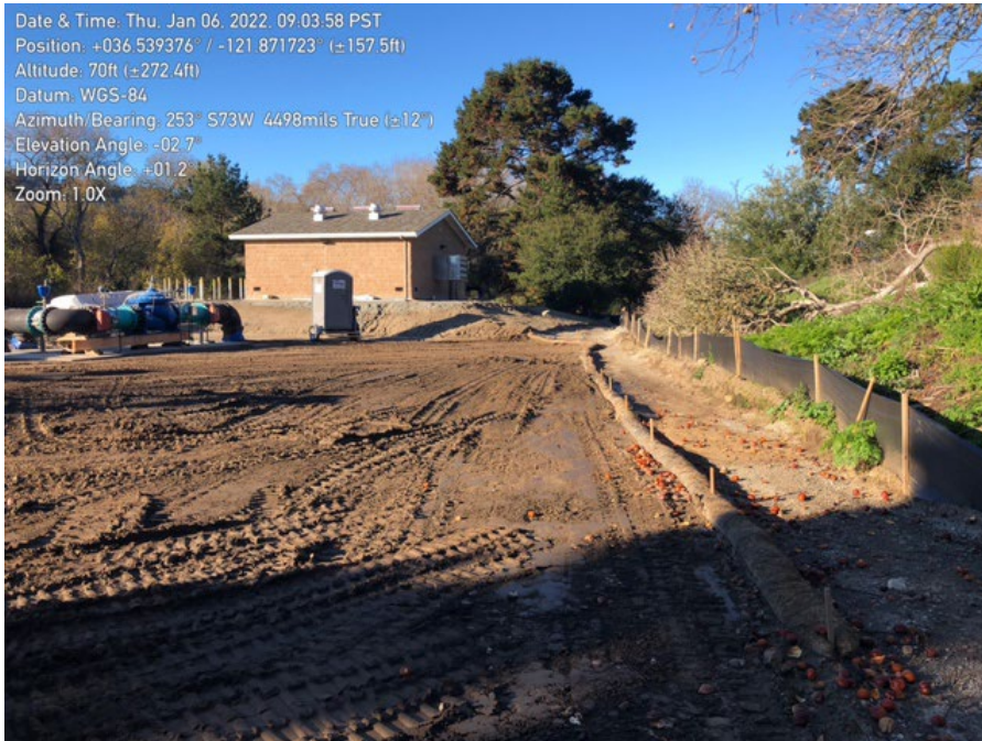
Photo 1. Monofilament straw wattle installed on site.
