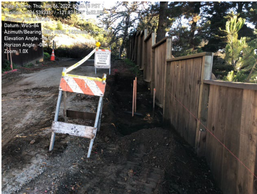
Photo 2. Retaining wall work.
