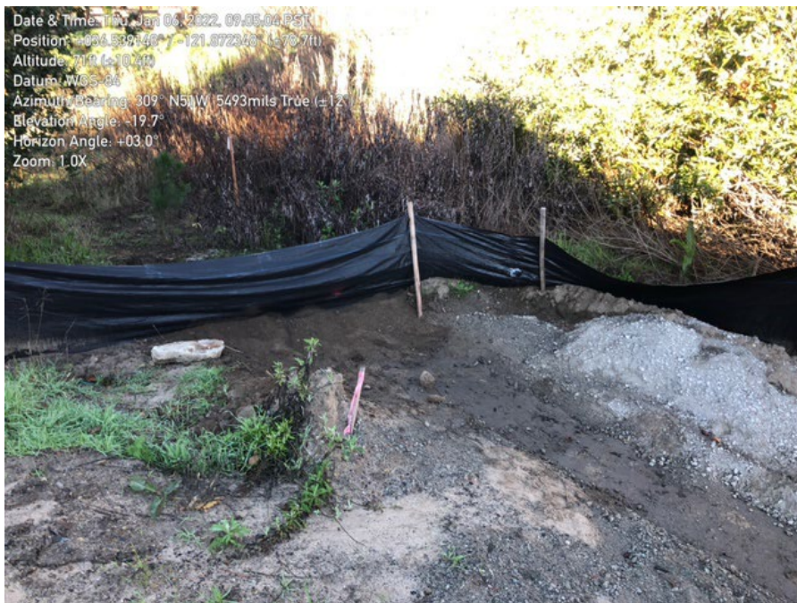
Photo 3. Silt fence in NW corner repaired.
