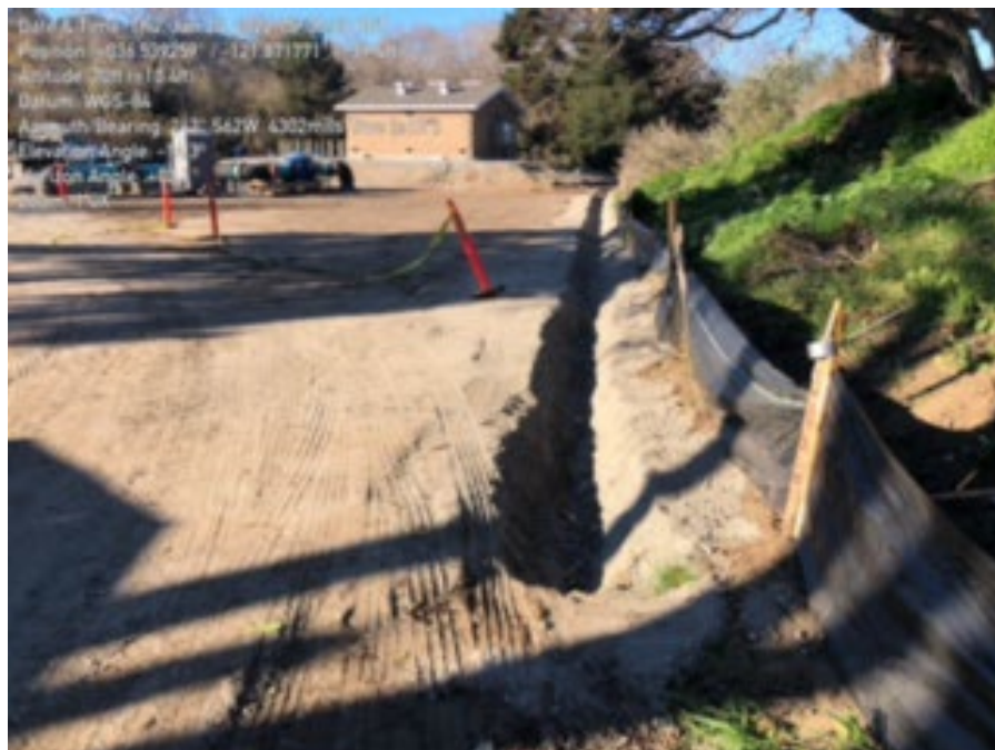
Photo 1. V-ditch installed within site boundary.
