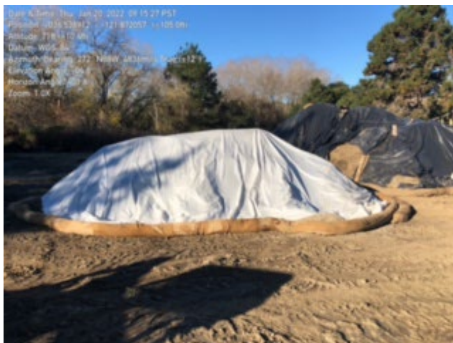
Photo 2. Spoils stock piles covered.
