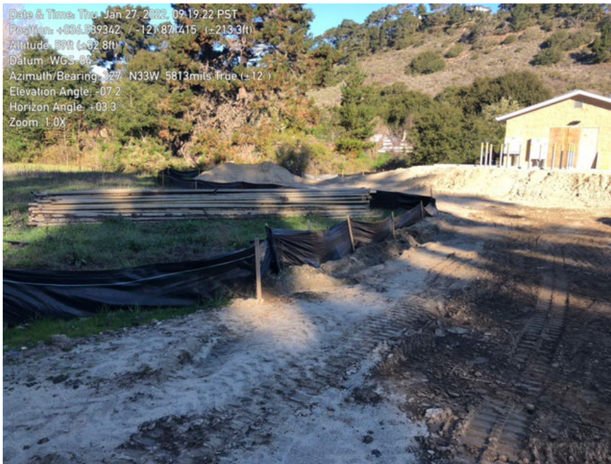
Photo 3. Silt fence in acceptable condition.
