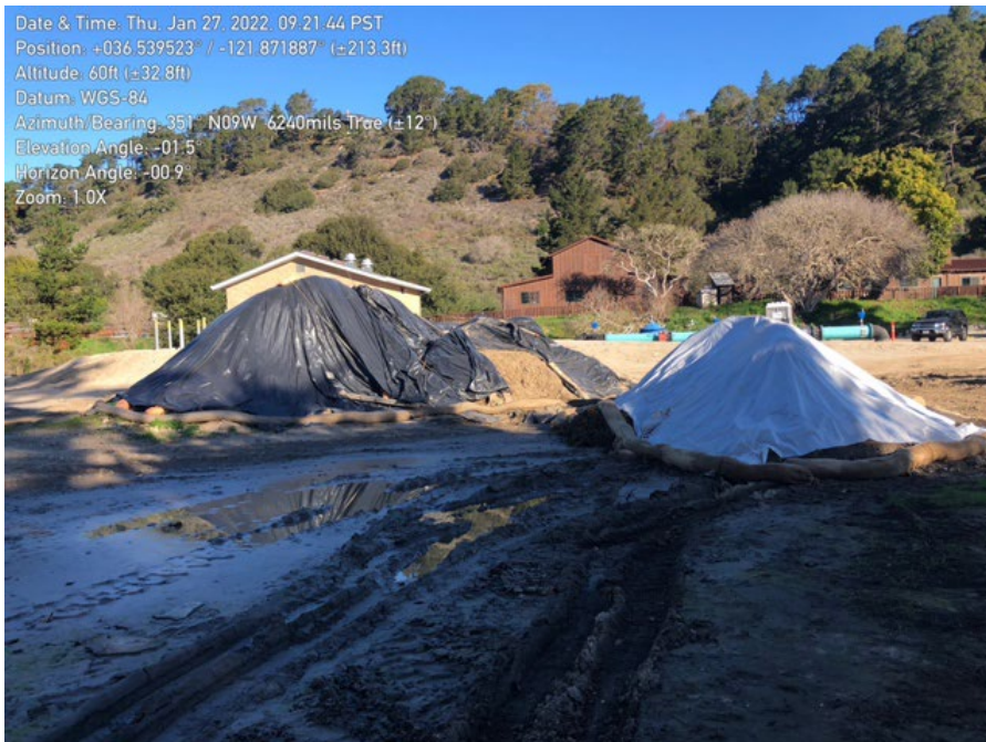
Photo 2. Spoils stock piles covered.
