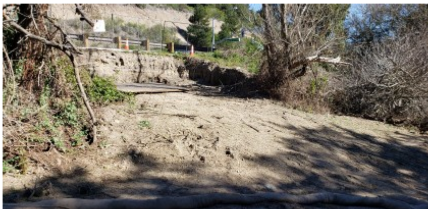
02/04/2022 - Carmel Valley Road tie in location.
