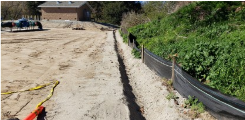
02/04/2022 - V ditch installation and exclusion fence.
