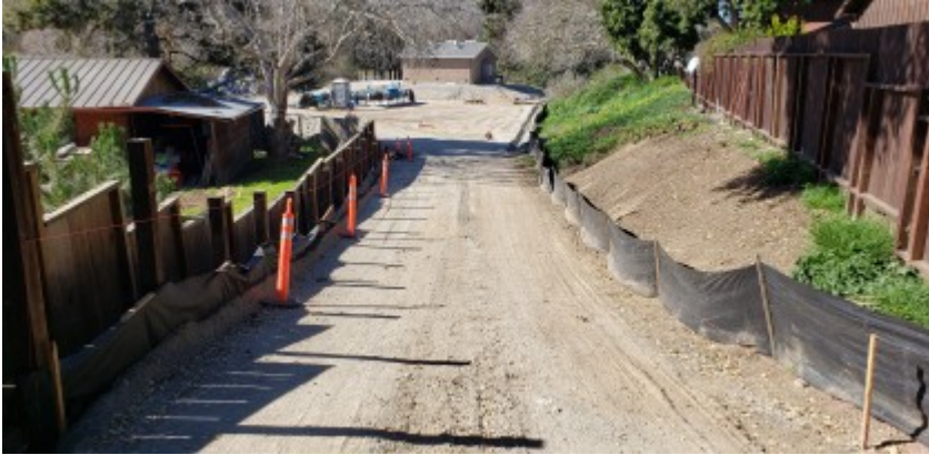
02/04/2022 - Site conditions - entrance.
