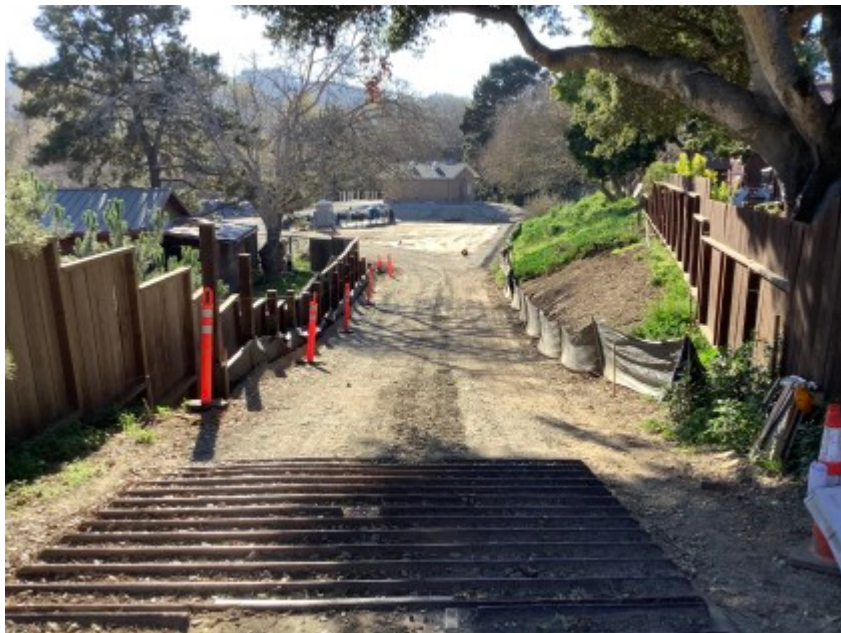
02/11/2022 - CVPS project site conditions. Access road.
