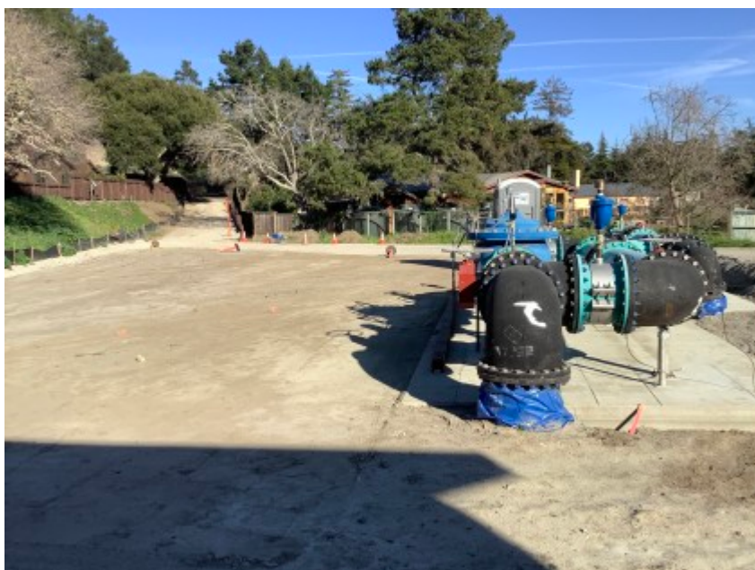
02/11/2022 - CVPS project site conditions.
