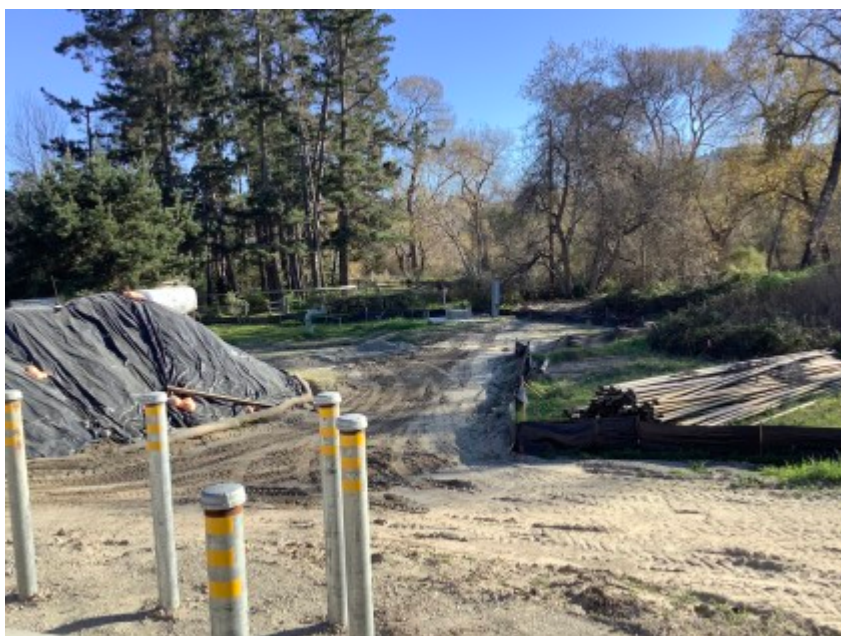
02/11/2022 - CVPS project site conditions. Intact exclusion fencing.
