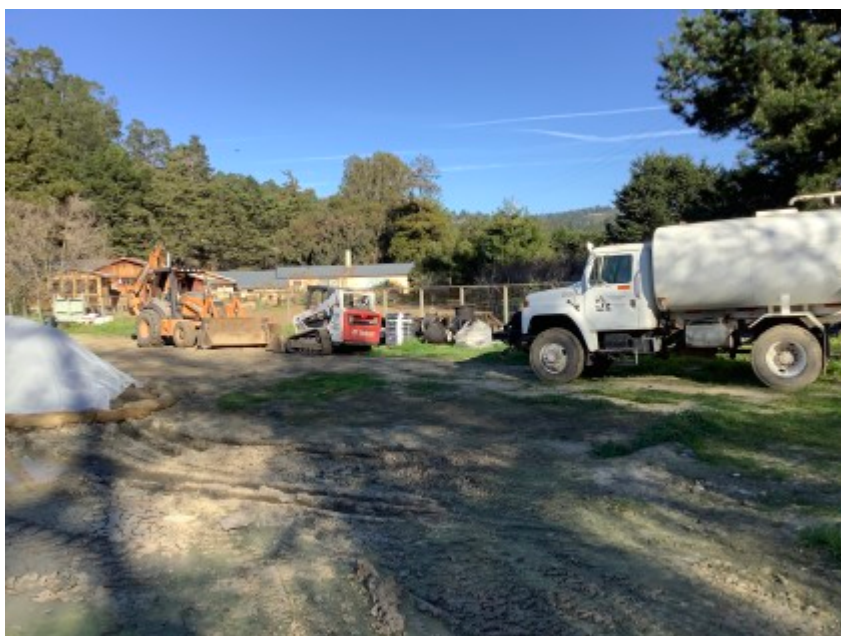
02/11/2022 - CVPS project site conditions. Staged equipment.
