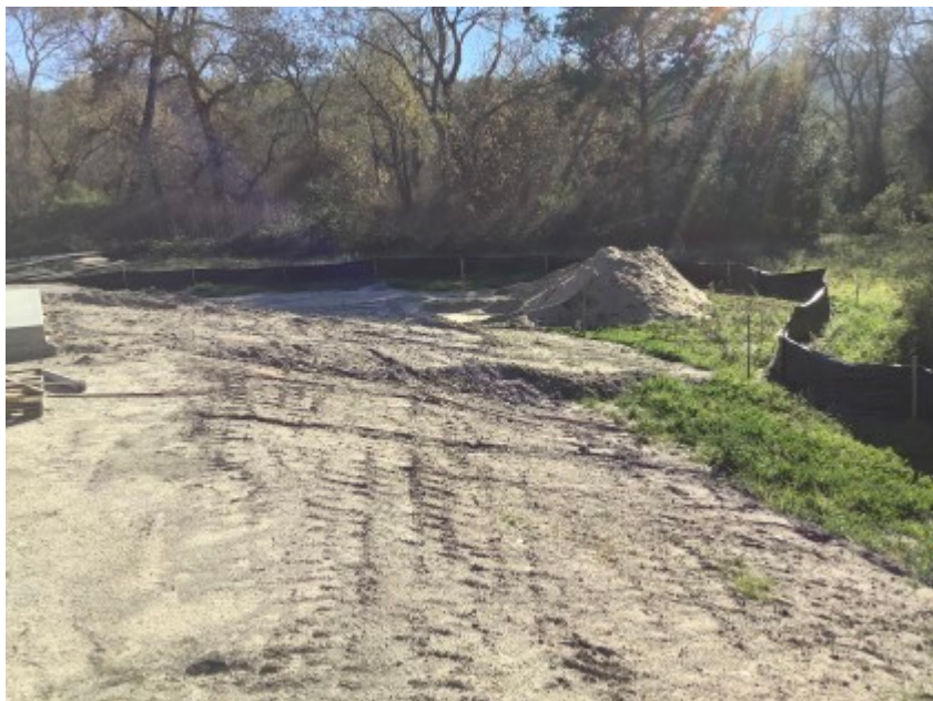
02/11/2022 - CVPS project site conditions. Intact exclusion fencing.
