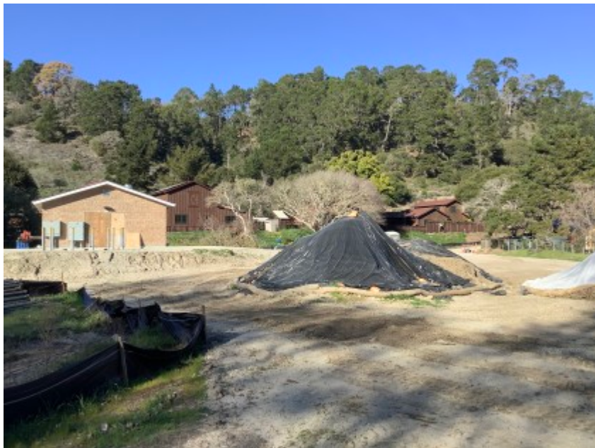
02/11/2022 - CVPS project site conditions.
