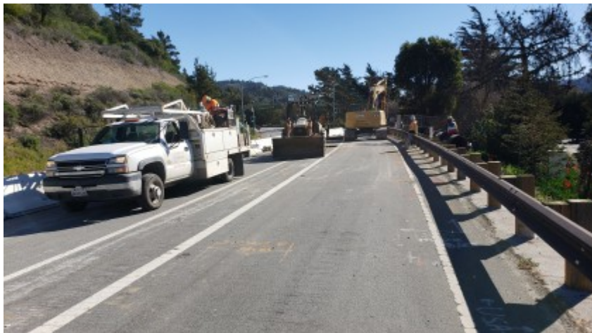
02/17/2022 - Carmel Valley Road traffic control and potholing.
