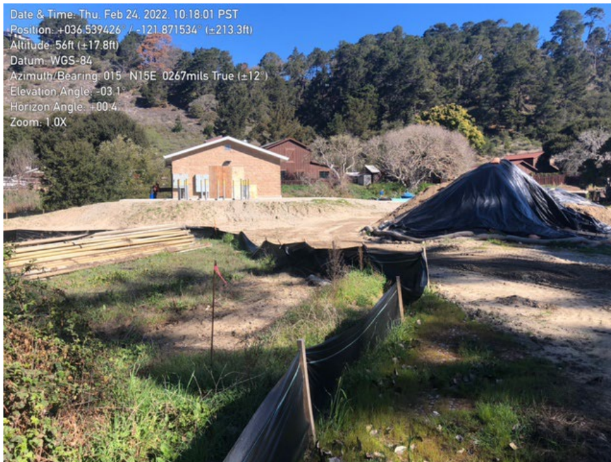
Photo 1. Overall site conditions.
