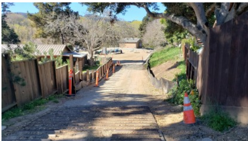
02/24/2022 - Project site access.
