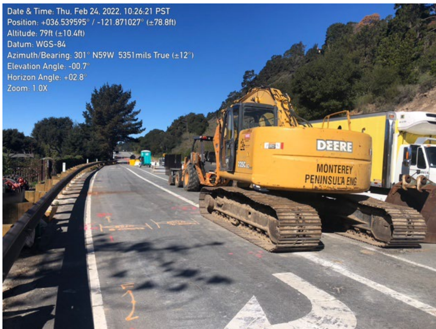
Photo 2. Equipment staged on Carmel Valley Road.
