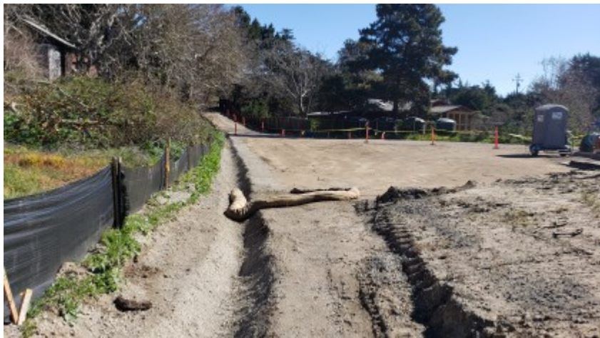
02/24/2022 - Project site conditions.
