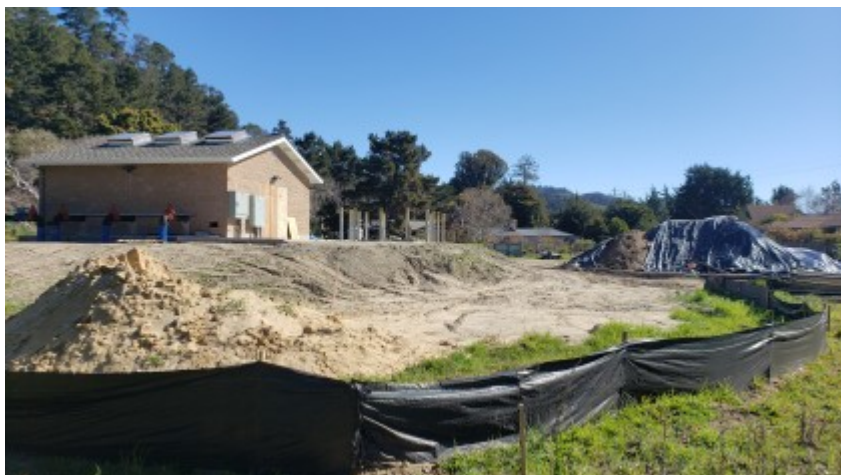
02/24/2022 - Project site conditions.
