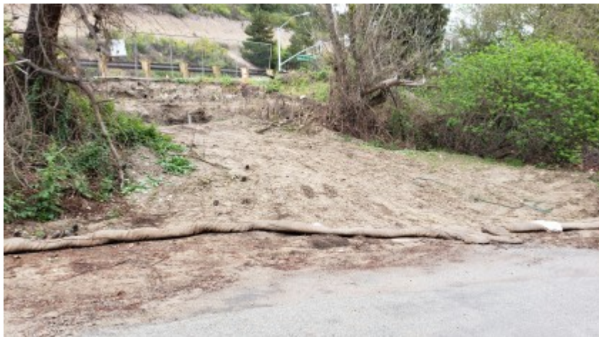
03/04/2022 - Carmel Valley Road Tie in.
