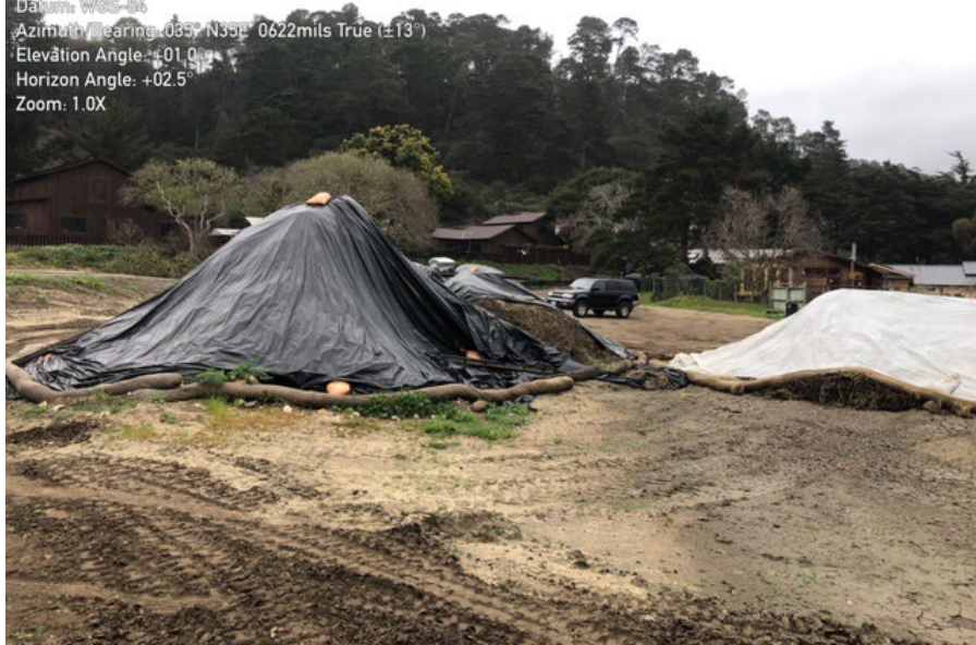
Photo 2. BMPs in place on spoils/materials.
