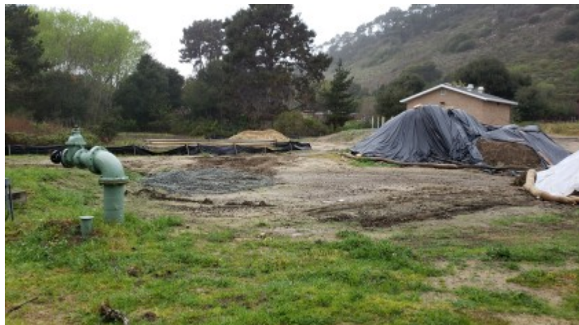
03/04/2022 - Project site conditions.
