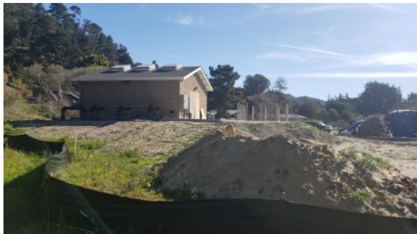
03/11/2022 - Project site conditions.
