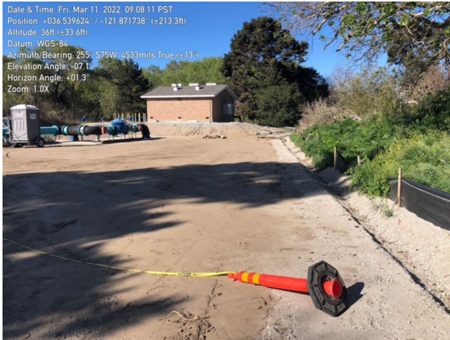
Photo 1. Overall site conditions.
