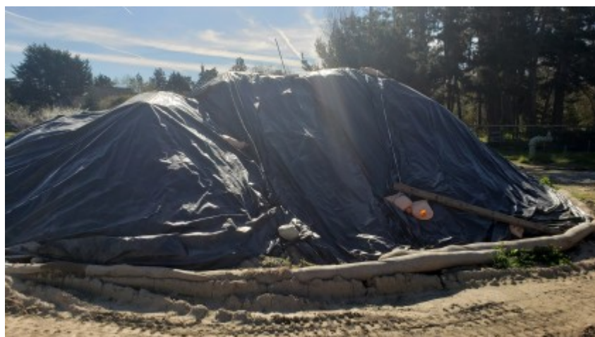
03/11/2022 - Erosion control in tact on spoils pile. DD&A performed maintenance on plastic sheeting.
