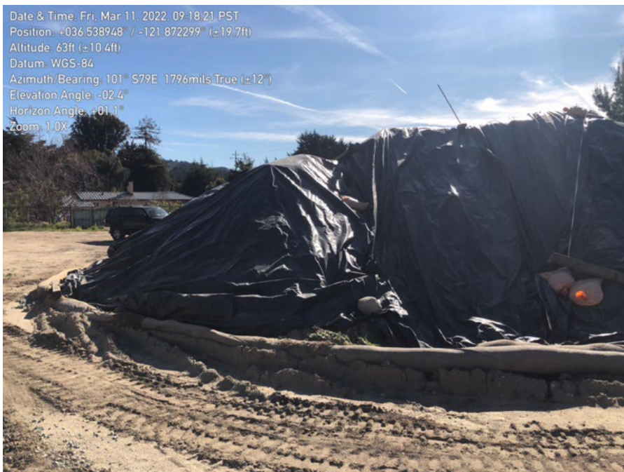
Photo 4. BMPs in place on spoils/materials.
