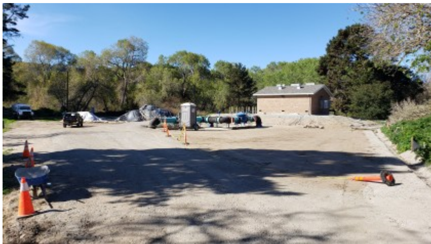
03/11/2022 - Project site conditions.
