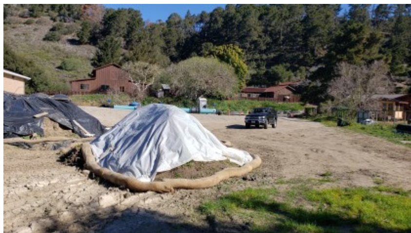
03/11/2022 - Erosion control on spoils pile.
