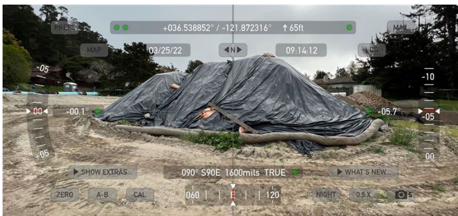
Photo 2. BMPs in place on spoils/materials.
