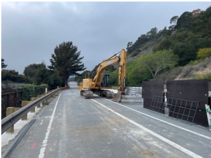
03/24/2022 - MPE equipment staged along Carmel Valley Road.
