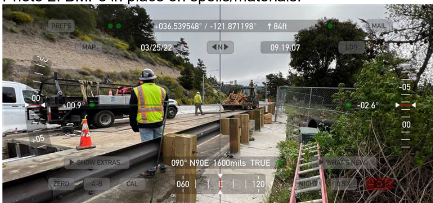
Photo 3. Construction activity on Carmel Valley Road tie-in
