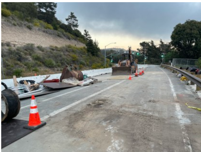
03/24/2022 - MPE equipment staged along Carmel Valley Road
