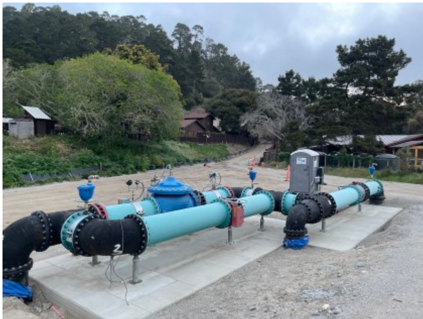
03/24/2022 - CVPS site conditions.
