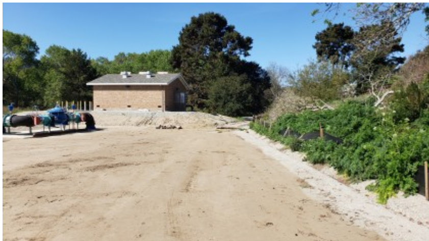
03/18/2022 - Project site conditions.
