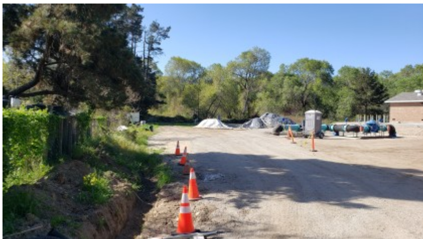
03/18/2022 - Project site conditions.
