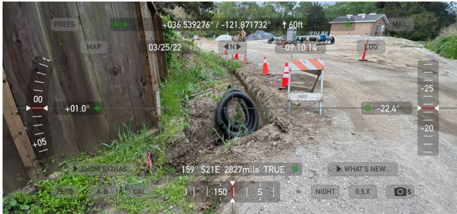
Photo 1. Overall site conditions.
