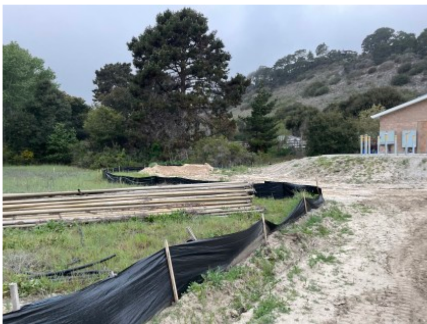
03/24/2022 - Intact exclusion fencing along western edge of CVPS.
