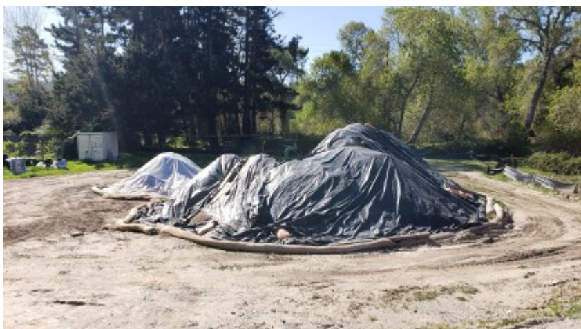
03/18/2022 - Erosion control intact on spoils piles.
