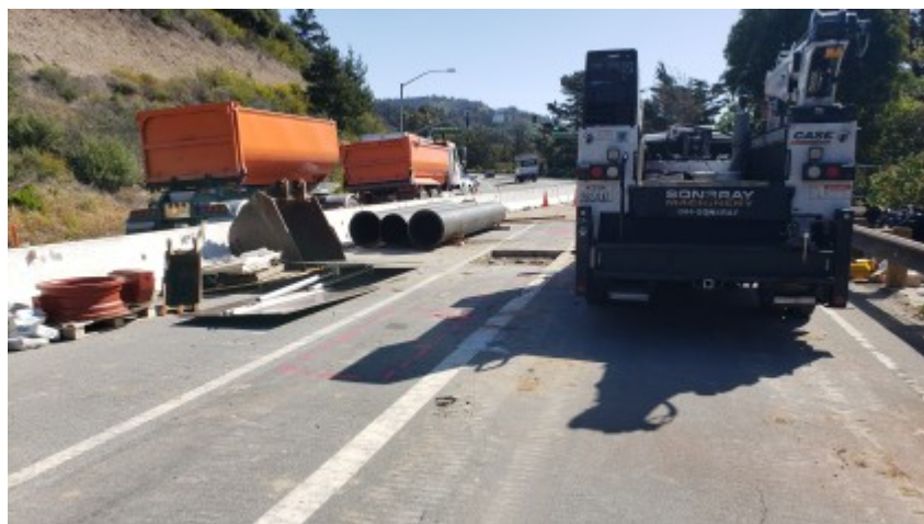
03/18/2022 - Carmel Valley Road tie-in traffic control.
