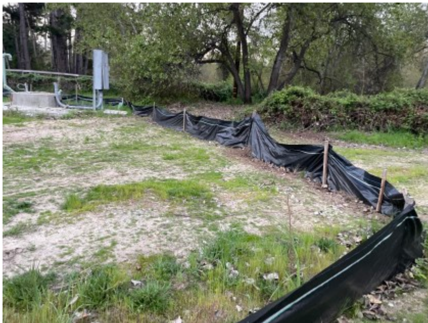
03/24/2022 - Intact exclusion fencing along southern edge of CVPS.
