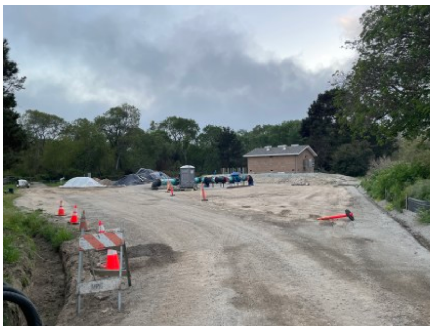
03/24/2022 - CVPS site conditions. Intact exclusion fencing on right side of photo.
