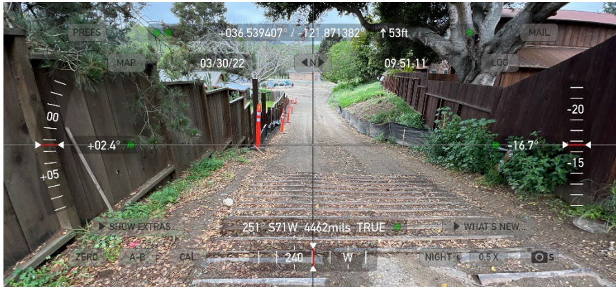
Photo 1. Overall site conditions.
