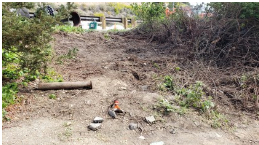
03/31/2022 - Area cleared for Carmel Valley Road tie in.
