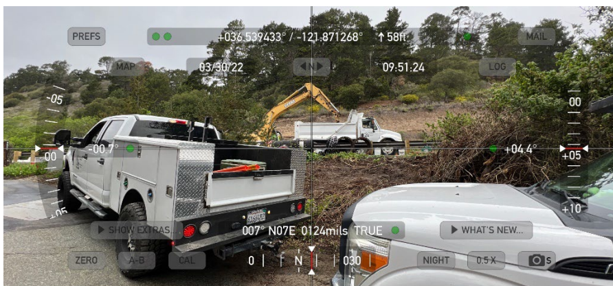
Photo 3. Construction activity on Carmel Valley Road tie-in
