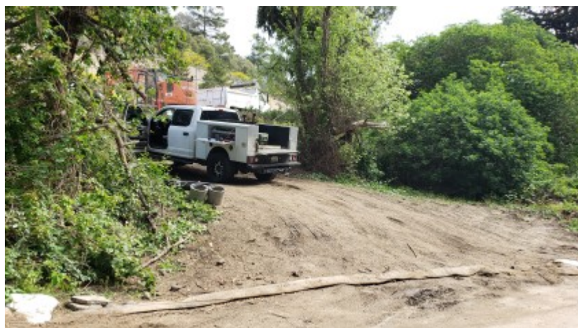
03/31/2022 - Carmel Valley Road tie in.
