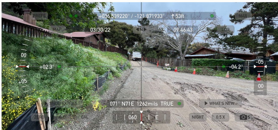
Photo 2. Active haul truck off-loading soil.
