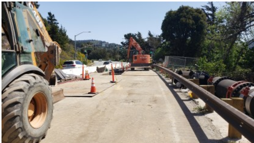
04/06/2022 - Installation of saddle on pipeline for tie-in.
