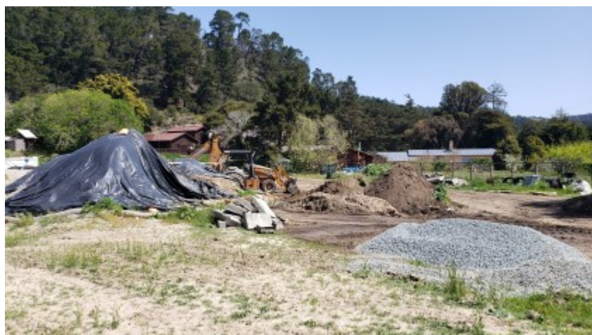
04/06/2022 - Staged spoils from tie-in installation will be covered at the end of the day.
