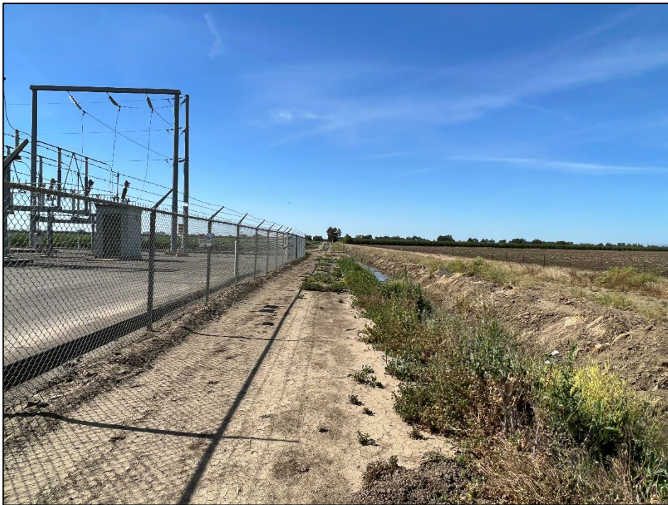
Photograph 8: Substation and Ditch 1. South aspect. 5/18/22
