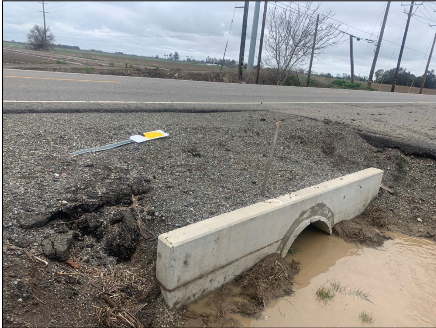
Photograph 2: Culvert 1 underneath County Road 27. Northeast aspect. 3/22/23
