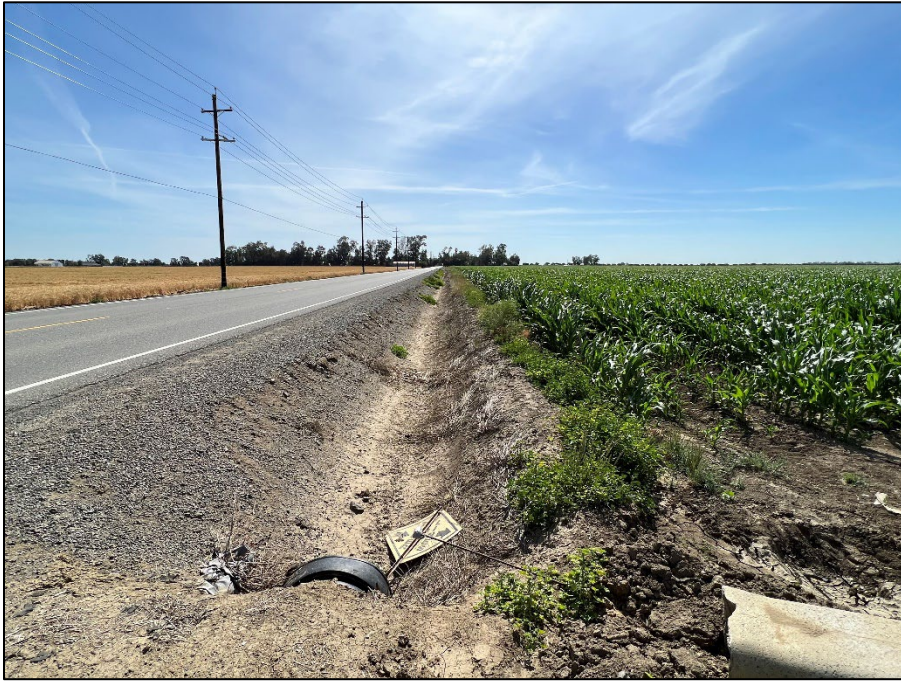
Photograph 9: Ditch 2a and adjacent agricultural field. East aspect. 5/18/22
