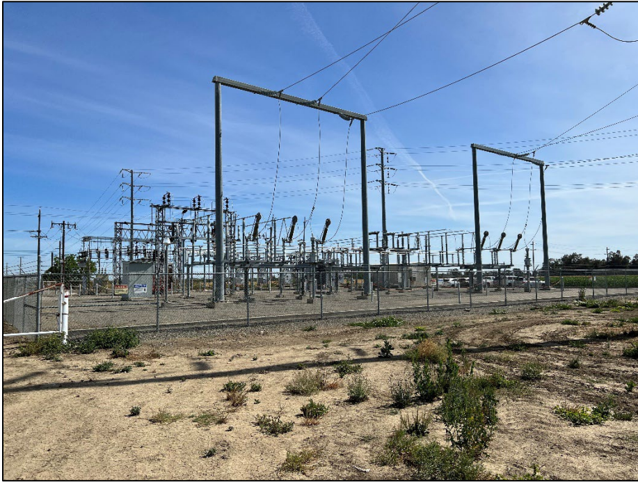
Photograph 7: Project Area from the southwest corner of the substation. Northeast aspect. 5/18/22
