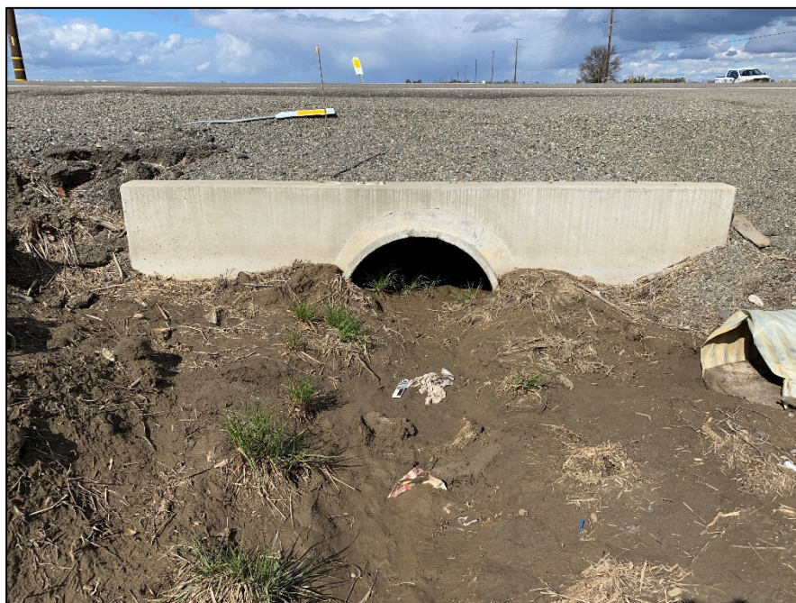
Photograph 4: P-57-001575/CA-YOL-278H, modern culvert under County Road 27 on 3/7/2023, facing north.
