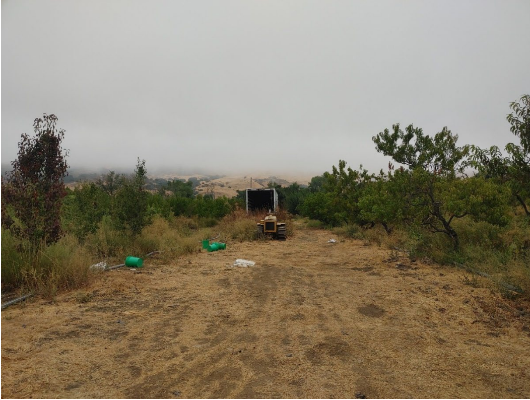
Image 11. Overview of Grove terminal, facing northeast (9/12/2023)
