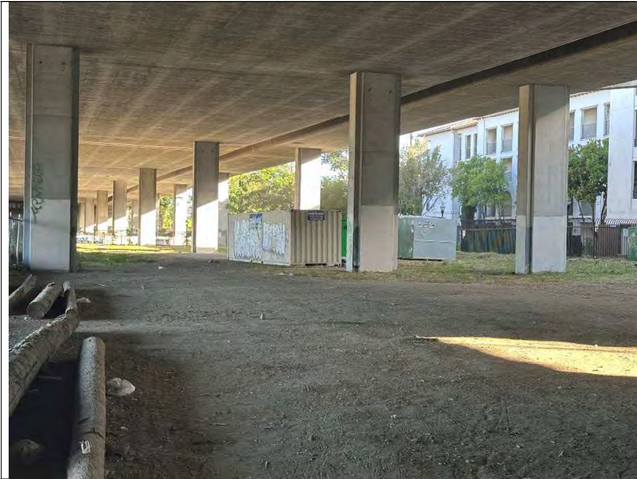
Photo 7: North-facing view of existing shipping containers within the MPR-2 work area.
