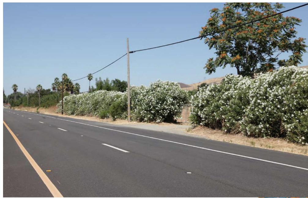
Adjacent to Grove Terminal
