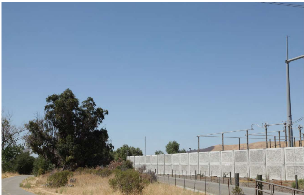
Adjacent to Metcalf Substation
