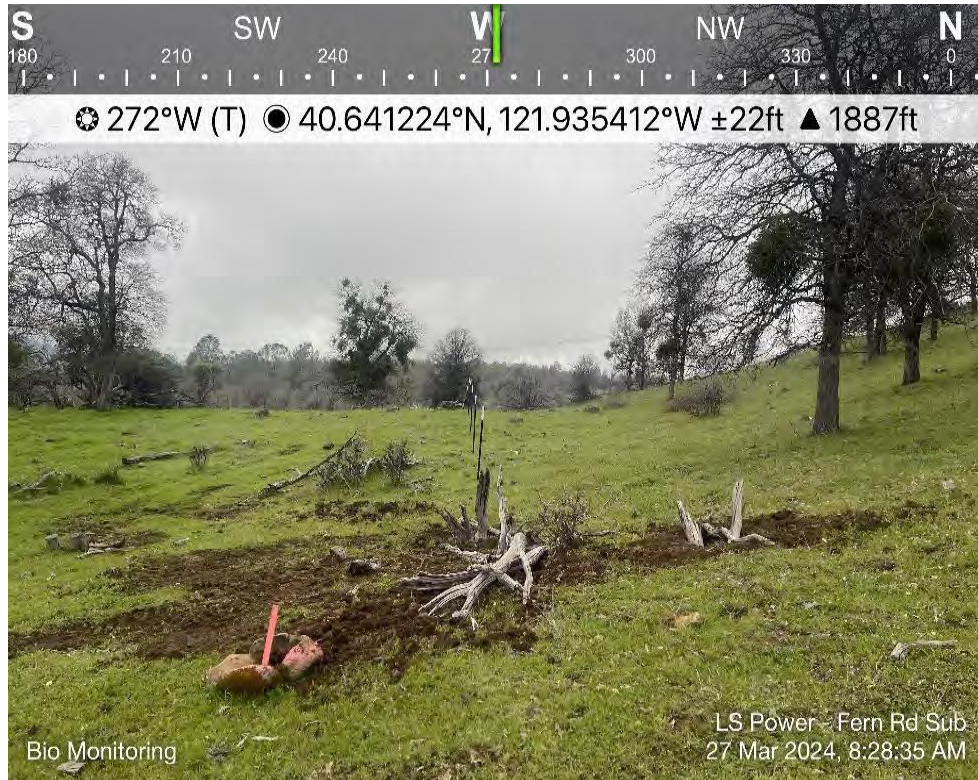
Photo 21. View of southeast corner of fence installation. Direction: Northwest. Date: 3/27/2024
