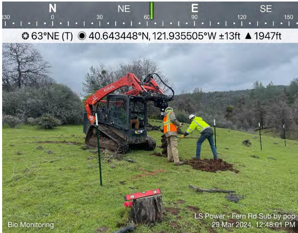
Photo 25. View of the last post hole to be dug with an auger. Direction: Southwest. Date: 3/29/2024
