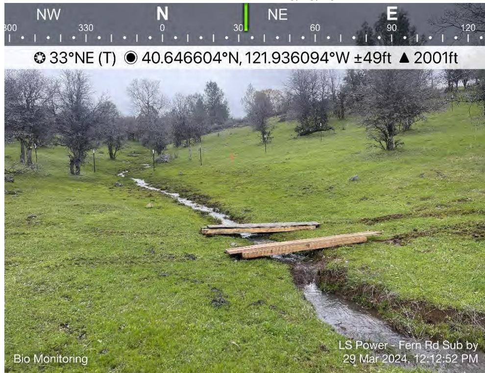
Photo 27. View of temporary crossing of intermittent stream for the fence crew's equipment. Direction: South. Date: 3/29/2024
