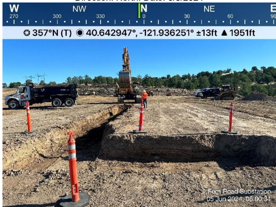
Photo 16. View of TTR excavating footing trenches around control enclosure pad.
