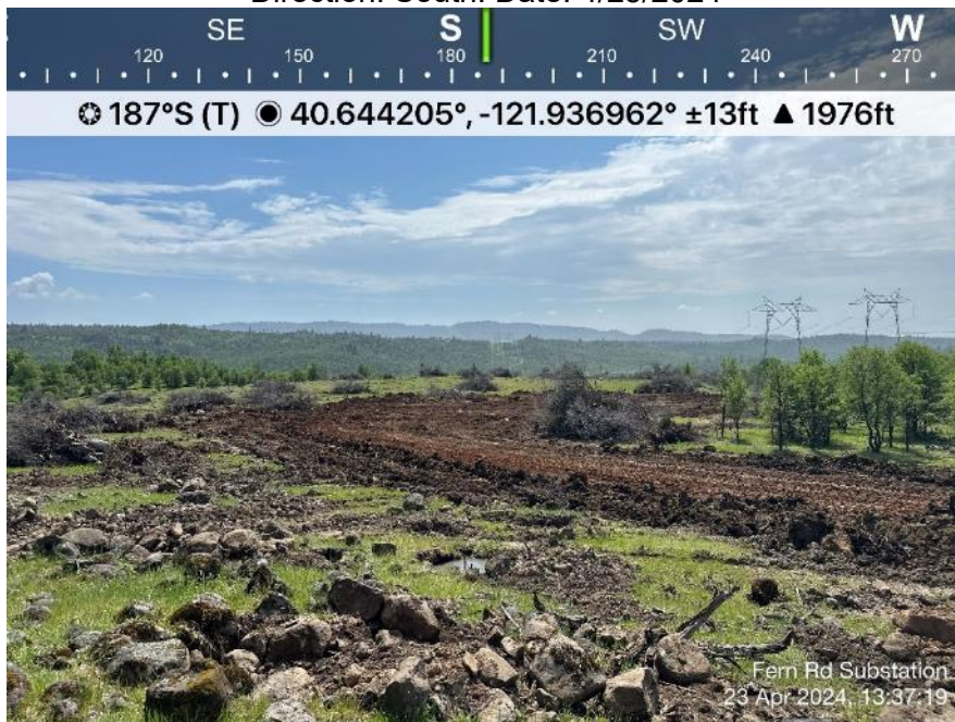
Photo 12. View of access road and main substation pad area. Direction: South. Date: 4/25/2024
