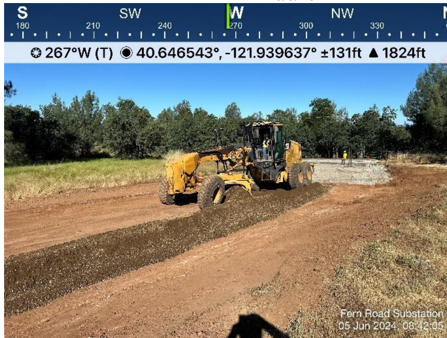
Photo 17. View of grader spreading base on the access road. Direction: West. Date: 6/5/2024
