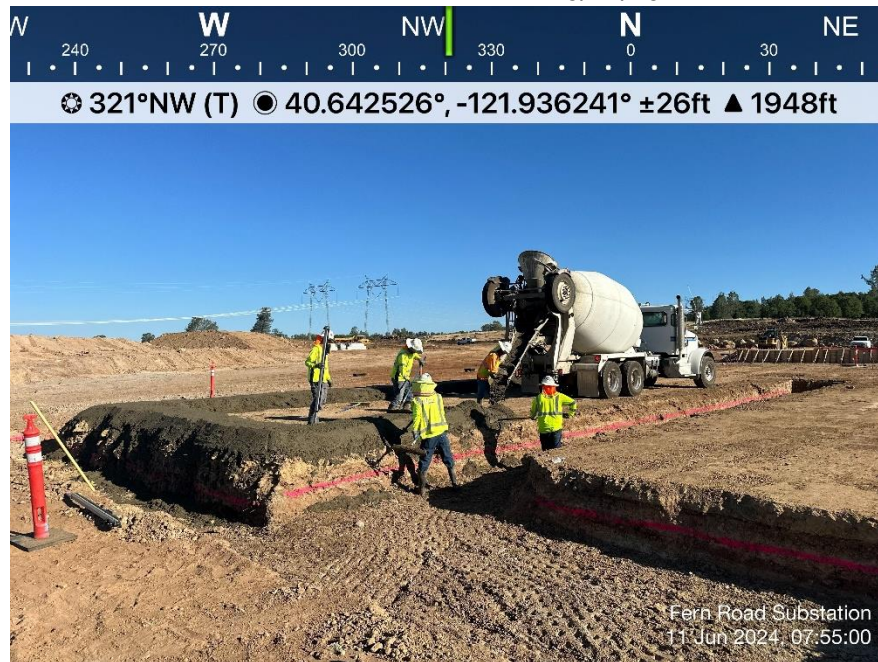
Photo 19. View of TTR slurry pour at control enclosure 2. Direction: Northwest. Date: 6/11/2024
