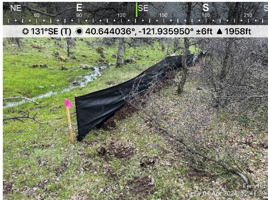
Photo 4. View of silt fence installation start on eastern perimeter.
