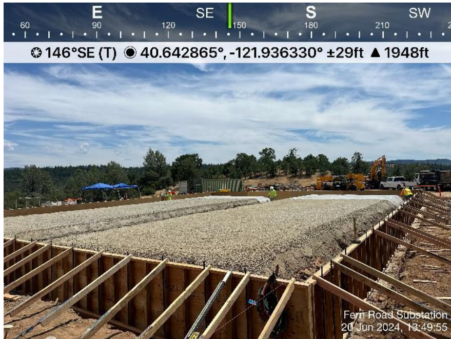
Photo 22. View of TTR installing vapor barrier at control enclosure 2. Direction: Southeast. Date: 6/20/2024
