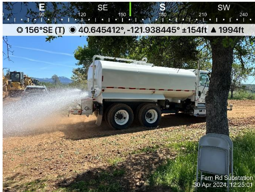
Photo 13. View of TTR water truck doing dust control. Direction: Southeast. Date: 4/30/2024
