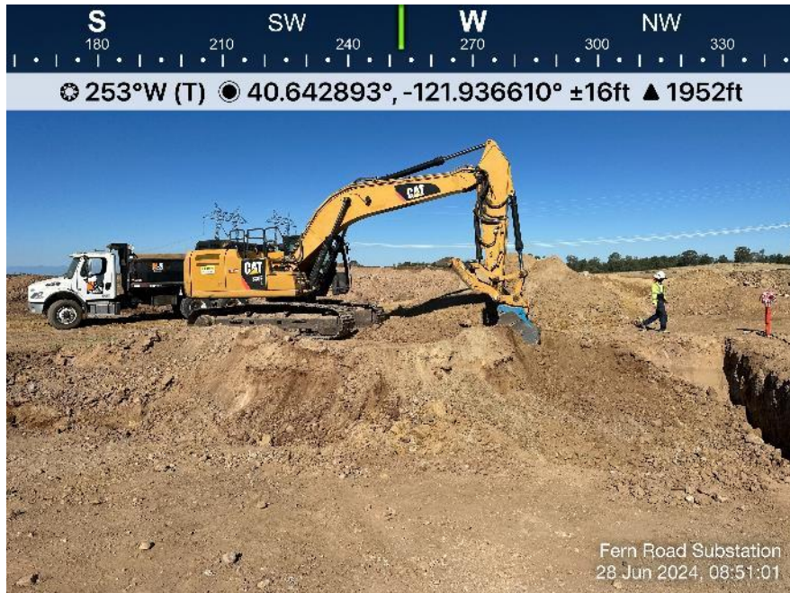
Photo 24. View of TTR excavating the transformer foundation pit for transformer 2. Direction: West. Date: 6/28/2024
