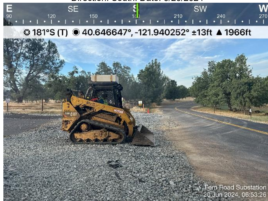
Photo 20. View of TTR cleaning up rock and track out from construction entrance on Fern Road. Direction: South. Date: 6/20/2024
