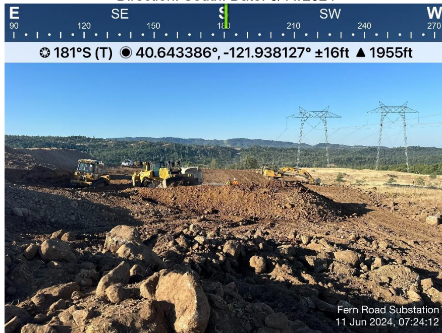
Photo 18. View of TTR conditioning soil for fill and compaction in SW corner. Direction: South. Date: 6/11/2024
