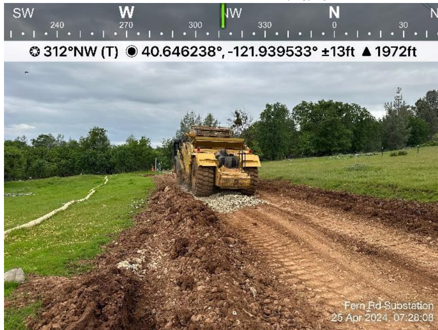
Photo 11. View of TTR scraper depositing rock on access road. Direction: Northwest. Date: 4/25/2024
