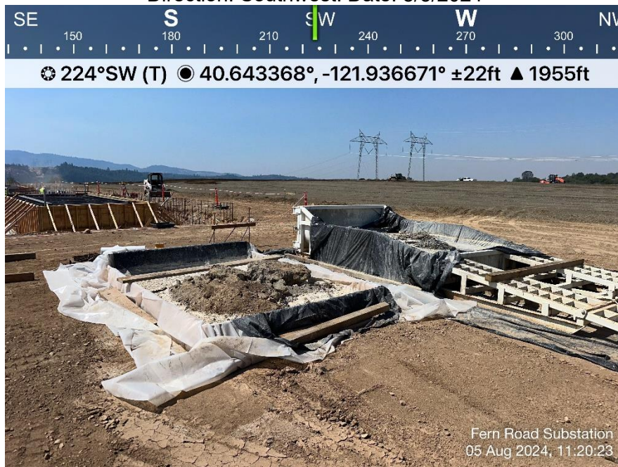
Photo 14. View of TTR concrete washout after clean up. Direction: Southwest. Date: 8/5/2024
