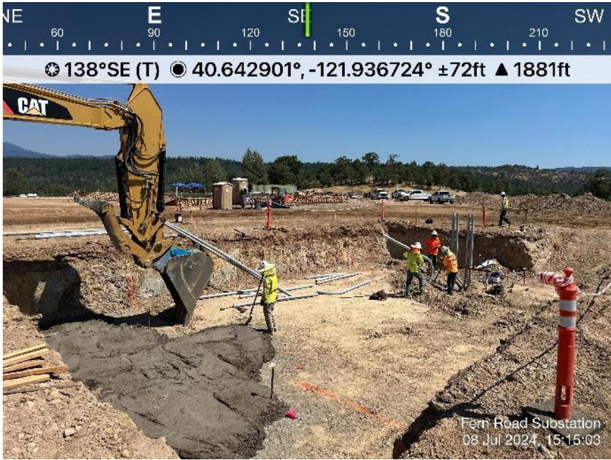
Photo 4. View of TTR crew installing conduit in transformer 2 (T2) foundation pit. Direction: Southeast. Date: 7/8/2024
