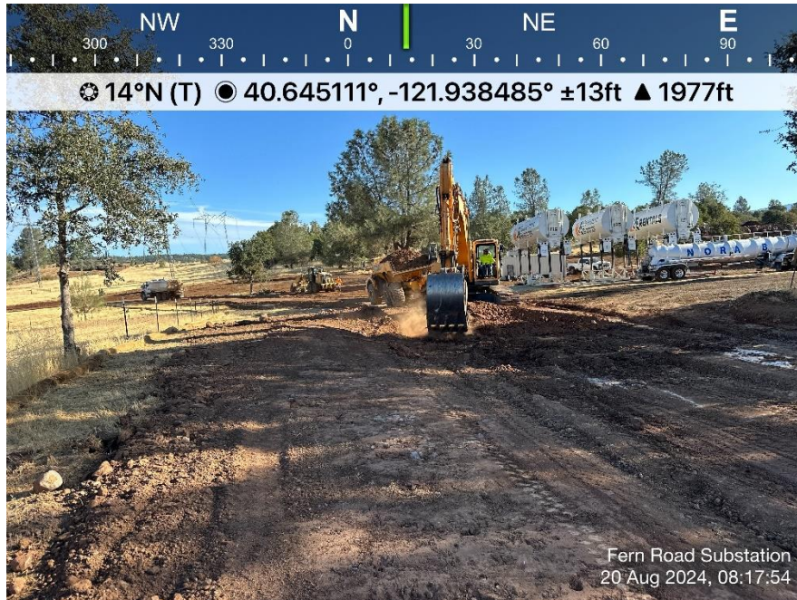
Photo 17. View of TTR working on swales around the laydown yard pad. Direction: North. Date: 8/20/2024
