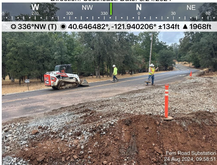
Photo 20. View of TTR scraping and brushing track-out from Fern Road at construction entrance. Direction: Southeast. Date: 8/24/2024
