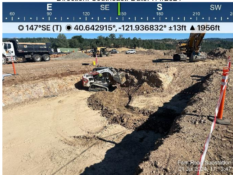
Photo 2. View of TTR skid steer trenching for conduit in transformer 1 (T1) foundation pit.
