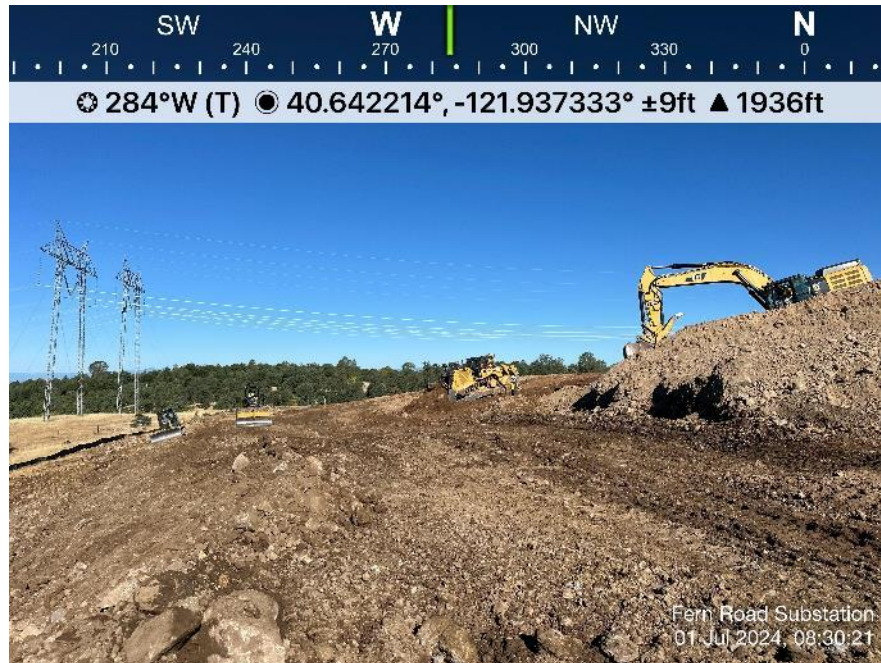
Photo 2. View of TTR skid steer trenching for conduit in transformer 1 (T1) foundation pit.
