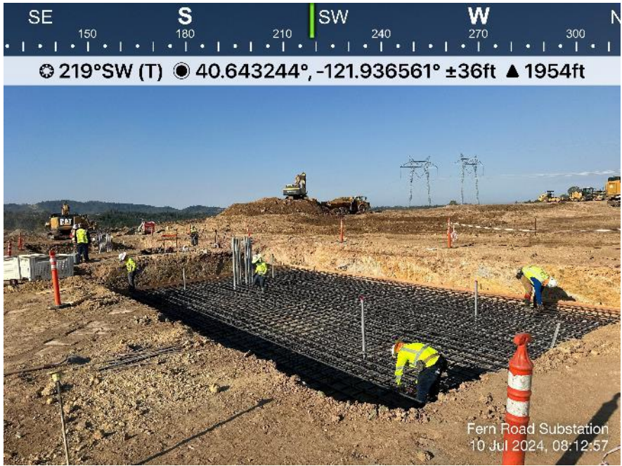
Photo 5. View of TTR crew fine tuning foundation framing and rebar install in T1 foundation pit. Direction: Southwest. Date: 7/10/2024
