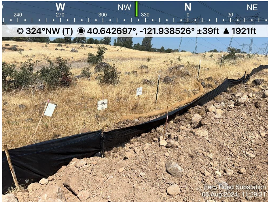
Photo 15. View of repaired silt fence on western perimeter. Direction: Northwest. Date: 8/5/2024
