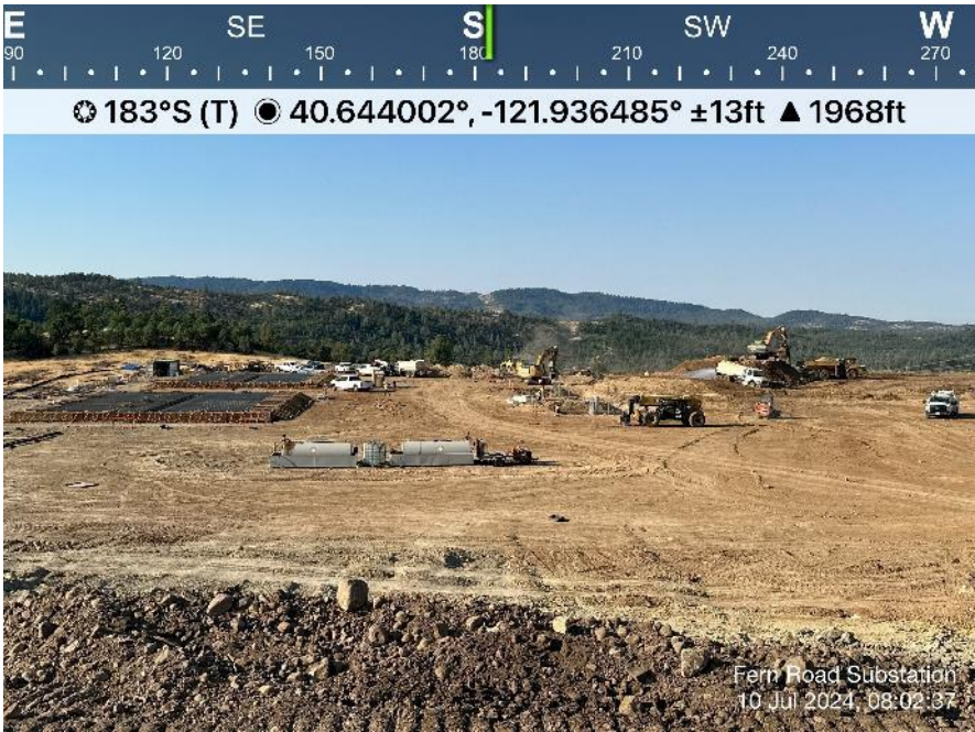
Photo 6. Overview of substation pad showing control enclosure #1 and #2 foundation frame ups on the left, T1, T2, & transformer 3 (T3) pits just right of center, and excess soil pile on the right.
