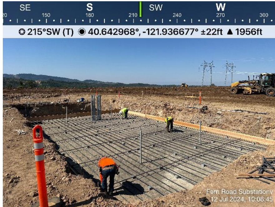
Photo 9. View of TTR installing a layer of rebar into the T2 foundation framing. Direction: Southwest. Date: 7/12/2024
