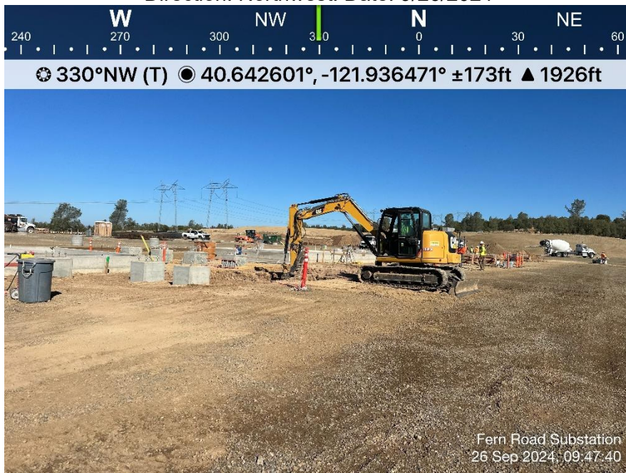
Photo 24. View of TTR excavating substation component foundation pit. Direction: Northwest. Date: 9/26/2024
