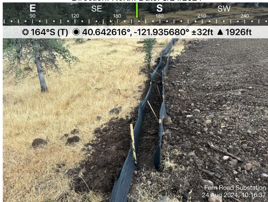
Photo 22. View of silt fence at low point showing no offsite discharge. Direction: North. Date: 8/24/2024
