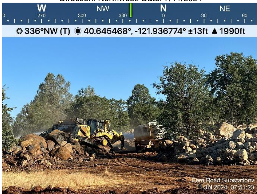
Photo 8. View of TTR crew starting to push rock up farther into expanded storage area. Direction: Northwest. Date: 7/11/2024
