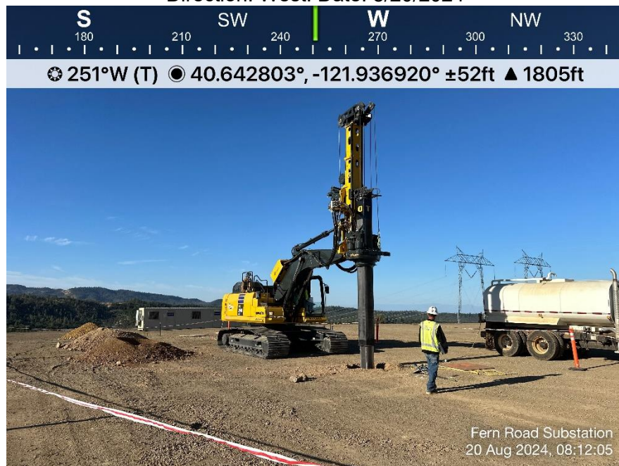
Photo 16. View of Komatsu drill rig drilling pier holes in substation pad. Direction: West. Date: 8/20/2024
