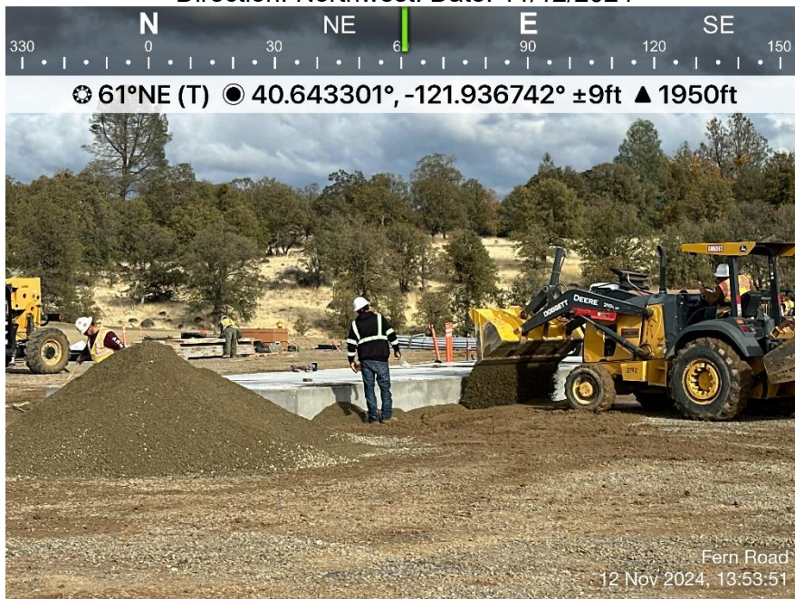
Photo 12. View of Dacon crew backfilling around foundation of PGE control building. Direction: Northwest. Date: 11/12/2024
