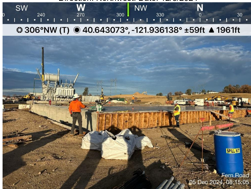
Photo 16. View of TTR stripping forms from outside of Control Enclosure 1 foundation.
