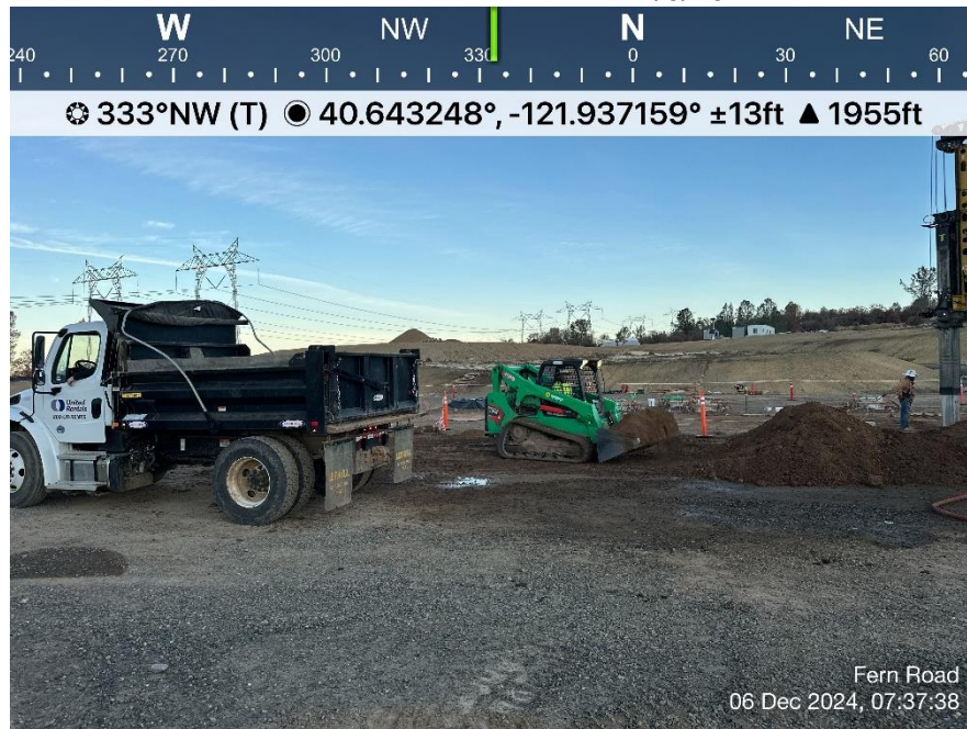
Photo 22. View of TTR crew excavating conduit and ground trenches in GIS building foundation. Direction: South. Date: 12/6/2024
