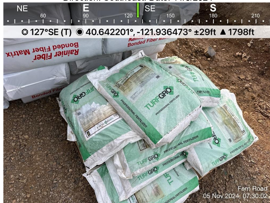
Photo 8. View of bonded fiber matrix and fertilizer for upcoming hydroseeding. Direction: Southeast. Date: 11/5/2024
