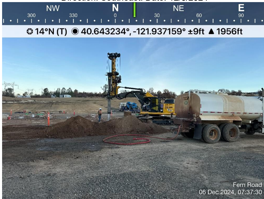
Photo 20. View of TTR crew drilling dead-end pier foundation holes on substation pad. Direction: Southeast. Date: 12/6/2024
