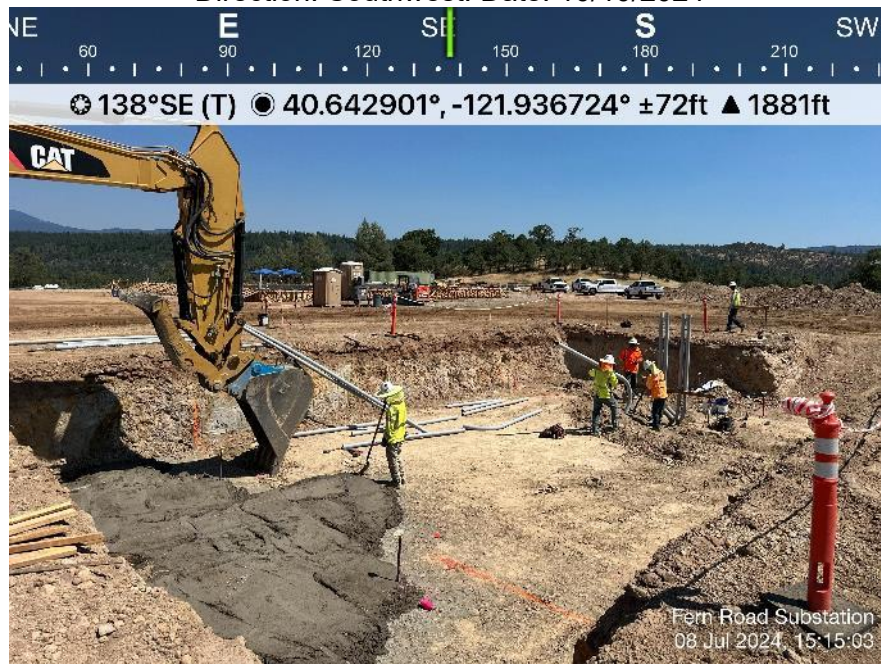
Photo 4. View of TTR installing tying in rebar for the GIS building foundation footings. Direction: Southwest. Date: 10/10/2024
