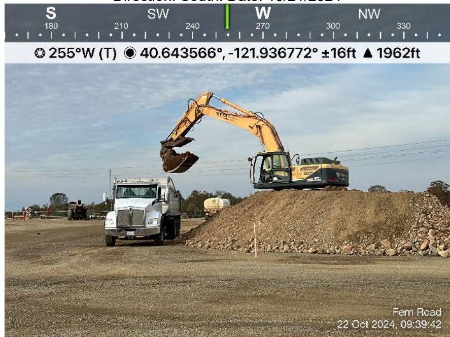
Photo 6. View of TTR loading spoil stockpile into trucks for off-hauling. Direction: South. Date: 10/21/2024
