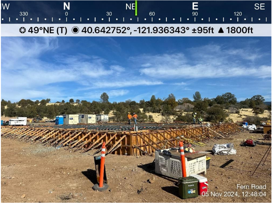
Photo 10. View of TTR pouring concrete in 3-foot pier foundations.
