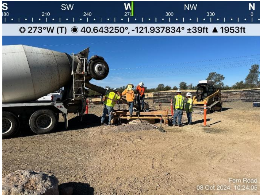
Photo 1. View of TTR pouring concrete at pier foundation on northwest side of substation pad. Direction: West. Date: 10/8/2024
