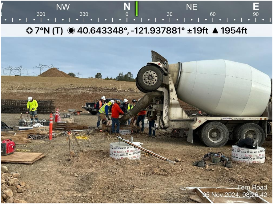
Photo 10. View of TTR pouring concrete in 3-foot pier foundations.
