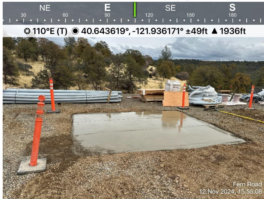
Photo 14. View of Dacon crew working on PGE generator and propane tank concrete pad forms.
