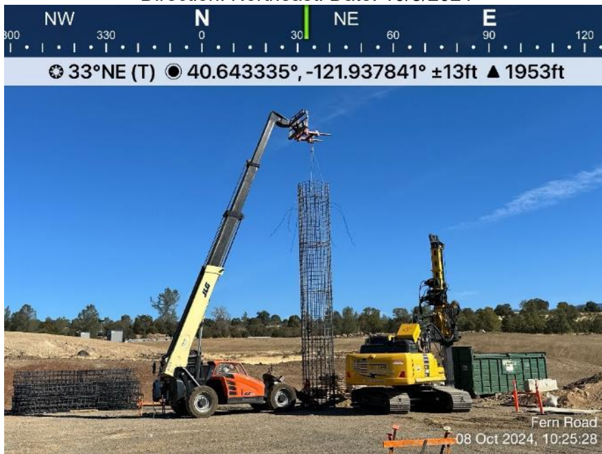
Photo 2. View of TTR installing a pier foundation rebar cage and drilling. Direction: Northeast. Date: 10/8/2024
