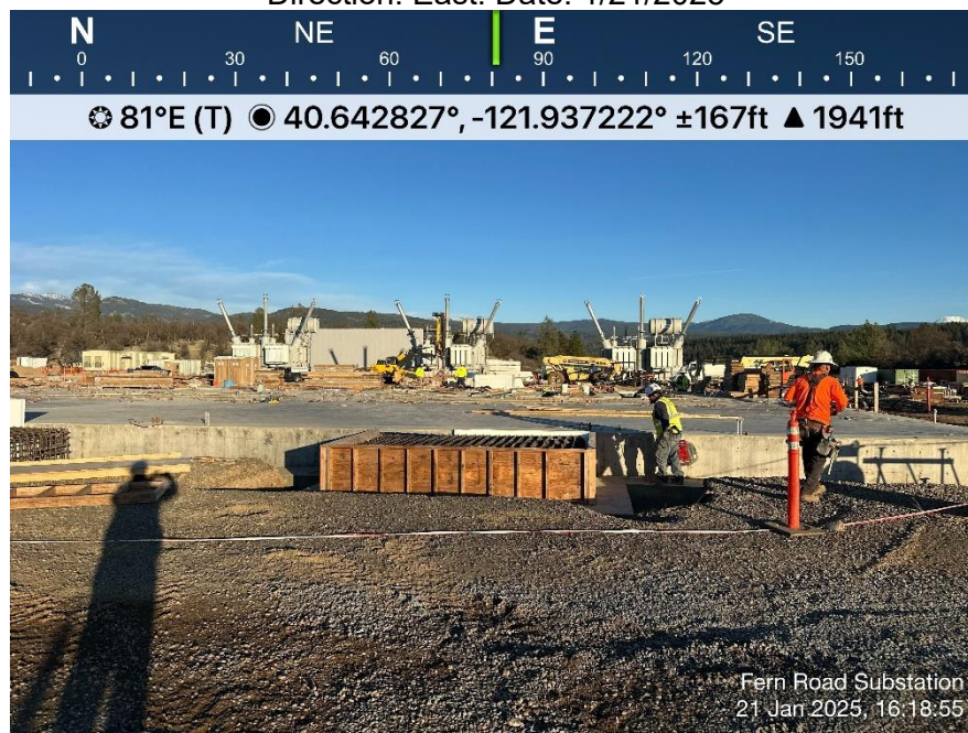
Photo 2. View of TTR constructing concrete forms for foundations around the GIS building foundation slab.
