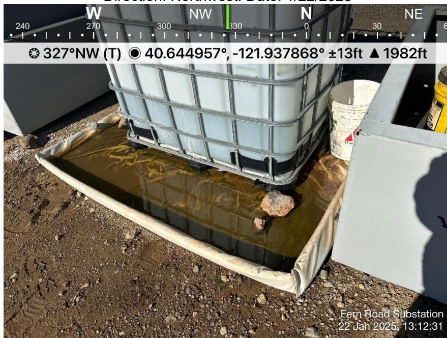
Photo 14. View of stormwater in secondary containment of DEF container. Direction: Northwest. Date: 1/22/2025
