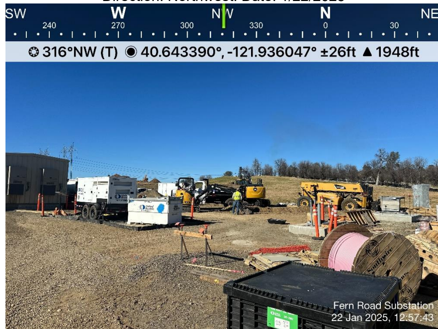
Photo 8. View of the Dacon crew digging in the PGE portion of the substation pad. Direction: Northwest. Date: 1/22/2025
