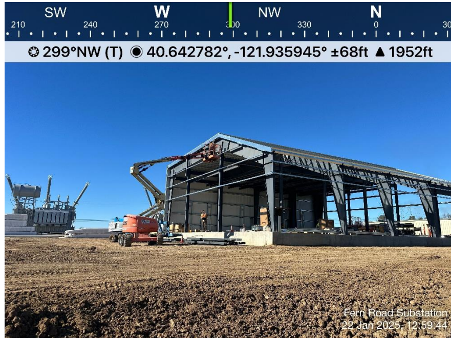
Photo 7. View of Siemens crew installing siding on control enclosure #1. Direction: Northwest. Date: 1/22/2025
