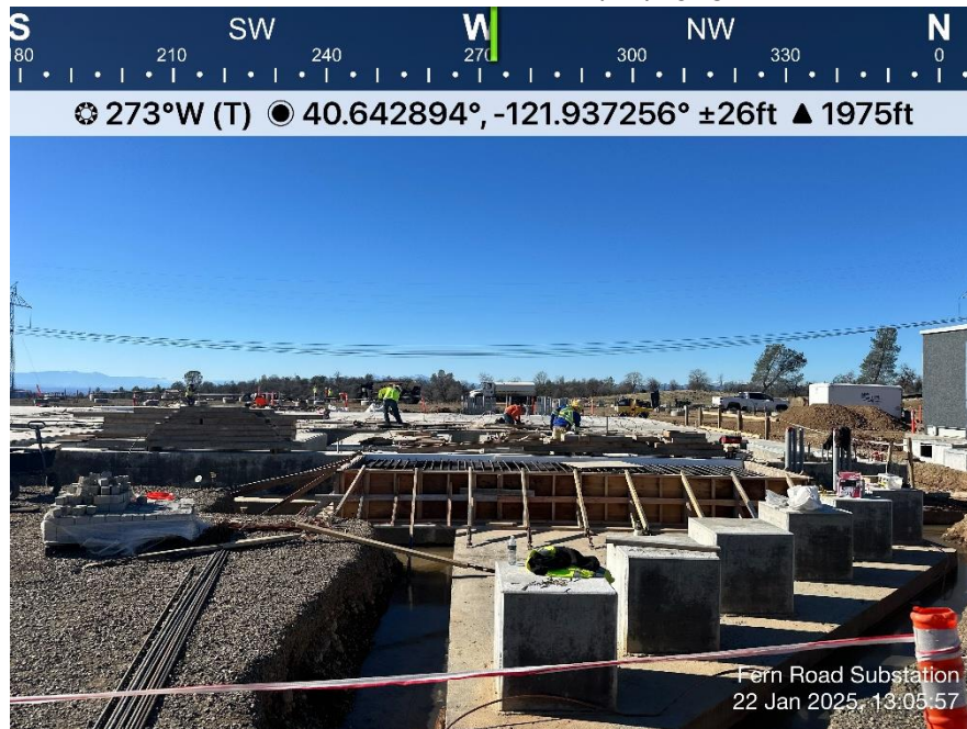
Photo 12. View of TTR trenching and installing ground wire. Direction: North. Date: 1/22/2025
