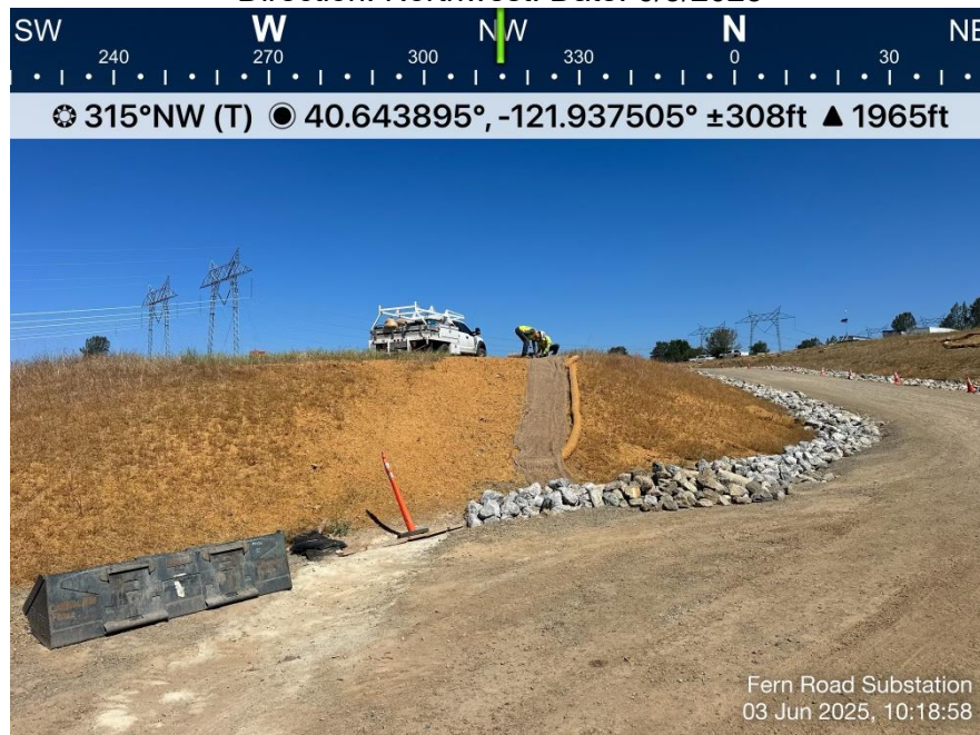
Photo 20. View of crew placing jute netting over exposed soil of backfilled fiber optic trench from MPR-5.
