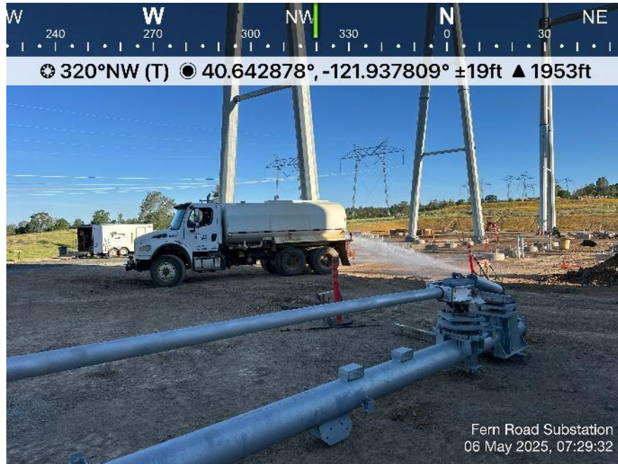
Photo 9. View of TTR crew doing dust control on substation pad. Direction: Northwest. Date: 5/6/2025
