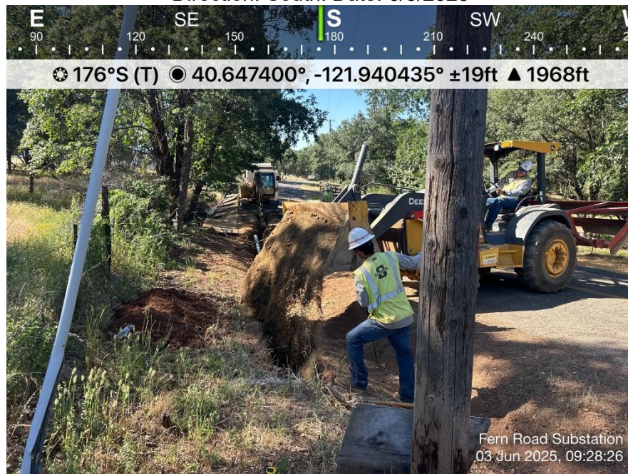
Photo 20. View of crew placing jute netting over exposed soil of backfilled fiber optic trench from MPR-5.
