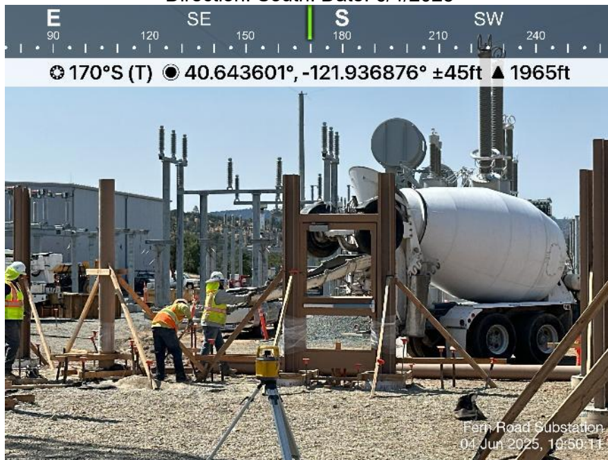
Photo 24. View of crews pouring concrete around PGE wall supports. Direction: South. Date: 6/4/2025
