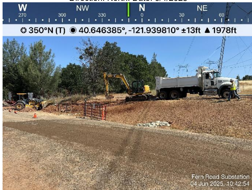
Photo 22. View of Outback crew trenching, laying conduit and backfilling MPR-5 distribution line trench on north side of access road.
