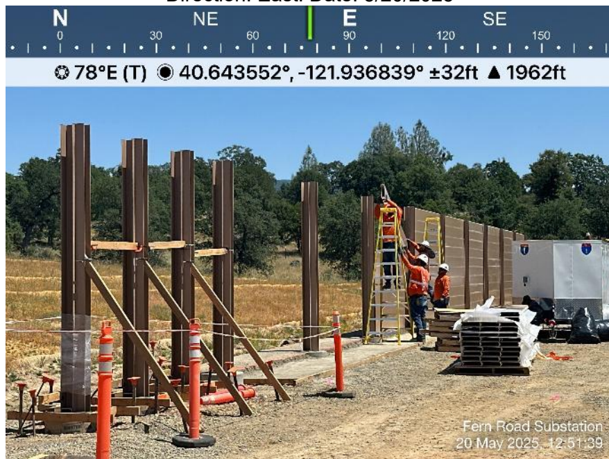
Photo 14. View of Dacon crew constructing wall around PGE portion of substation pad. Direction: East. Date: 5/20/2025
