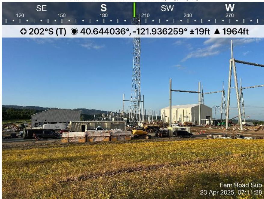
Photo 2. Overview of east half of substation with microwave tower and control enclosures. Direction: South. Date: 4/23/2025
