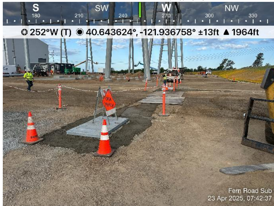
Photo 6. View of Outback crew backfilling trench to pull box on south side of entrance gate for MPR-5 power cables.
