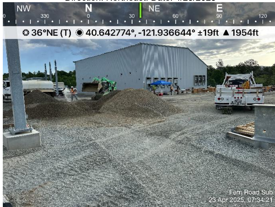
Photo 4. View of TTR crew spreading gravel on substation pad. Direction: Northeast. Date: 4/23/2025
