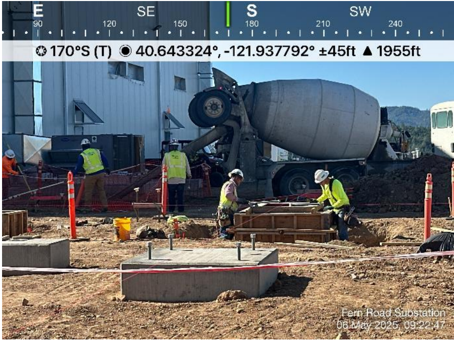
Photo 11. View of TTR crew doing a slurring pour and prepping a foundation form. Direction: South. Date: 5/6/2025
