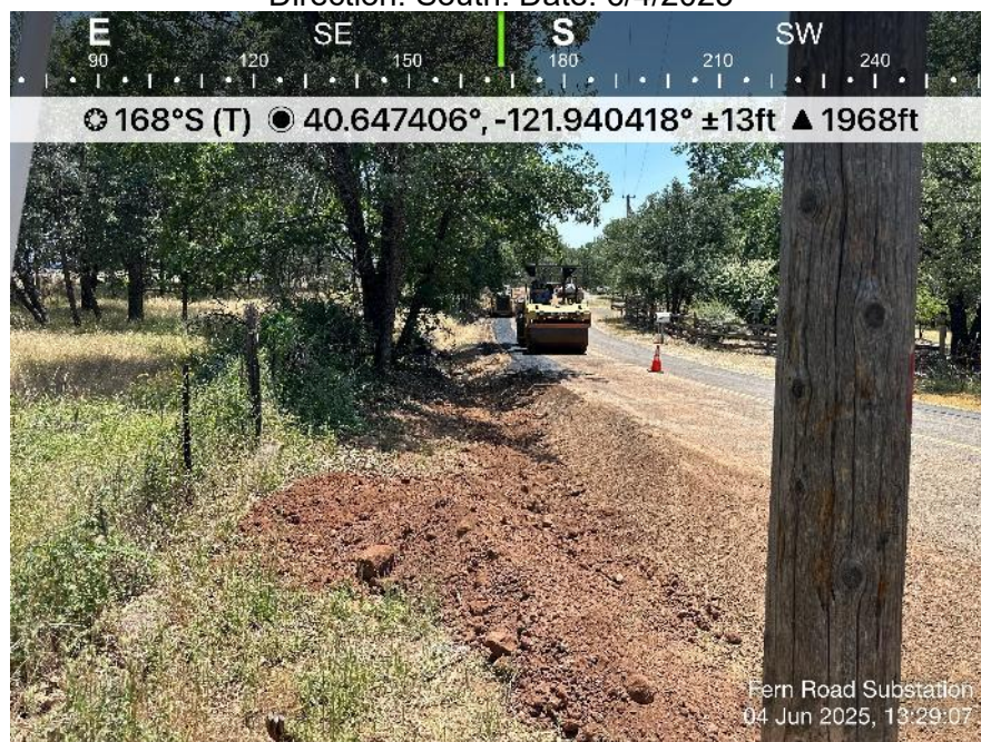
Photo 26. View of MPR-5 backfilled trench and paving activities from distribution pole. Direction: South. Date: 6/4/2025
