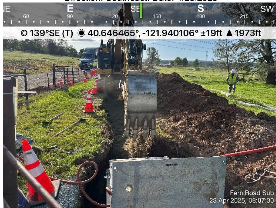
Photo 6. View of Outback crew backfilling trench to pull box on south side of entrance gate for MPR-5 power cables.
