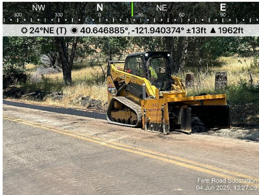
Photo 27. View of Outback skidsteer with trench paver attachment paving trench on Fern Road. Direction: West. Date: 6/4/2025
