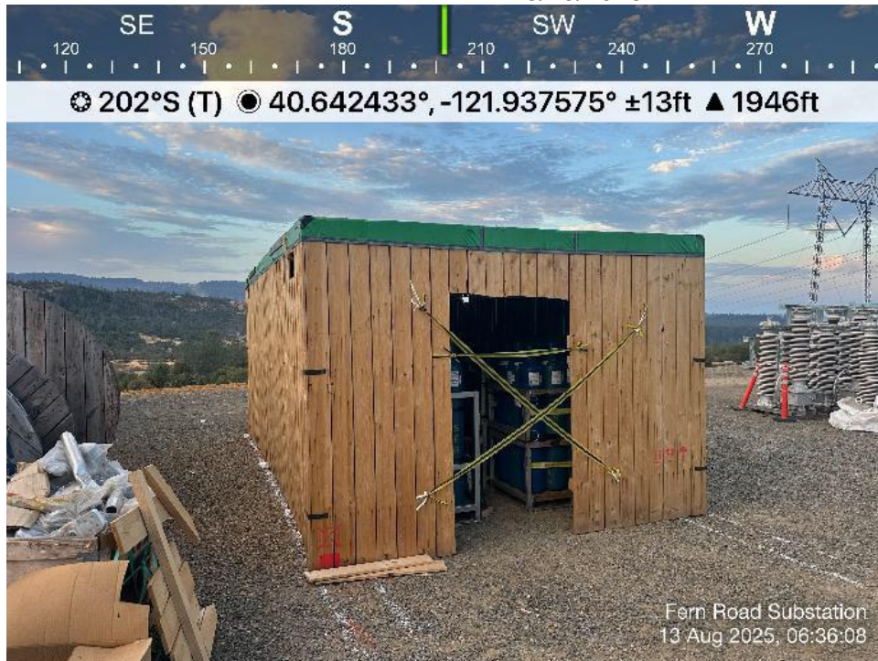
Photo 14. View of SF6 gas cylinder temporary storage on south side of substation pad.
