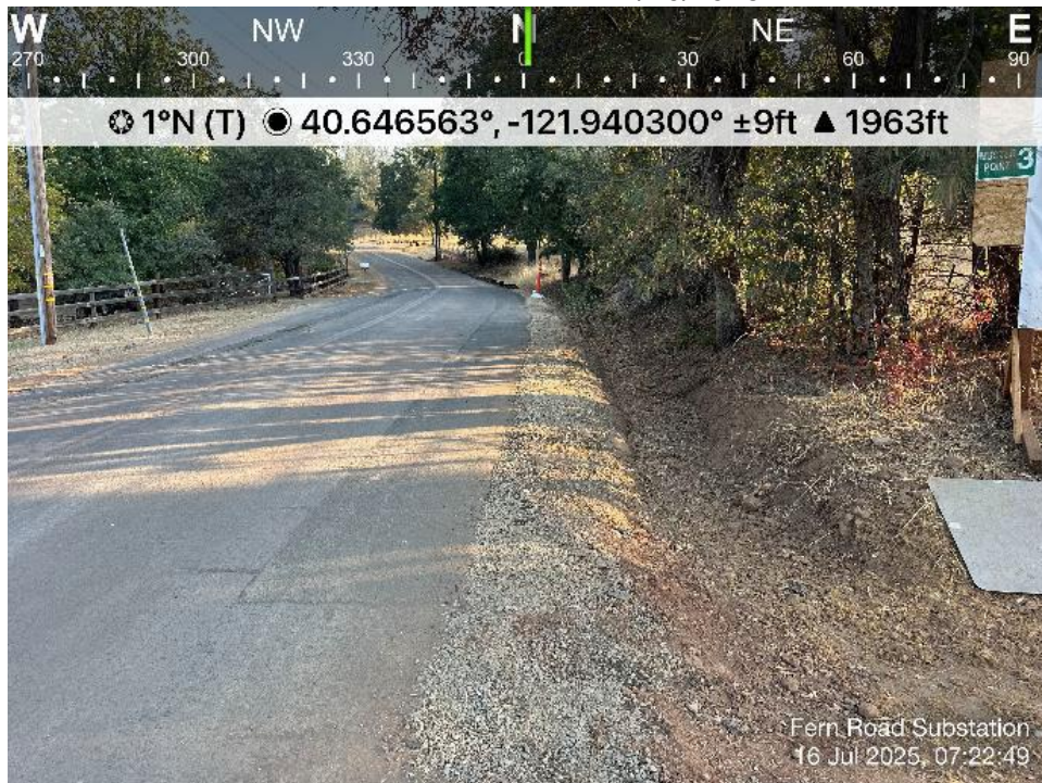
Photo 6. View of completed and repaved MPR-5 electrical trench on Fern Road.
