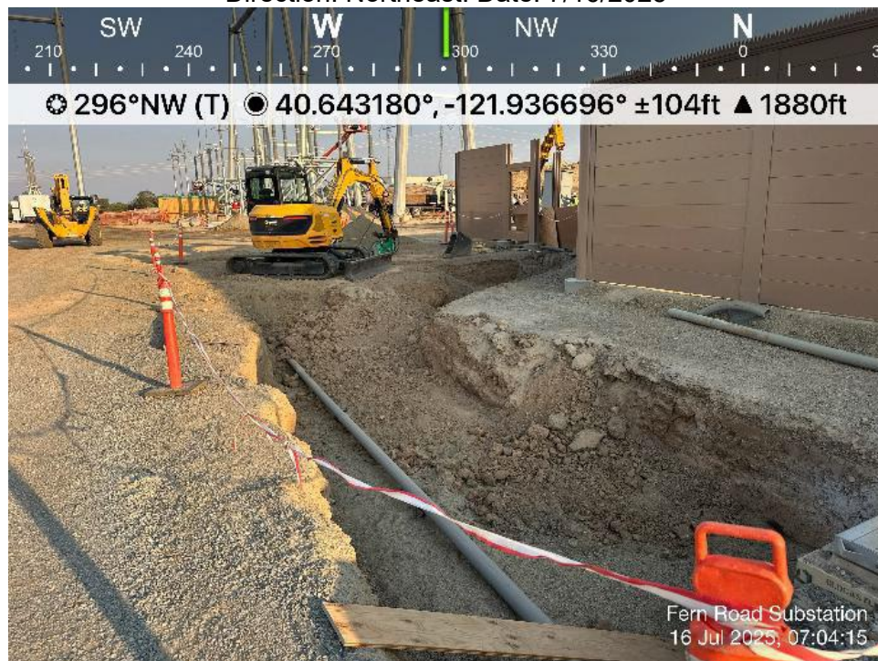
Photo 4. View of excavation and conduit installation outside of PG&E fence area. Direction: Northeast. Date: 7/16/2025
