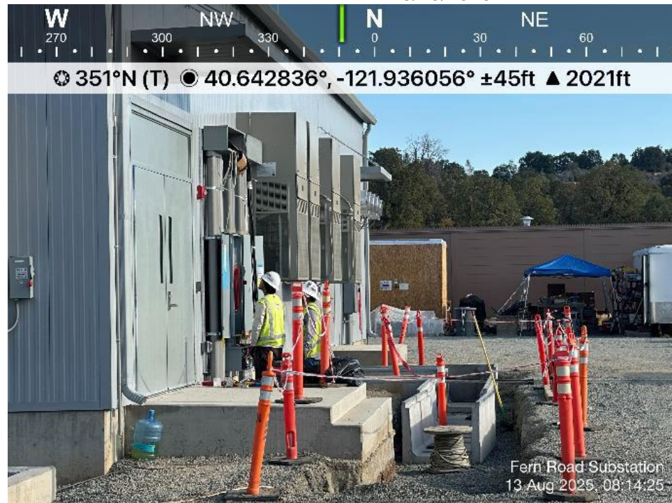
Photo 12. View of control enclosure electrical panel work. Direction: North. Date: 8/13/2025
