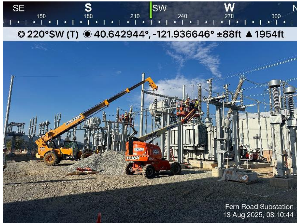
Photo 11. View of overhead electrical infrastructure work. Direction: Southwest. Date: 8/13/2025
