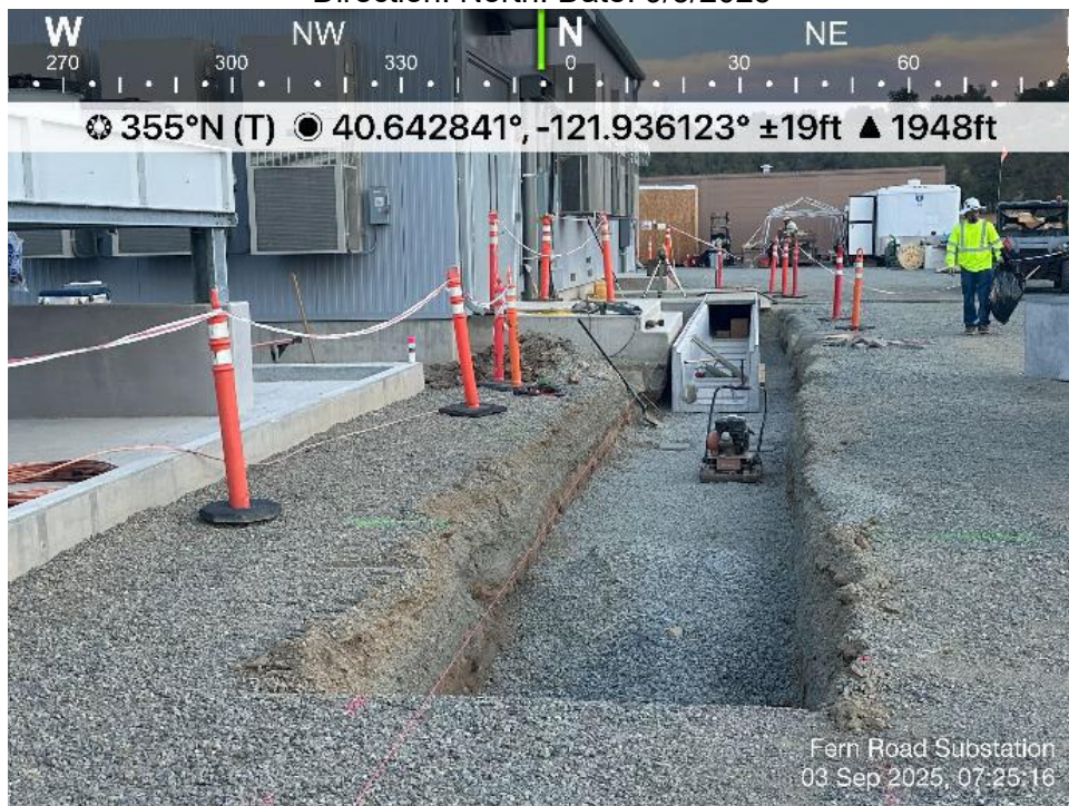
Photo 18. View of progression of cable tray installation outside control enclosure. Direction: North. Date: 9/3/2025
