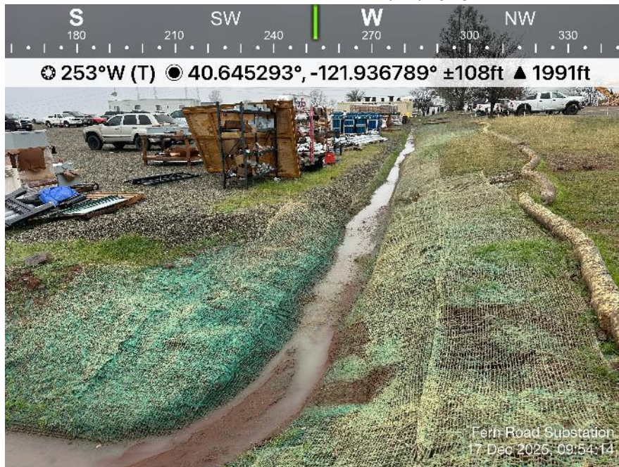
Photo 25. View of laydown/parking area swale. Direction: West. Date: 12/17/2025
