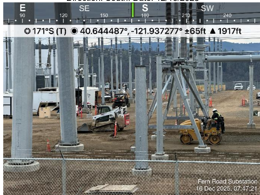
Photo 16. View of TTR civil crew returning substation pad to subgrade.
