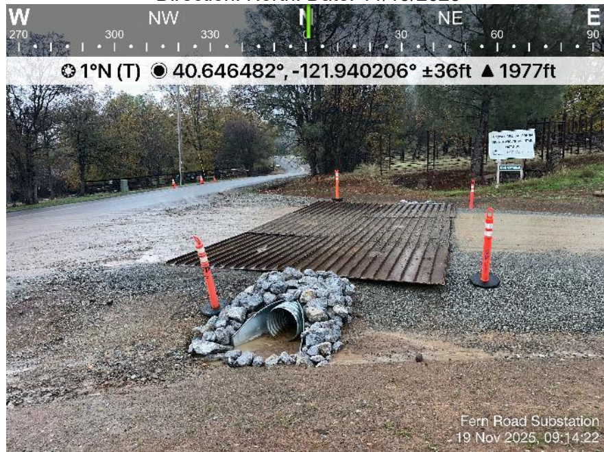
Photo 12. View of recently installed entrance road culvert.
