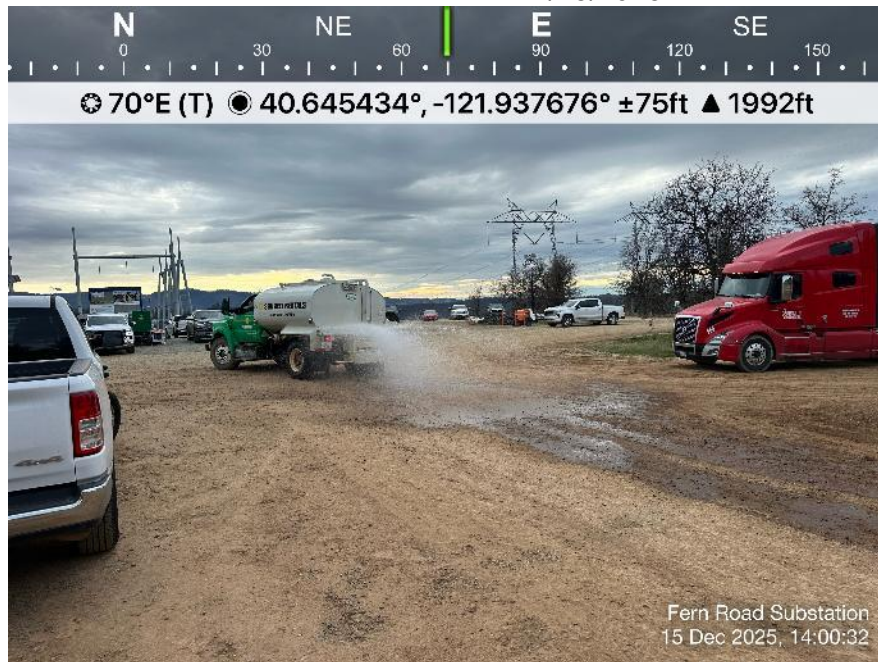
Photo 13. View of dust control in the laydown/parking area. Direction: East. Date: 12/15/2025
