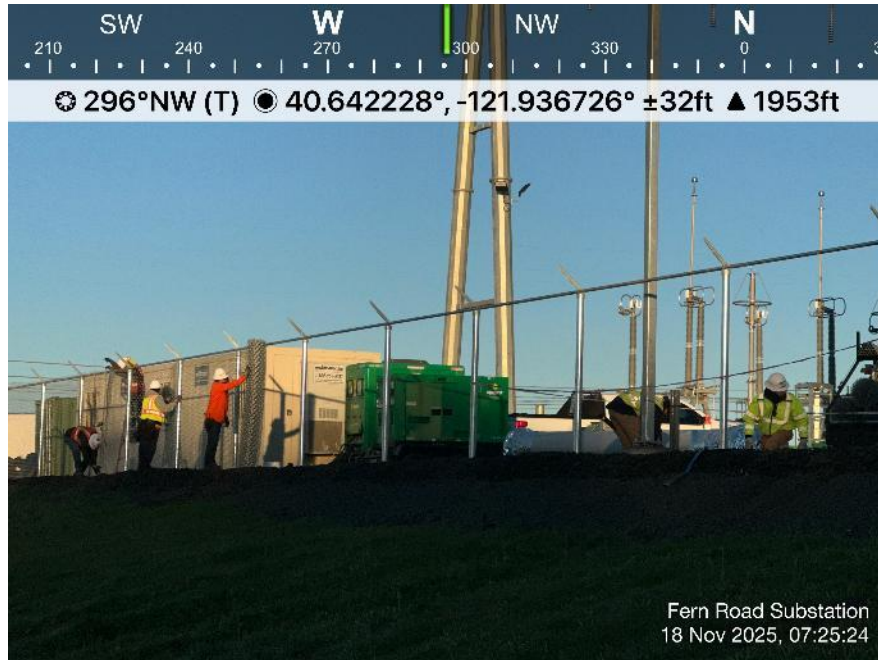
Photo 1. View of Chain Link Fence installing mesh on the perimeter fence. Direction: Northwest. Date: 11/18/2025
