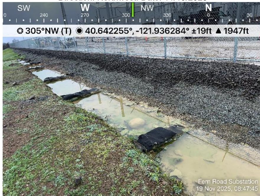
Photo 10. View of gravel bag reinforcement of the area that was beginning to erode from water running down the length of the silt fence. Recommend overlapping the gravel bags so the downslope end of each bag is on top of the upslope end of the next bag.
