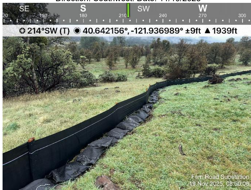
Photo 10. View of gravel bag reinforcement of the area that was beginning to erode from water running down the length of the silt fence. Recommend overlapping the gravel bags so the downslope end of each bag is on top of the upslope end of the next bag.
