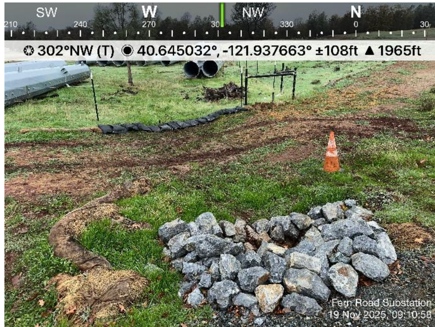
Photo 12. View of recently installed entrance road culvert.
