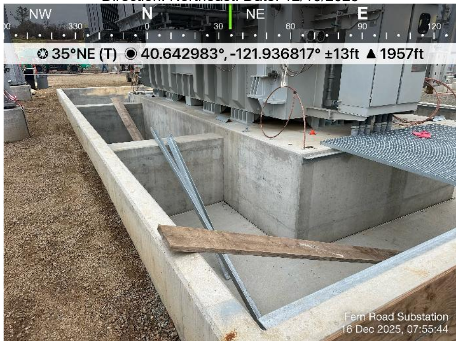
Photo 18. View of transformer containment areas with wildlife escape ramps installed. Direction: Northeast. Date: 12/16/2025
