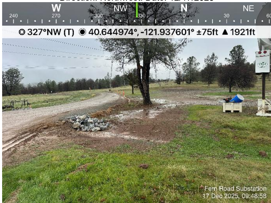
Photo 24. View of area drained by access road culvert. Direction: Northwest. Date: 12/17/2025
