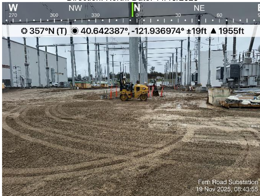
Photo 8. View of mini roller compacting backfilled trench area. Direction: North. Date: 11/19/2025
