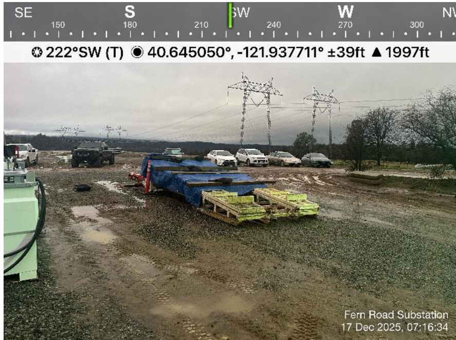
Photo 23. View of concrete washout covered against the rain. Direction: Southwest. Date: 12/17/2025
