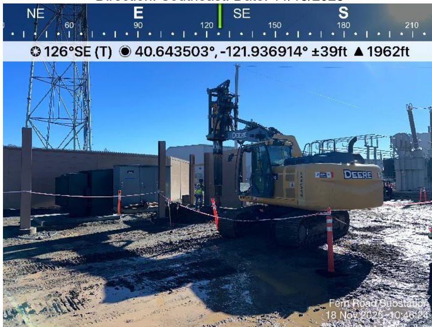
Photo 2. View of drilling in the PG&E fence area. Direction: Southeast. Date: 11/18/2025
