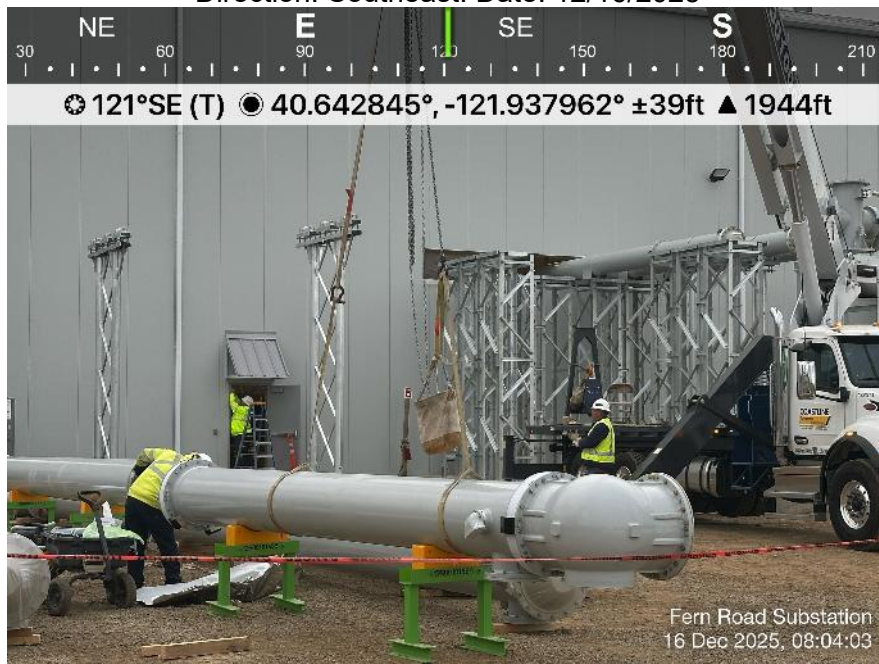
Photo 20. View of TTR preparing to lift a Gas Insulated Bus (GIB) into place. Direction: Southeast. Date: 12/16/2025
