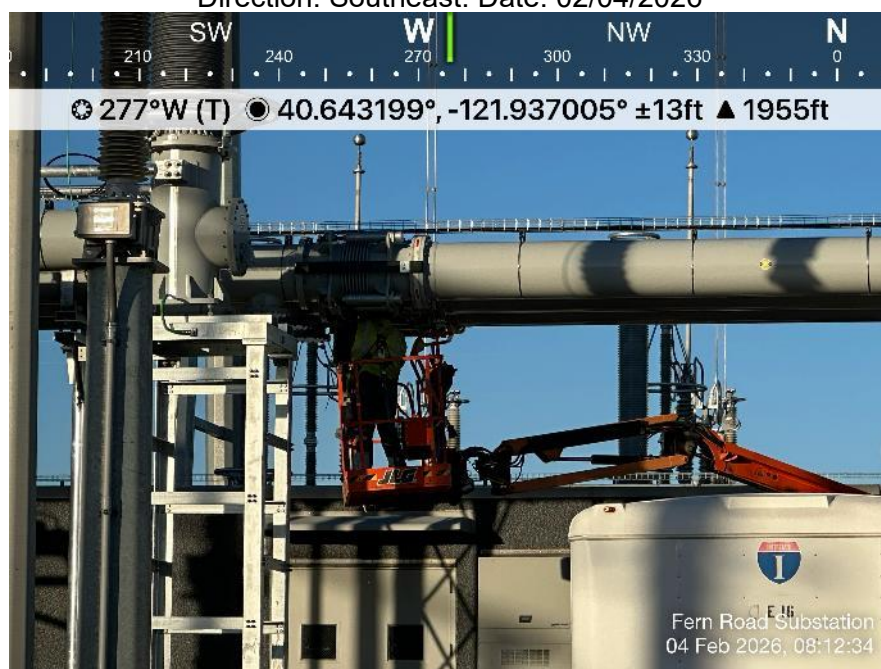
Photo 6. View of TTR doing overhead work on Gas Insulated Bus (GIB). Direction: Southeast. Date: 02/04/2026
