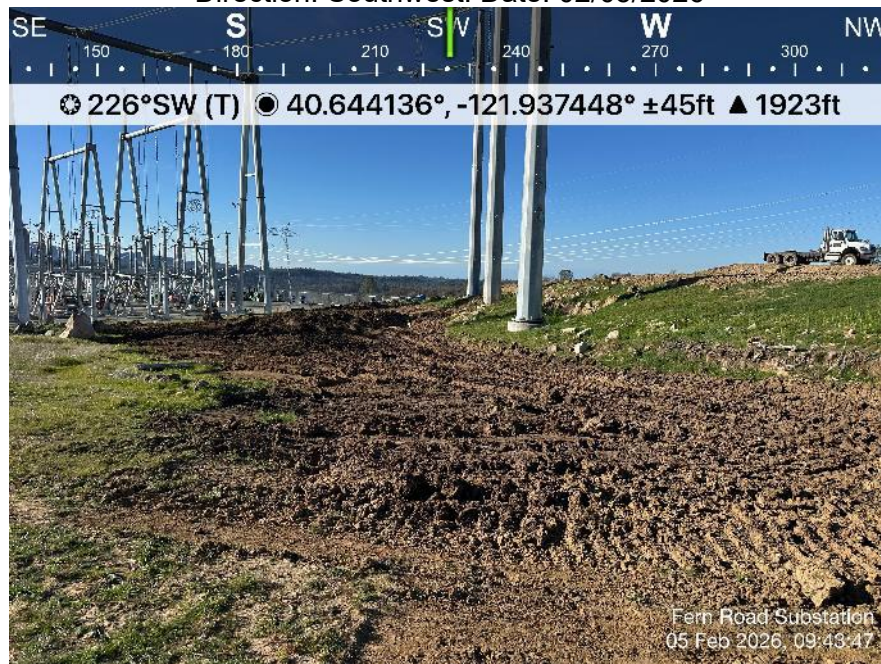
Photo 20. View of area around PG&E tangent poles that needs grading and stabilization. Direction: Southwest. Date: 02/05/2026
