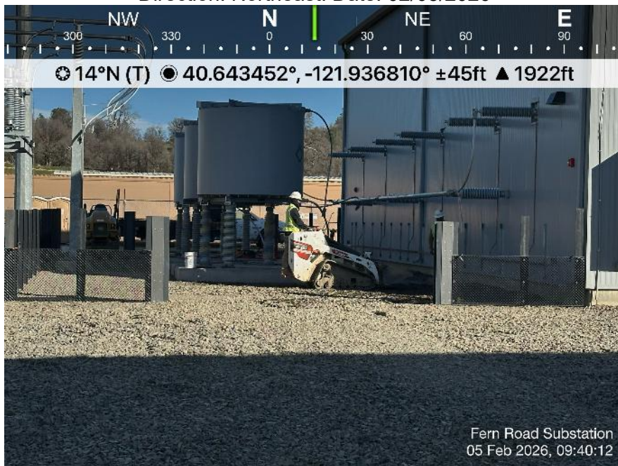
Photo 16. View of TTR spreading finish rock. Direction: Northeast. Date: 02/05/2026
