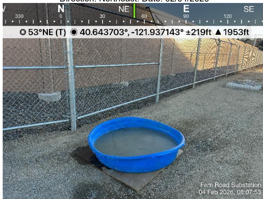
Photo 10. View of concrete washout used after pour for non-conductive fence post footings. Direction: Northeast. Date: 02/04/2026
