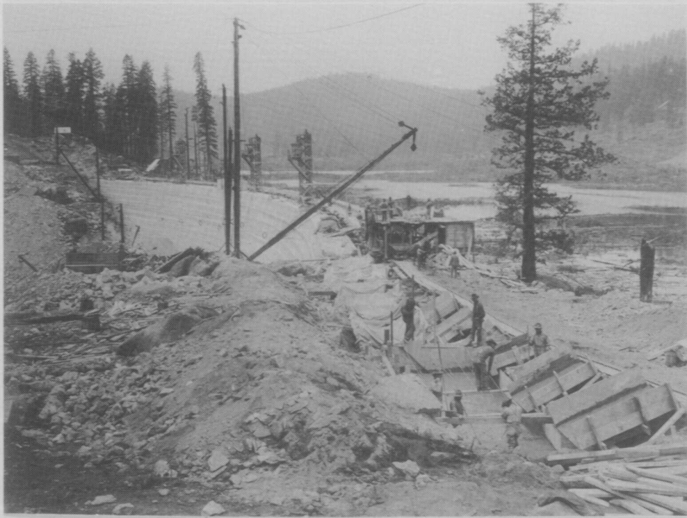
Plate 8 Pouring concrete at Dam No. 1, 1913 (SCE var. [b]:Album 3, No. 430).
