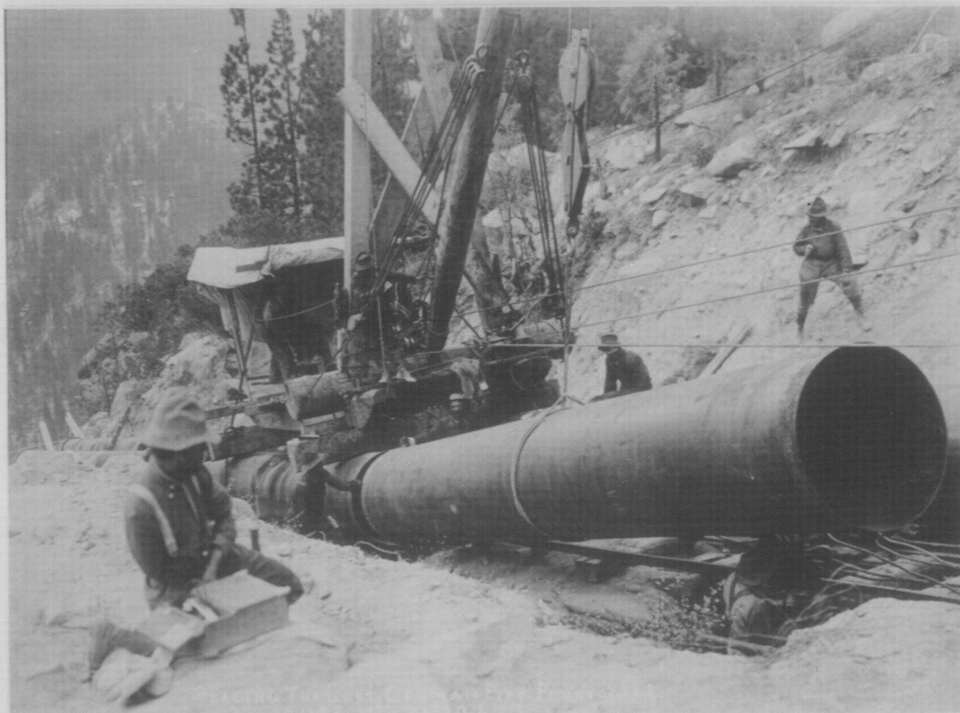
Plate 17 Penstock Construction, Penstock No. 1, 1913 (SCE var. [b]:Album 5, No. 631).
