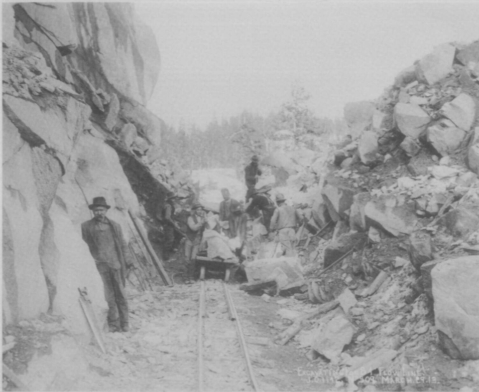
Plate 12 Excavating for the 84-inch flowline pipe, 1913 (SCE var. [b]:Album 5, No. 309).
