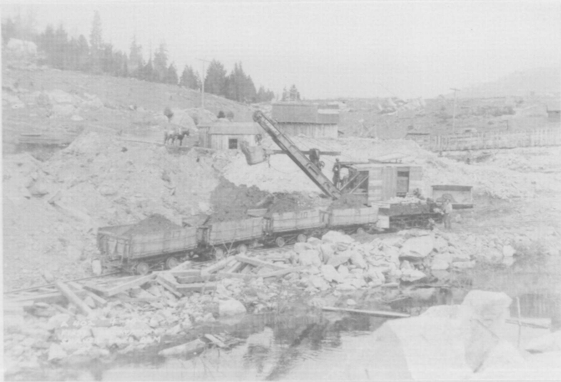
Plate 49 Initial Excavation for the Shaver Lake Dam, April 1926 (SCE var. [a]:Unnumbered Album, No. A402).
