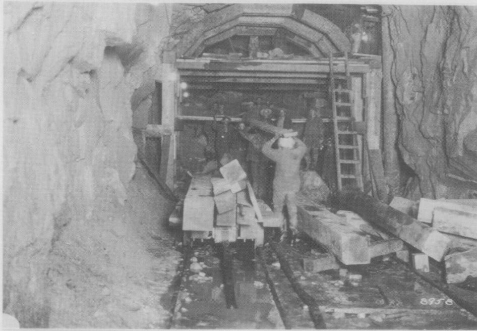
Plate 41 Timbering operations in the Florence Lake Tunnel, 1923 (SCE var. [b]:Album 1, No. 13-8958).
