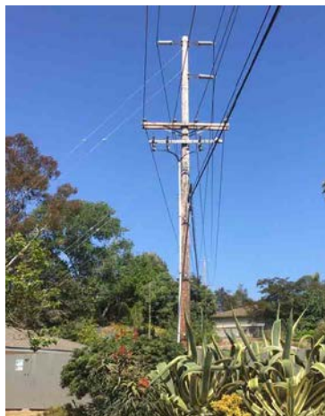
Pole Loc. 28: installed 1982, wood, looking east
