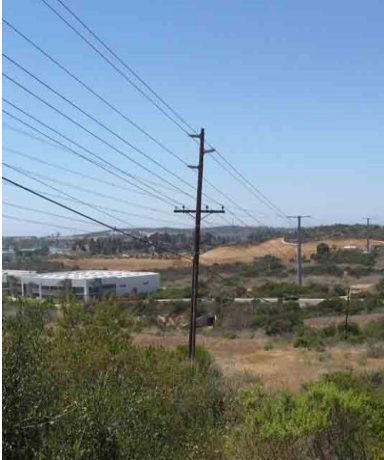
Pole Loc. 54.1: installed 1964, wood, looking northwest
