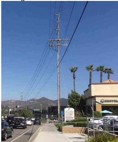
Pole Loc. 21: 1991, wood, looking southeast
