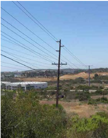
Pole Loc. 54.1: installed 1964, wood, looking northwest
