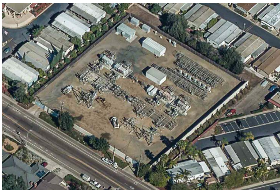
Figure 4. Bird's Eye Aerial View of San Marcos Substation
