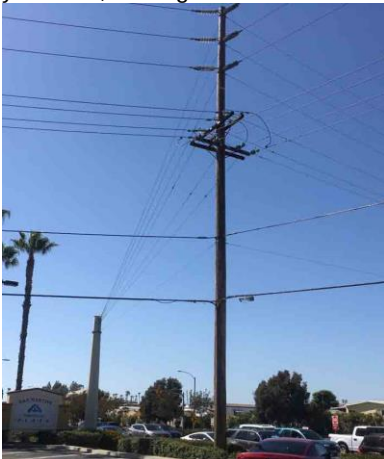
Pole Loc. 22: 1991, wood; Pole Loc. 24: recent steel stub, looking west
