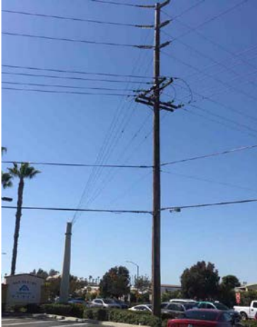
Pole Loc. 22: installed 1991, wood; Pole Loc. 24: recent steel stub, looking west
