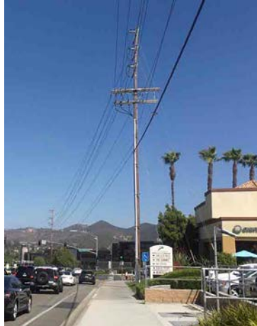
Pole Loc. 21: installed 1991, wood, looking southeast
