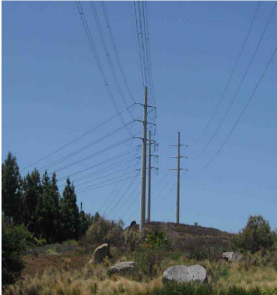
Steel poles looking south-southeast from Auto Park Way
