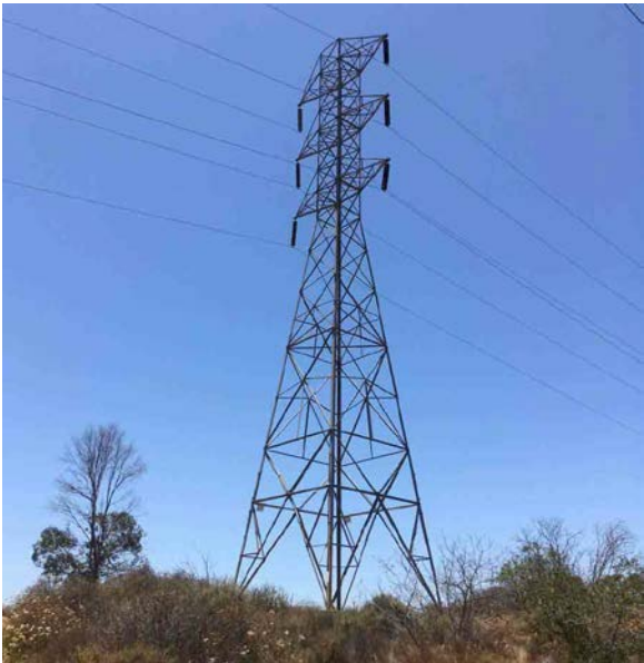
Tower Loc. 86: looking southwest from near intersection of Questhaven Road and Old Glen Street in San Marcos
