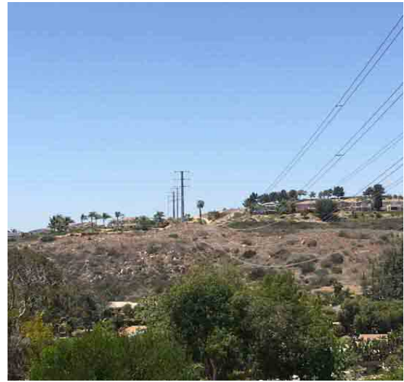
TL 13811/13825 looking north from Via Allondra
