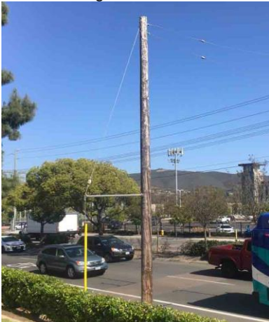
Pole Loc. 17: wood stub under 50 years old, looking southeast
