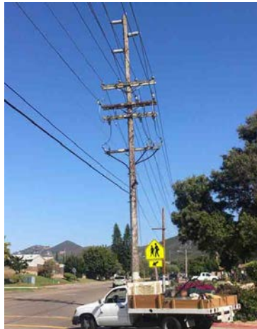
Pole Loc. 6, installed 1967, wood, looking southeast
