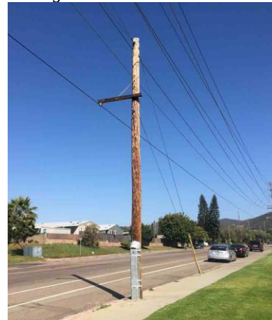
Pole Loc. 5: wood stub under 50 years old, looking east
