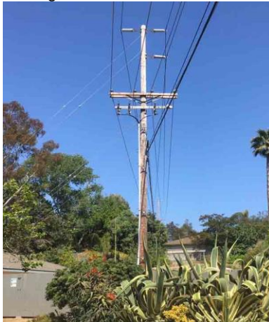
Pole Loc. 28: installed 1982, wood, looking east
