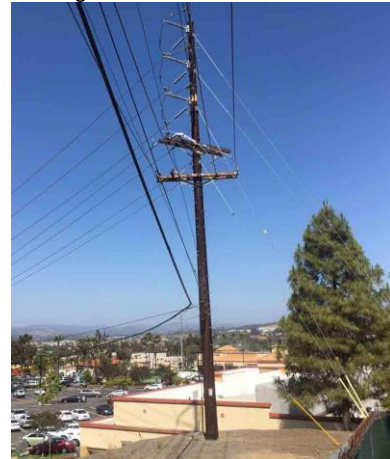
Pole Loc. 25: recent steel pole, looking east
