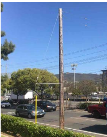
Pole Loc. 17: wood stub under 50 years old, looking southeast
