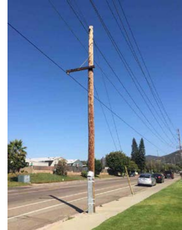
Pole Loc. 5: wood stub under 50 years old, looking east
