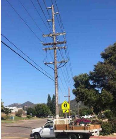
Pole Loc. 6: installed 1967, wood, looking southeast
