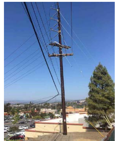
Pole Loc. 25: recent steel pole, looking east
