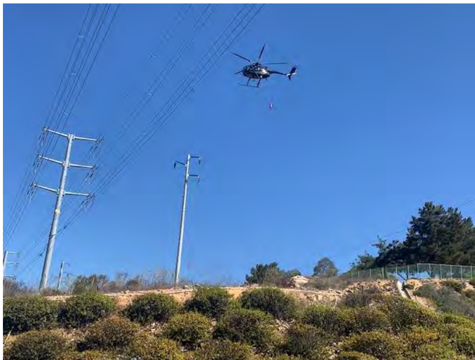
Photograph 48: August 30, 2022. View of helicopter flying hard line near Location 58. Facing: Northeast.
