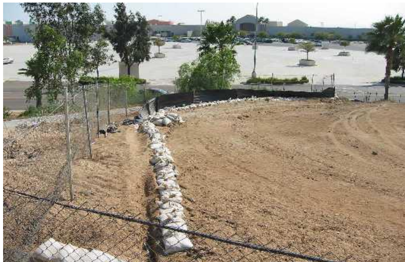
Gravel bags used as perimeter control.
