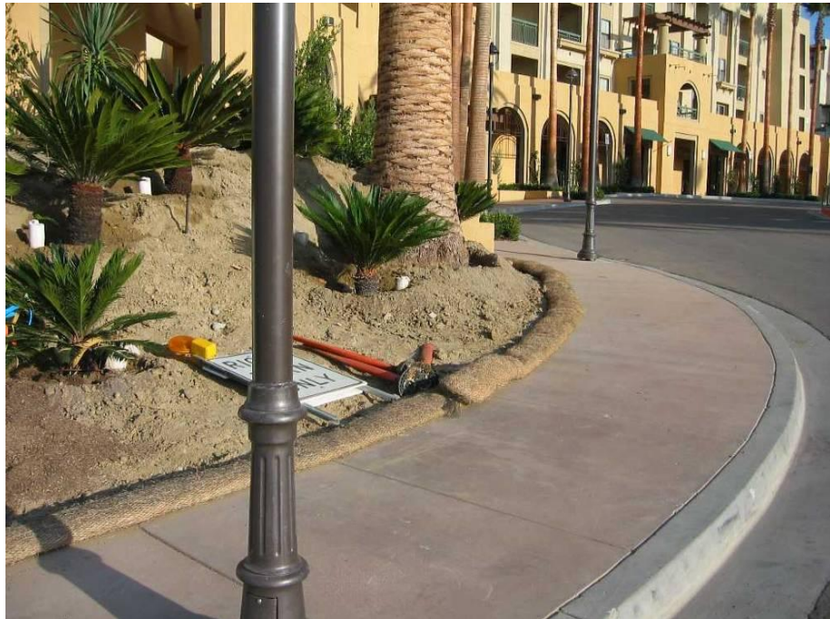
Fiber rolls as perimeter control.
