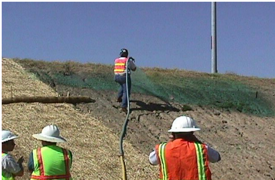
Applying soil stabilization manually in harder to reach areas.
