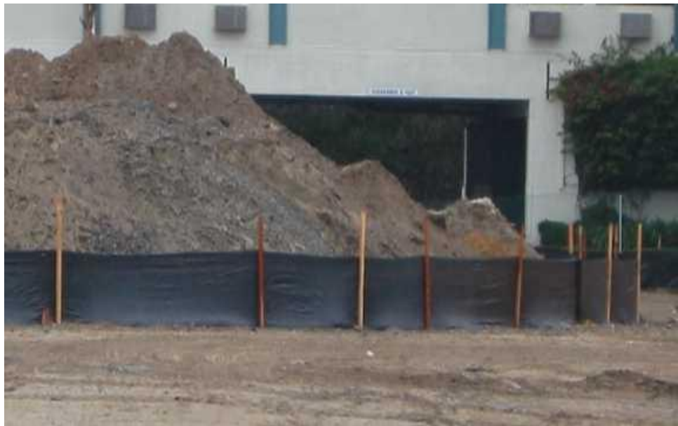
Silt fence used for stockpile perimeter control.
