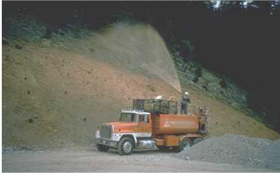
Applying hydraulic mulch.
