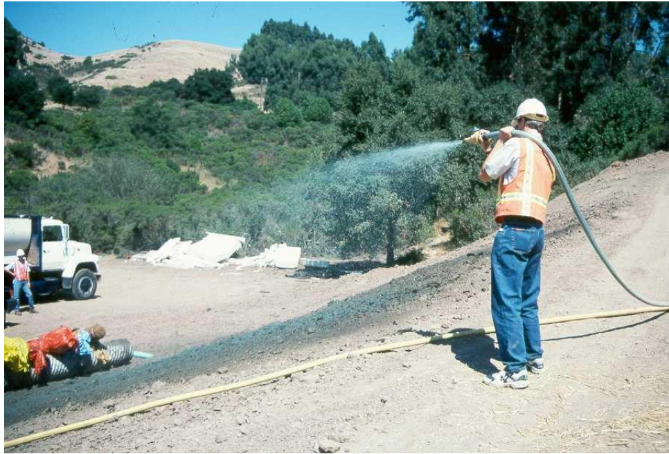
Applying hydroseed.
