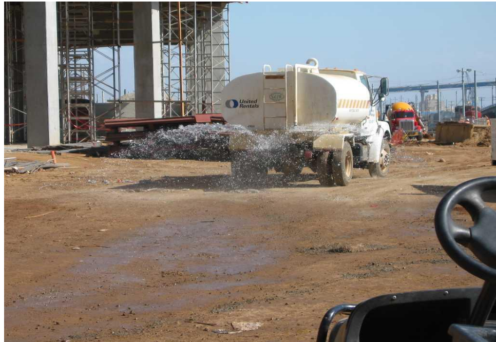
Water being applied for dust control.
