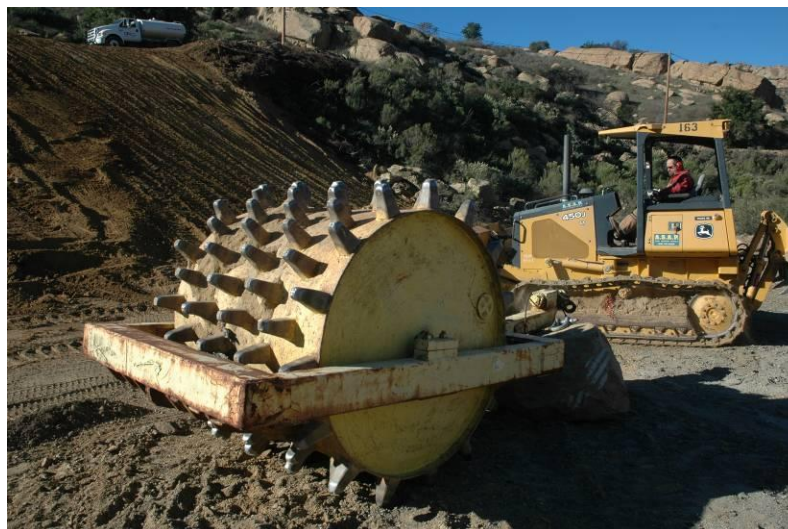
Sheepsfoot used for soil preparation
