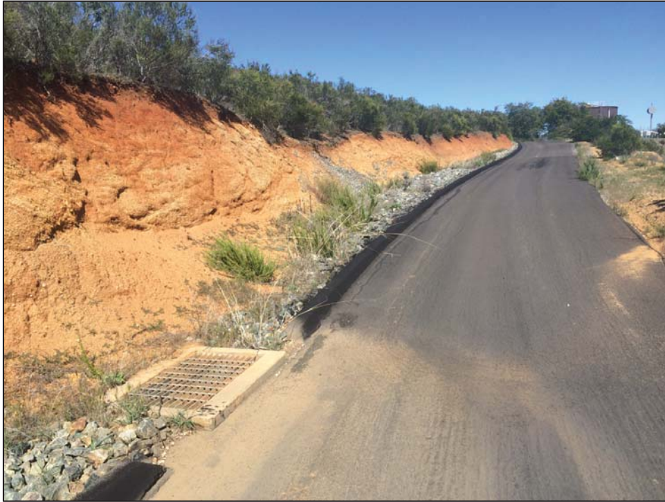
Figure 25. Western Segment of Bell Bluff Truck Trail, View to the Northeast
