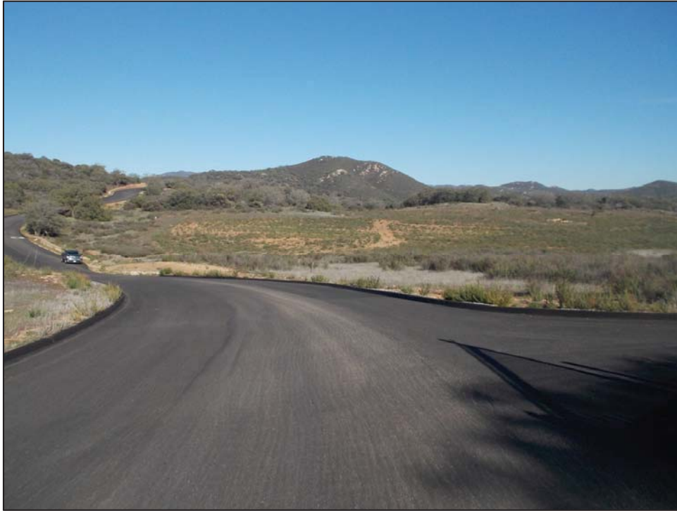
Figure 6. Overview of SVC Location, View to the East
