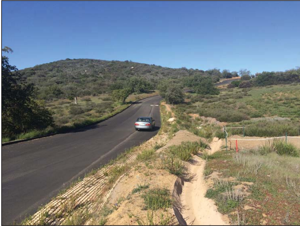
Figure 27. Middle Segment of Bell Bluff Truck Trail, View to the Northeast
