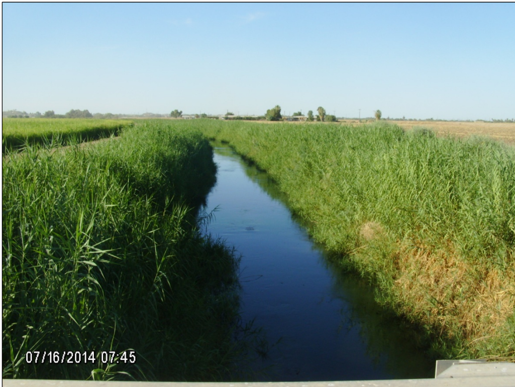
Photo E.4. Reservation Main Drain at Arnold Road, view to south.
