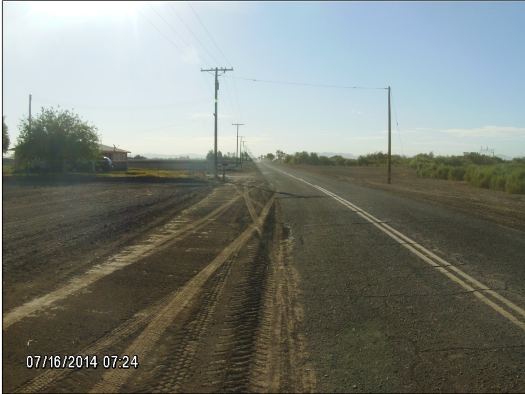
Photo E.3. West end of project corridor on Arnold, view to east.
