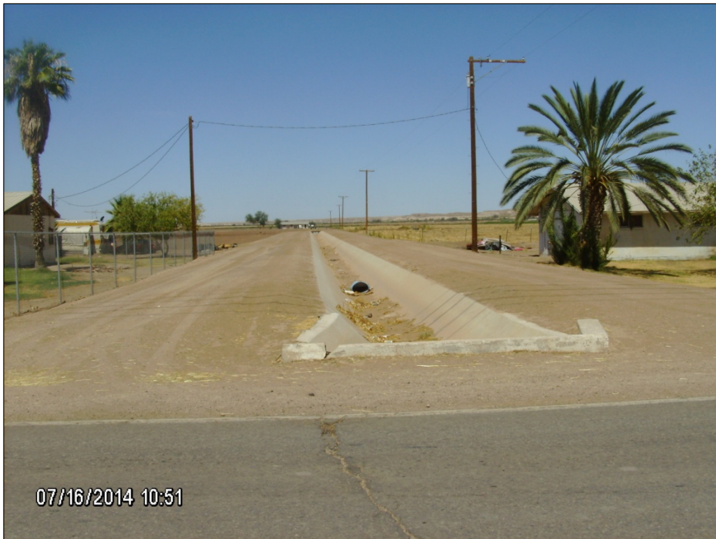
Photo E.12. Pima Canal at Picacho Road, view to east.
