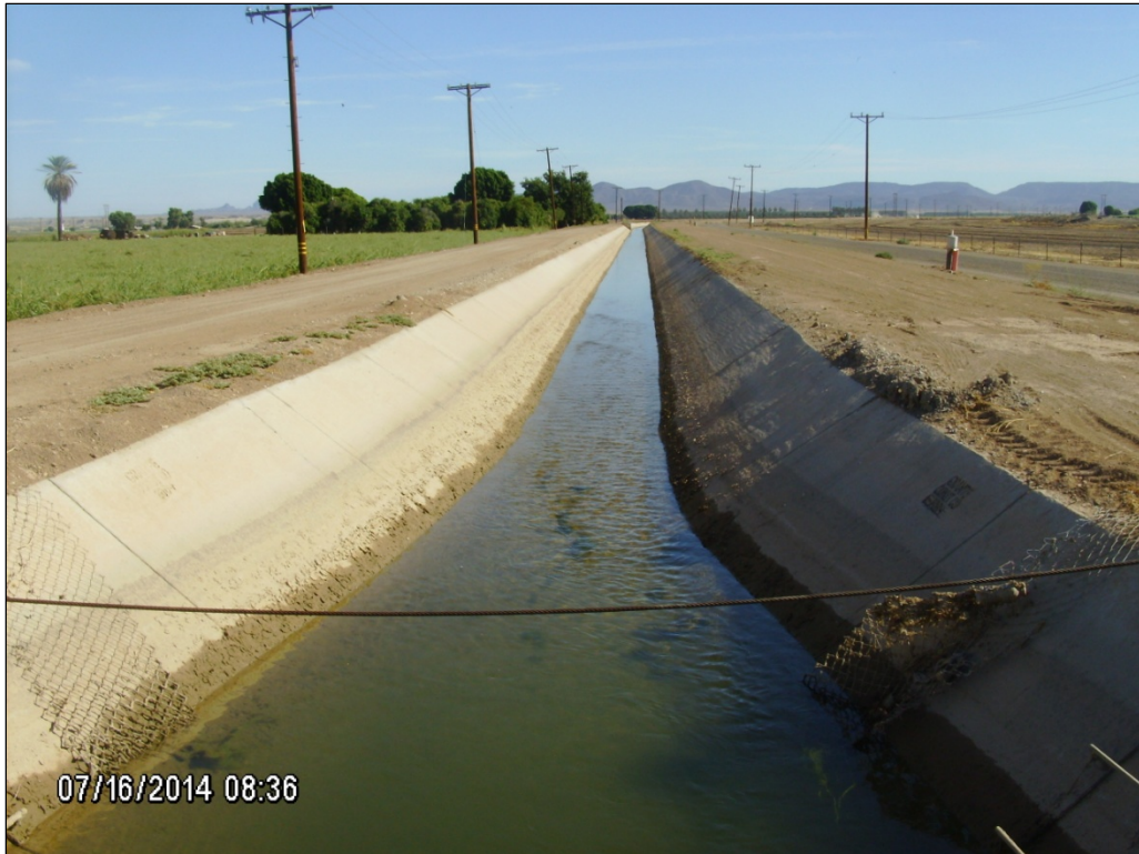
Photo E.6 Cocopah Canal at Arnold Road, view to north.
