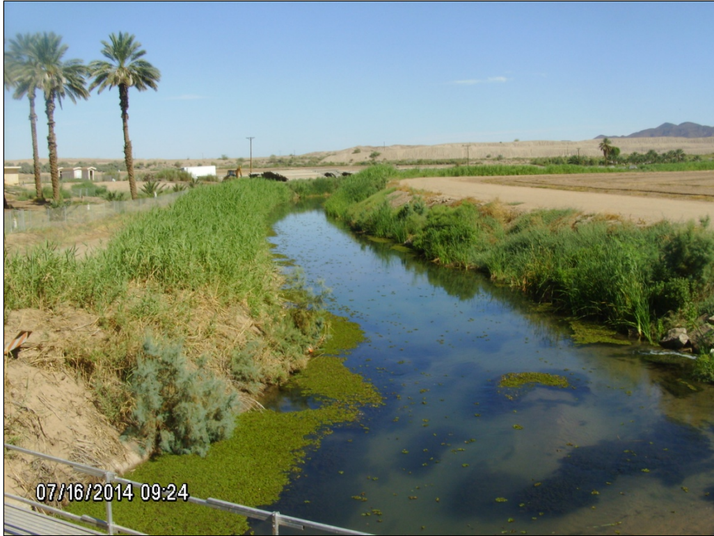
Photo E.9. Reservation Main Drain at Stalnacker Road, view to north. Note Kariba Weed in canal.
