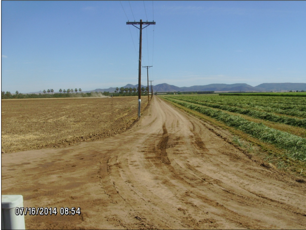
Photo E.7. Haughtelin and Perez Roads, view to north.
