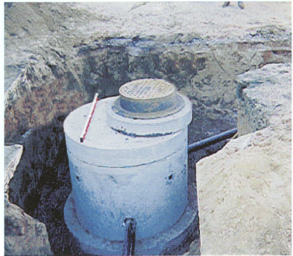
Manhole Installation
