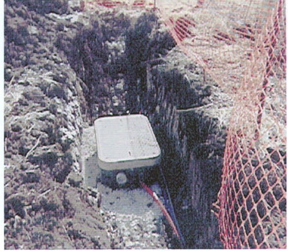
Handhole Installation
