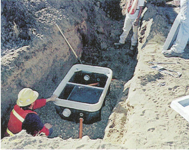
Handhole Installation
