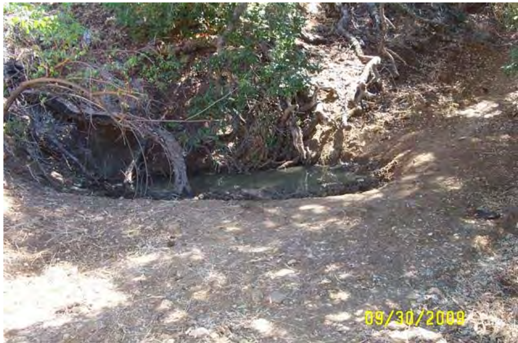
S9: Tributary to Santa Margarita Creek (NRPW), crossing along access road to Tower 69/0, culvert inlet
