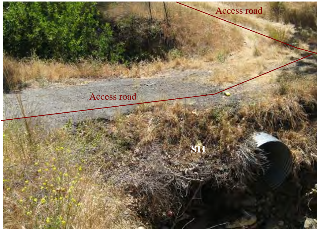
S11: Tributary to San Luis Obispo Creek (NRPW) with two culverts (3 and 4 foot wide), facing southeast June, 2009
