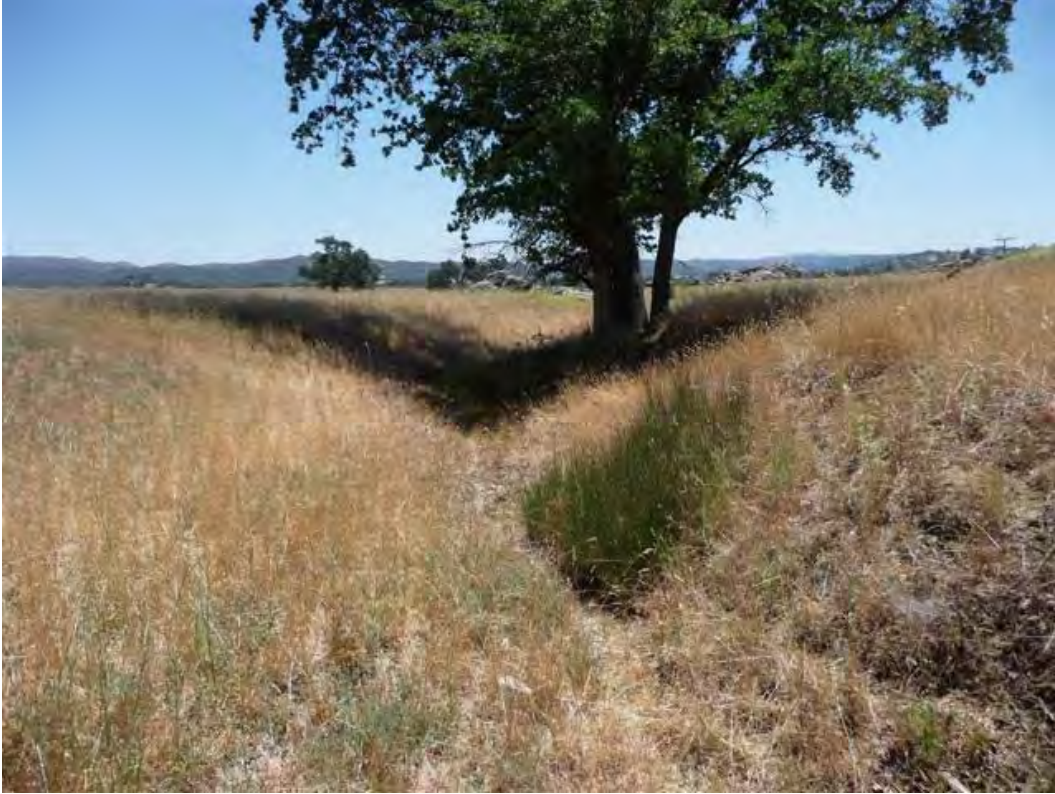
S40 (Tributary to Santa Margarita Creek): NRPW approximately 100 feet north of Pole 65/2, facing southeast June, 2009
