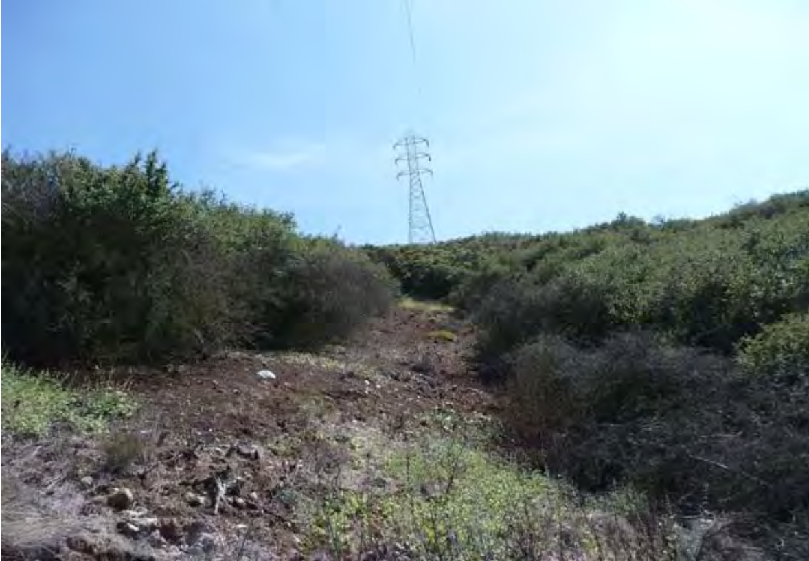
Tower 74/2 in northern mixed chaparral, facing north
