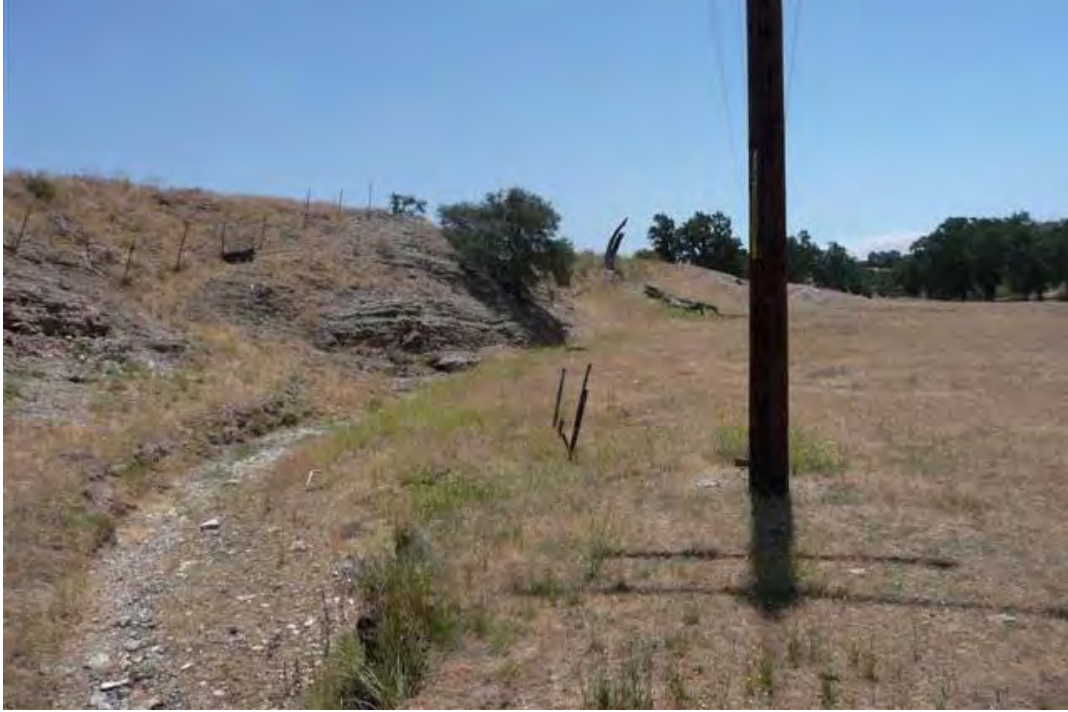
S30 (South Fork Paloma Creek): NRPW east of Pole 63/8, facing south
