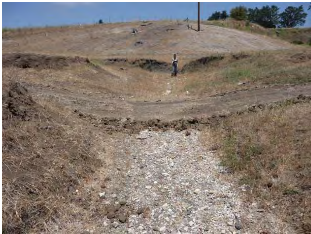
S2c: NRPW SW of Pole 63/9, facing northeast
