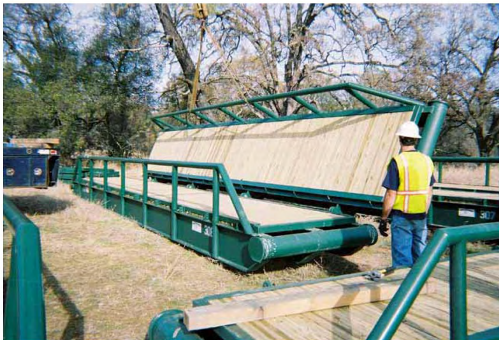
Figure 2.5-1: Typical Temporary Bridge
