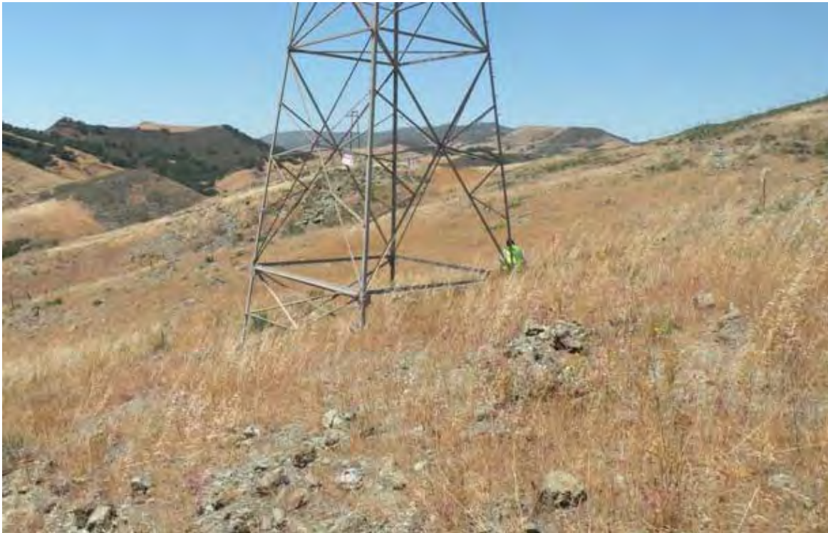
Tower 73/1 on serpentine outcrops, facing north
