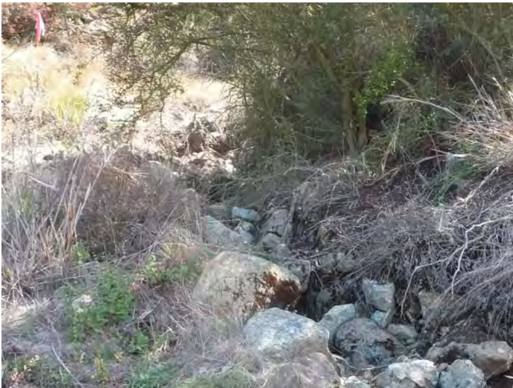
S31: NRPW west Tower 74/1, facing upstream June, 2009
