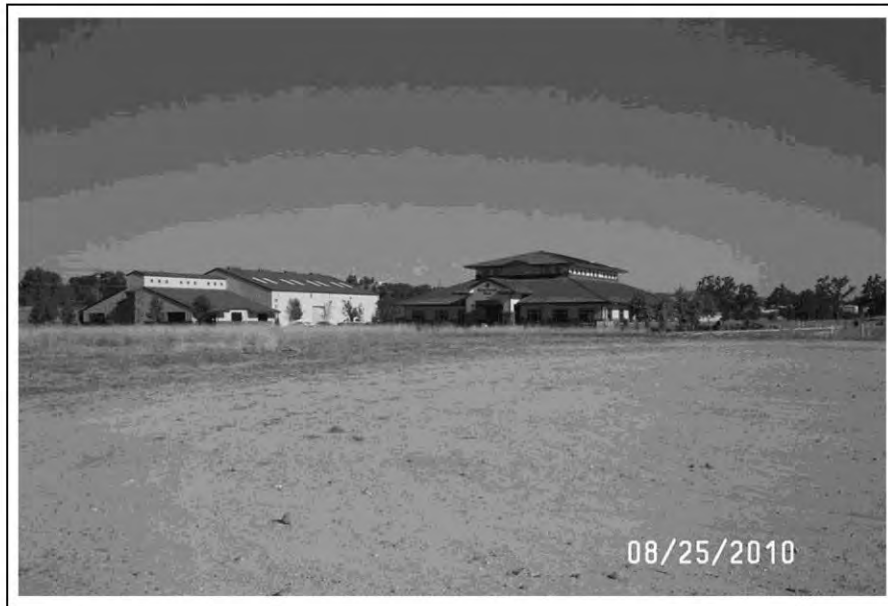
Templeton Service Center Staging Area Looking North-Northwest.
