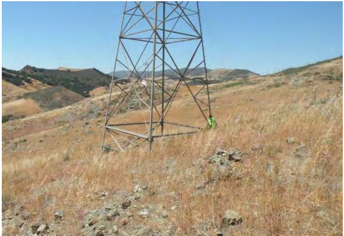
Tower 73/1 on serpentine outcrops, facing north
