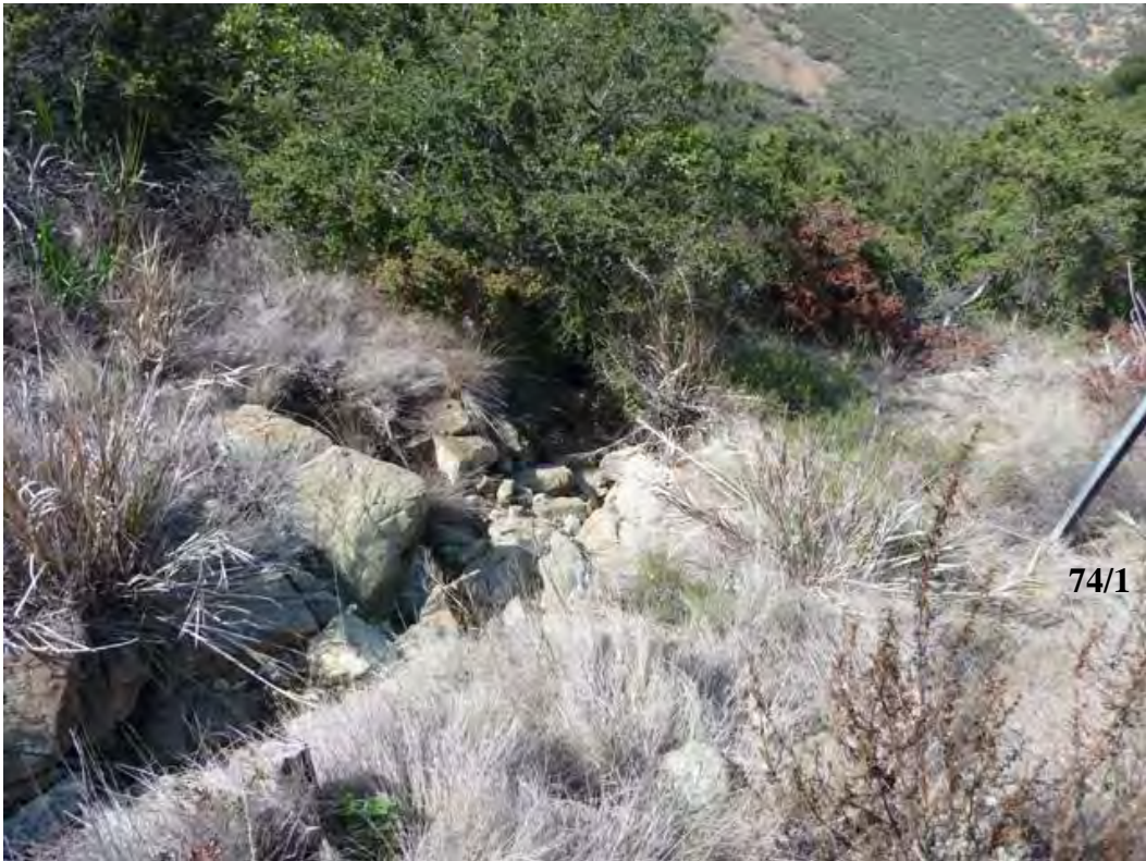
S31: NRPW west Tower 74/1, facing downstream
