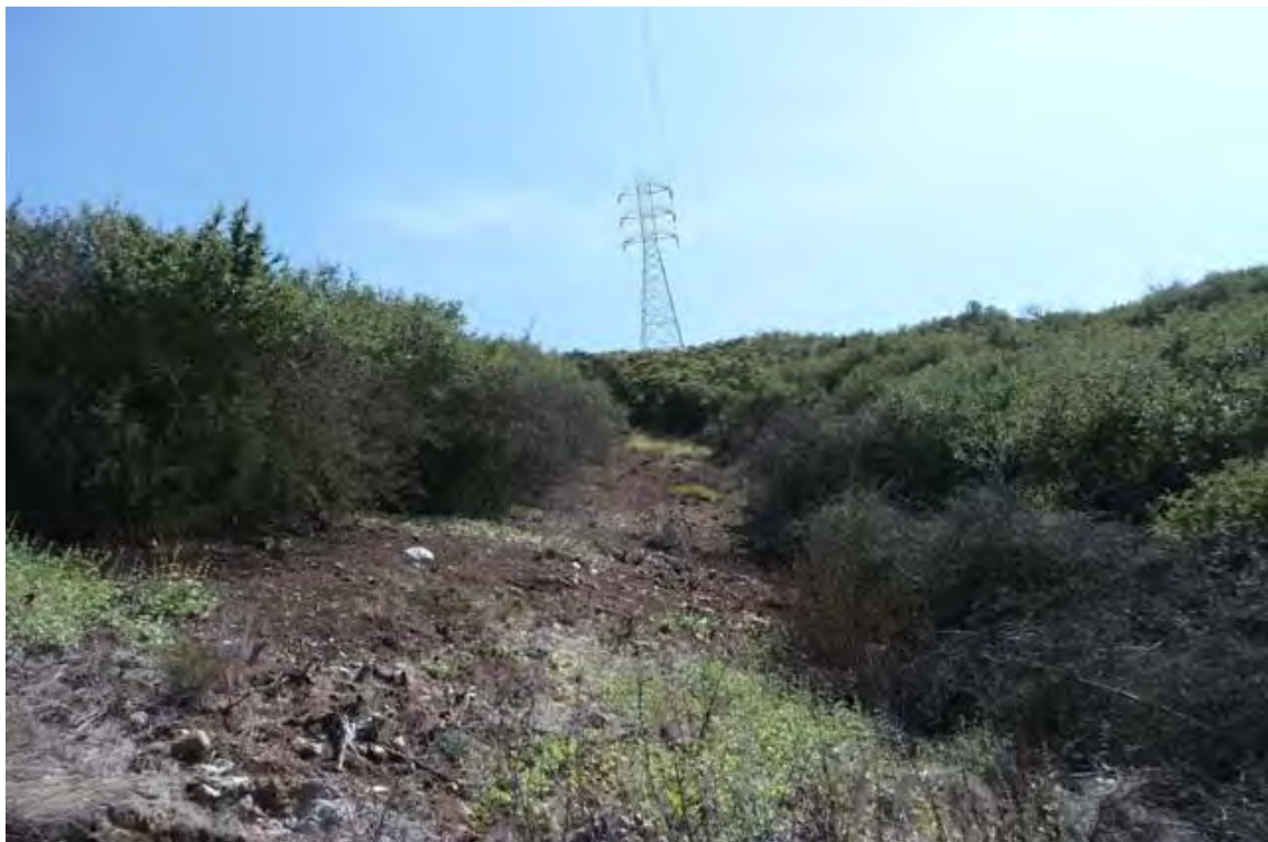
Tower 74/2 in northern mixed chaparral, facing north
